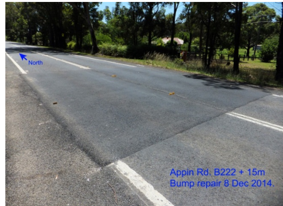
Photo 2: Pavement repair at B222 + 15m, 8/12/2014 (Photo courtesy of Colin Dove).
