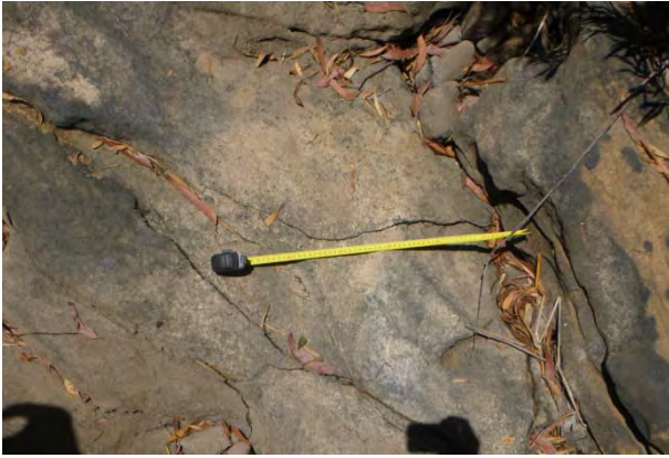
Photo 3: Impact WCA5_LW38_008- Fracturing identified on the Georges River. Taken on 10/12/2015.
