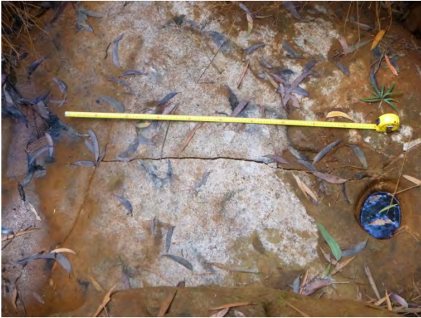
Photo 5: Impact WCA5_LW38_007- additional fracturing to base of GR110. Taken on 16/11/2015.
