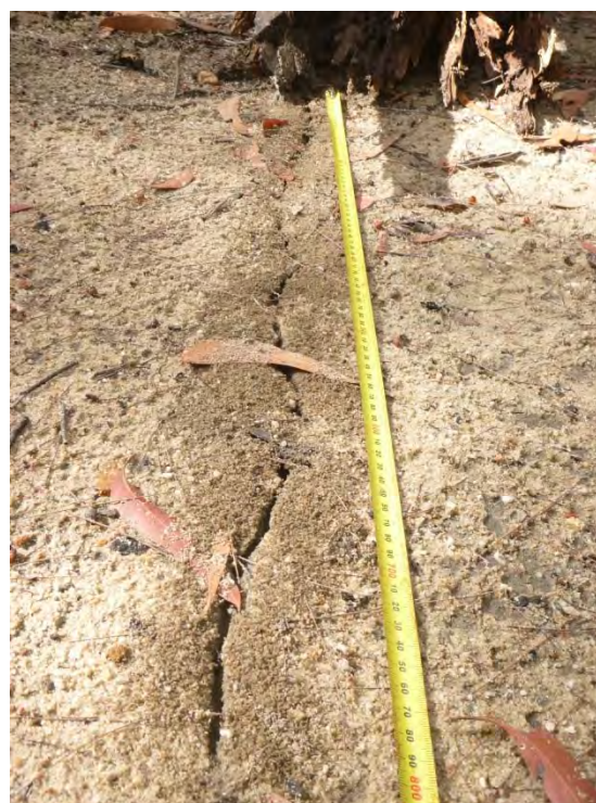
Photo 2: WCA5_LW38_011 – Width of widest soil crack identified. Taken on 16/3/16.
