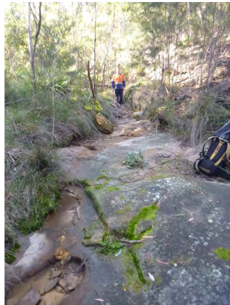
Photo 5: WCA5_LW38_003 – Length of fracturing within Channel 2. Taken on 03/08/2015.
