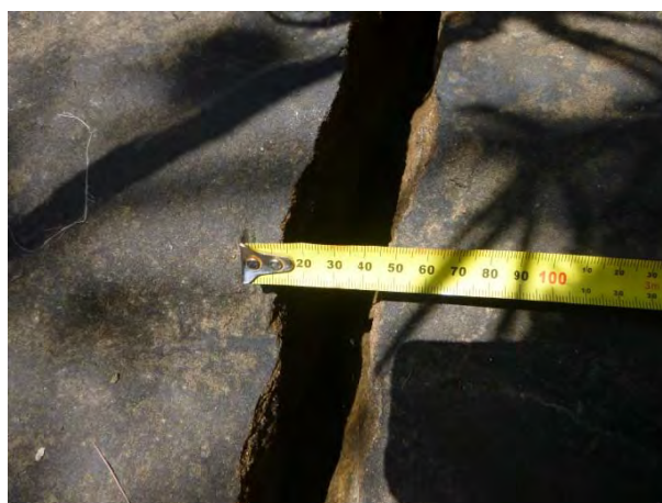
Photo 2: Impact WCA5_LW38_008- Fracturing identified on the Georges River. Taken on 10/12/2015.
