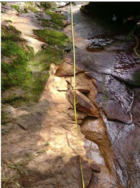
Photo 31: WCA5_LW36_001- fracturing and uplift looking upstream. Taken on 24/04/2015
