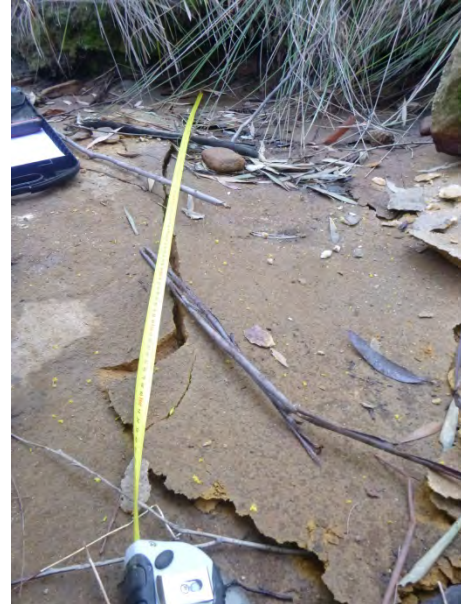
Photo 7: WCA5_LW38_003 – Longest section of uplift within fracture zone. Taken on 03/08/2015.
