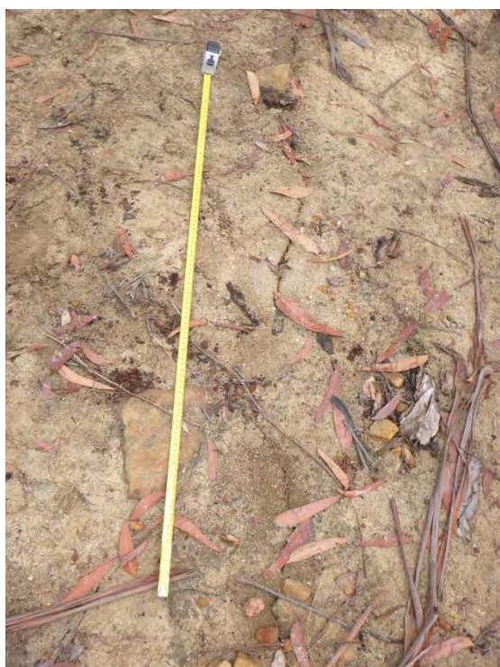
Photo 1: WCA5_LW38_011 – Soil cracking on access track. Taken on 16/3/16.
