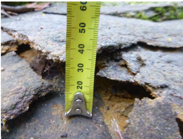
Photo 8: WCA5_LW38_003 – Maximum uplift within fracture zone. Taken on 03/08/2015.
