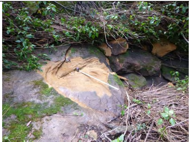
Photo 26: WCA5_LW38_001- fracturing with dislodged rock fragment. Taken on 24/04/2015
