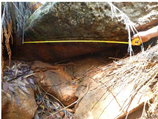
Photo 3: Impact WCA5_LW38_007- additional fracturing to boulder in GR110. Taken on 16/11/2015.
