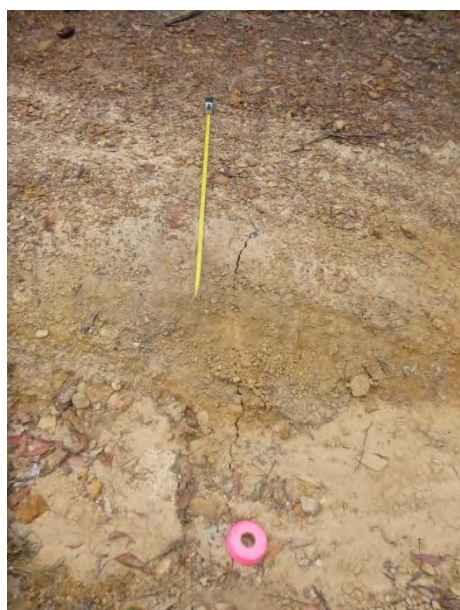
Photo 1: WCA5_LW38_006 – Soil crack looking across the fire trail. Taken on 25/9/15
