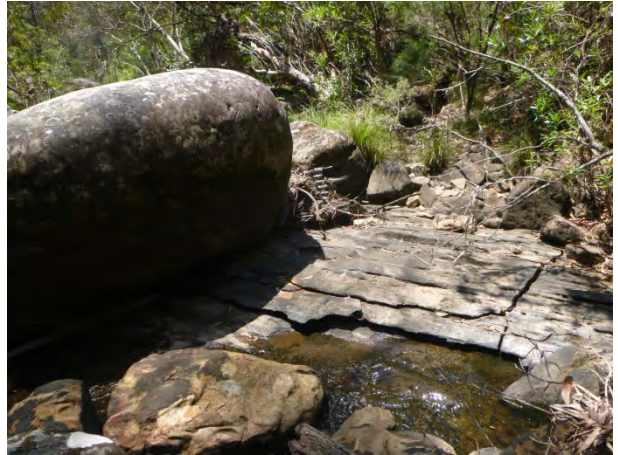
Photo 4: Impact WCA5_LW38_008- Fracturing identified on the Georges River. Taken on 10/12/2015.
