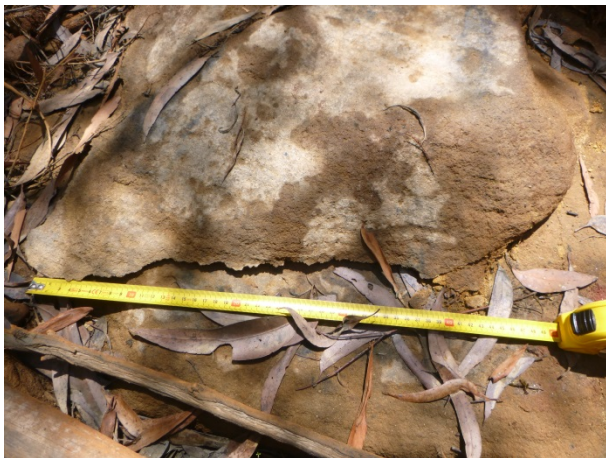
Photo 6: Impact WCA5_LW38_007, fracturing to base of GR110. Taken on 16/11/2015.
