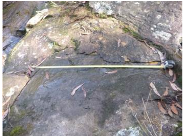
Photo 5: WCA5_LW38_005, fracturing and uplift downstream of Pool 1 in GR108. Taken on 20/08/2015.
