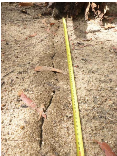
Photo 14: WCA5_LW38_011, soil crack on access track. Taken on 16/03/16.
