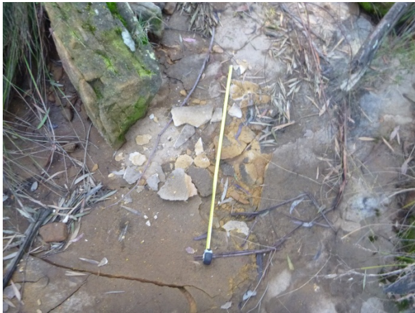
Photo 4: WCA5_LW38_003, fracturing and uplift within Channel 2, GR108. Taken on 03/08/2015.
