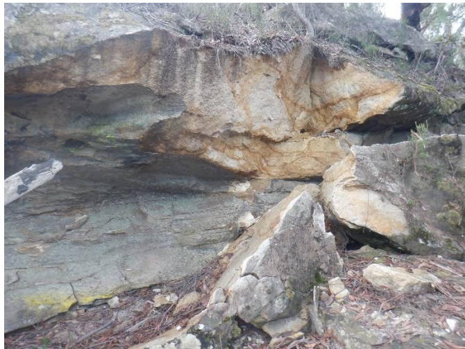
Photo 24: DA3B_LW18_022, Rock fall, northern slope of LA2 valley. Taken 16/8/2022.
