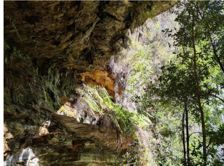
Photo 2: DA3B_LW17_041, Rockfall and Iron Staining at Waterfall 54, taken on 2/08/2022.
