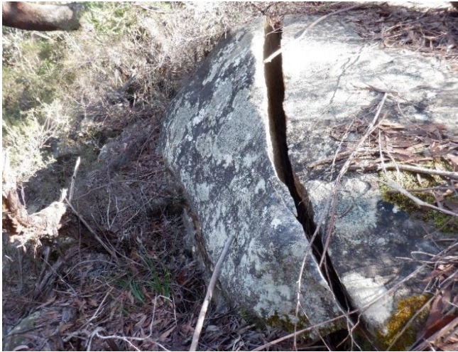
Photo 18: DA3B_LW18_016, Rock fracturing, northern slope of LA2 valley. Taken 16/8/2022.
