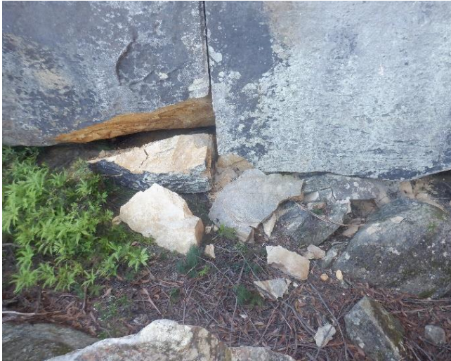
Photo 12: DA3B_LW18_010, Rockfall at 7m high cliffline, west of Fire Road 6A. Taken on 10/06/2022.
