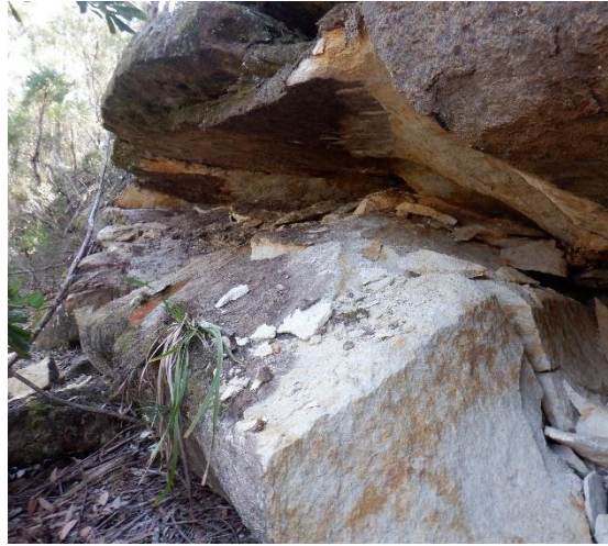
Photo 22: DA3B_LW18_020, Rock fall, northern slope of LA2 valley. Taken 16/8/2022.
