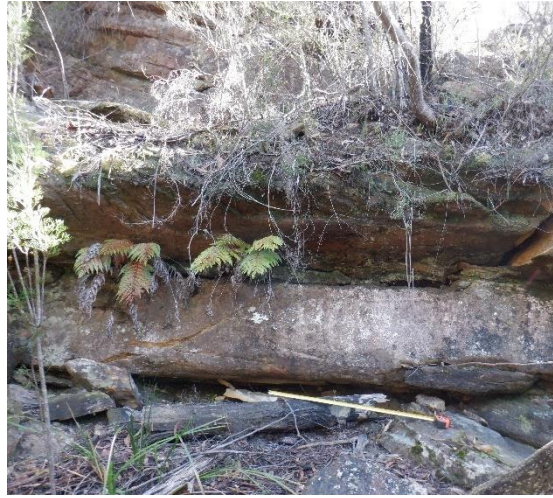
Photo 16: DA3B_LW18_014, Rock fracturing and rock fall, northern slope of LA2 valley. Taken 16/8/2022.
