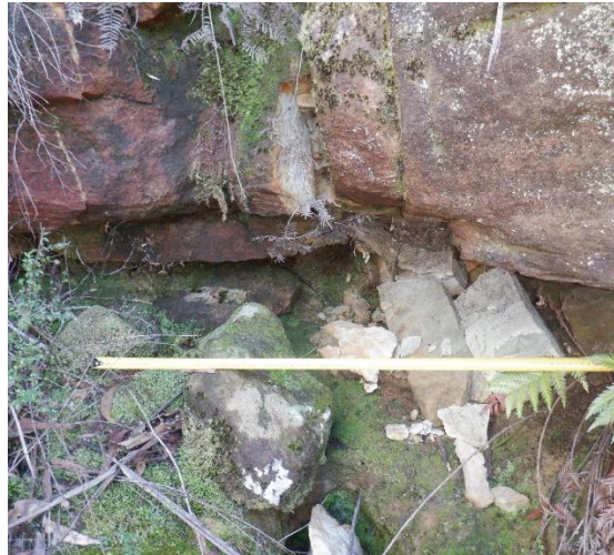
Photo 19: DA3B_LW18_017, Rock displacement and rock fall, northern slope of LA2 valley. Taken 16/8/2022.
