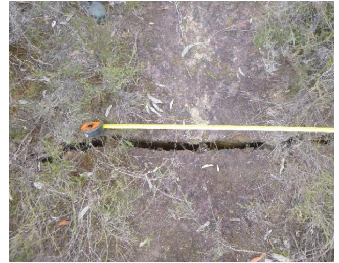
Photo 14: DA3B_LW18_012, Soil cracking near access track west of FR6A. Taken 30/6/2022
