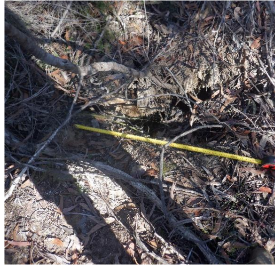
Photo 10: DA3B_LW18_008, Soil cracking near access track west of Fire Road 6A. Taken on 9/06/2022.
