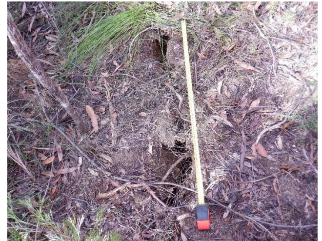
Photo 8: DA3B_LW18_006, Soil cracking to bushland near access track west of Fire Road 6A. Taken on 21/06/2022.
