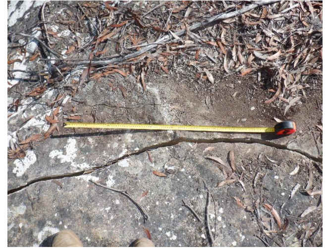
Photo 23: DA3B_LW18_021, Rock fracturing, Rock outcrop north of LA2 valley. Taken 16/8/2022.
