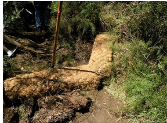
Plate 6-1 - Square Coir Logs for Knick Point Control
