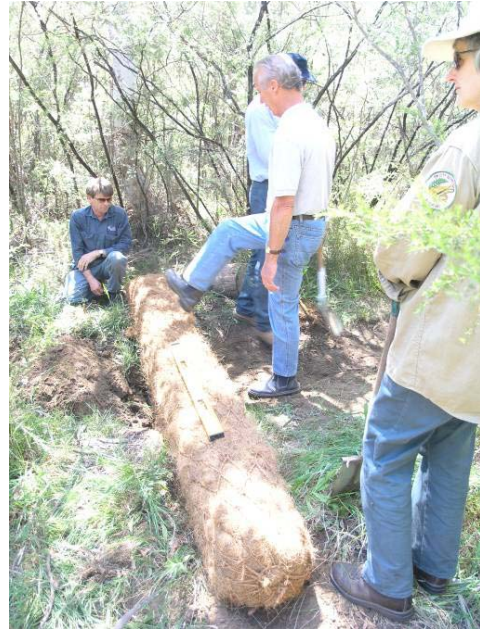
Plate 6-3 - Round Coir Logs Installed to Spread Water
