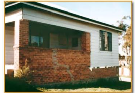
Inadequate footings ▲
