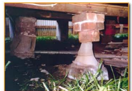
Inadequate footings ▲
