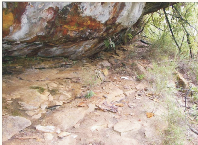
Plate 5: Site FRC 11 - Exfoliation and Block Fall from Rear Wall
