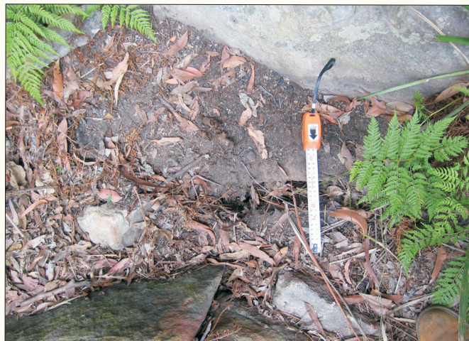
Plate 7b: Site D4 - Cracking in Soil outside Shelter
