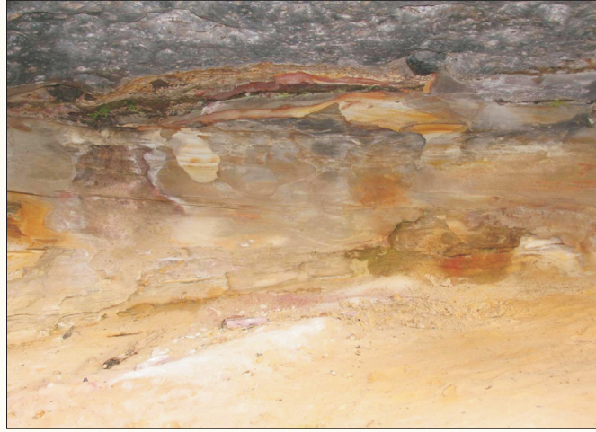
Plate 1: Site FRC 4 - Opening of Existing Bedding Plane at Rear Wall and Minor Roof Fall
