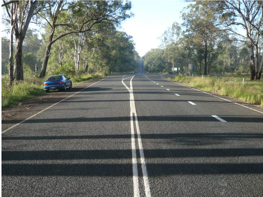
View looking south along Douglas Park Drive towards its intersection with the Appin West pit top access.
