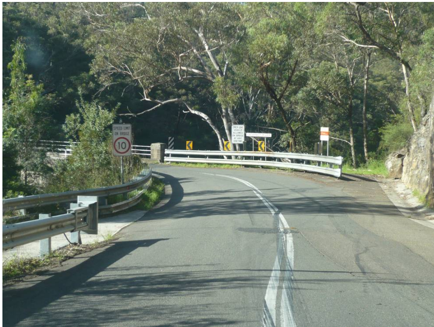
View looking east along Wilton Road on approach to the bridge at Broughtons Pass Weir.
