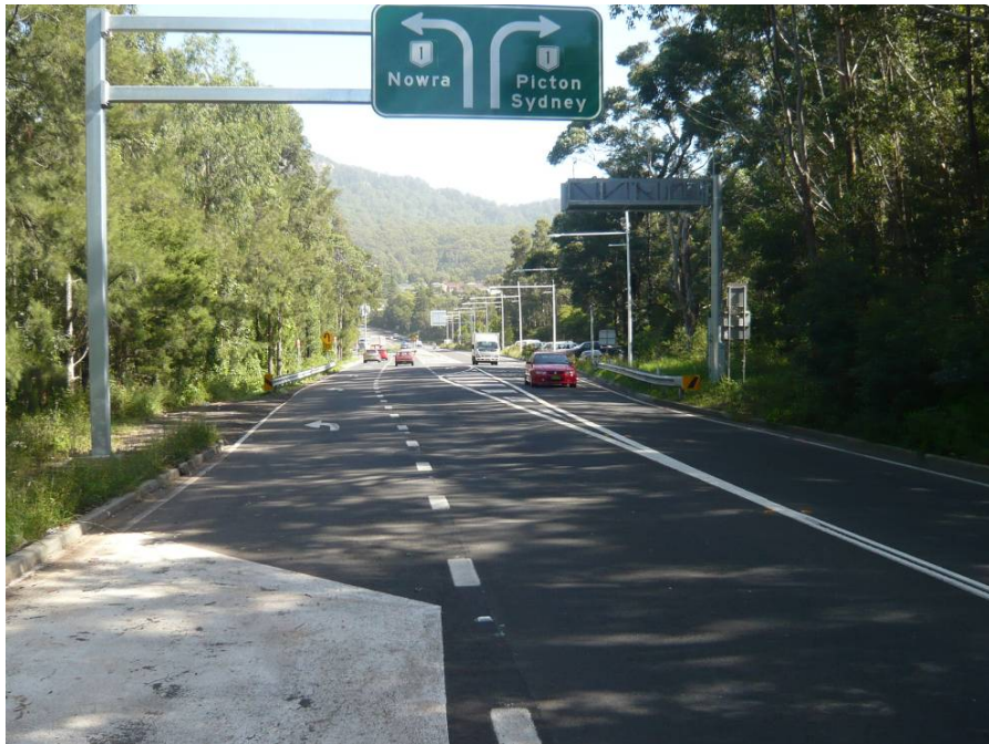
View looking west along Mount Ousley Road towards its interchange with the F6 Southern Freeway.
