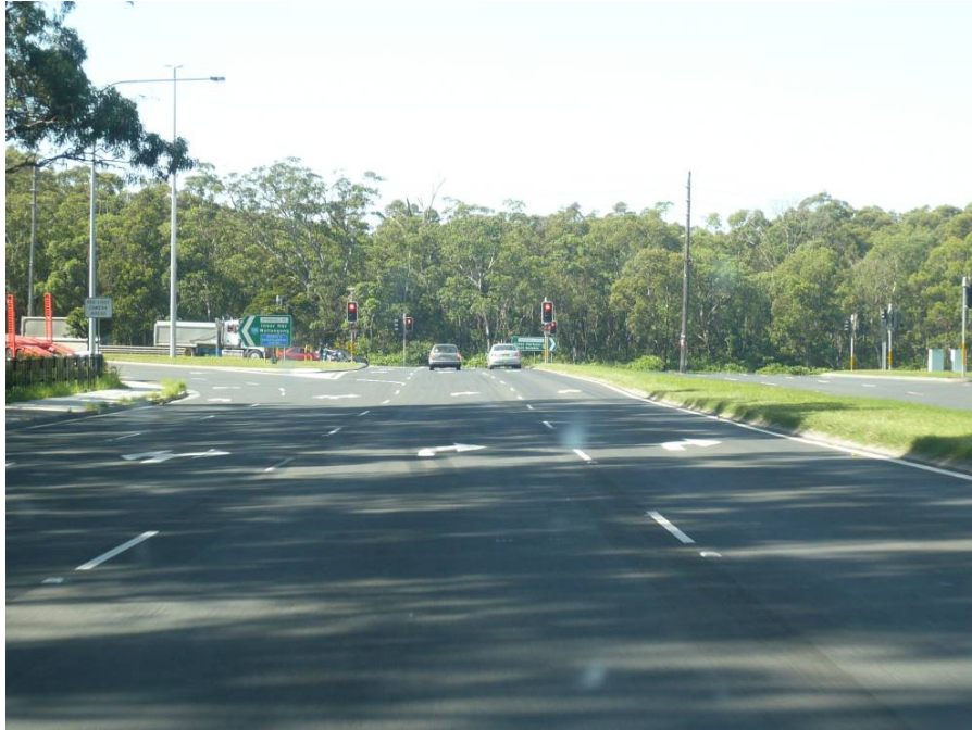
View looking east along Masters Road on approach to Springhill Road.
