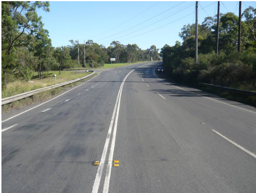
View looking west along Bulli-Appin Road towards the Appin East pit top entry.
