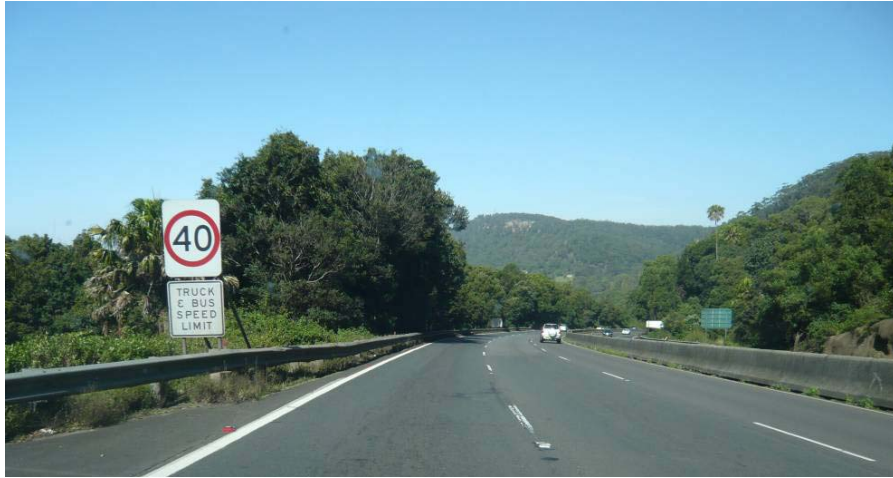
View looking south along Mount Ousley Road that indicates the bus and truck speed limit on this section of road.
