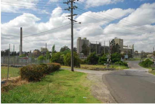
Maldon Cement Works. Photo: M. Pearson 2008
