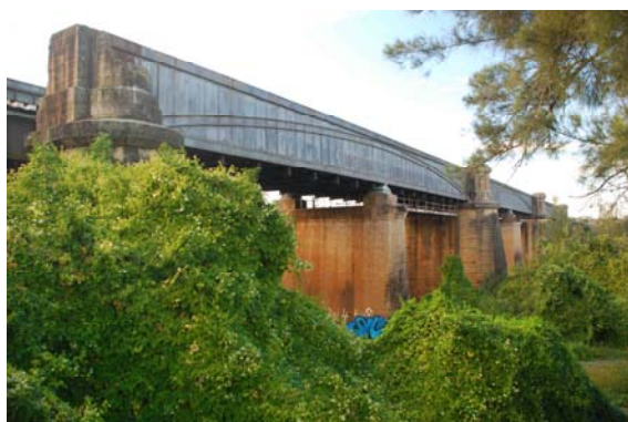
Menangle Rail Bridge Photo: M. Pearson 2008
