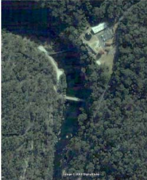
Broughtons Pass Weir, Google Earth image
