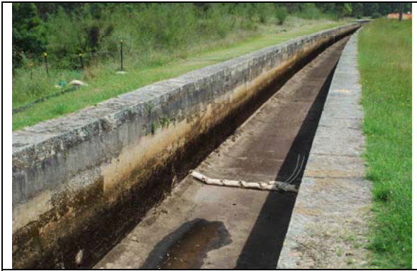
Upper Nepean canal, empty for maintenance. Photo: M. Pearson 2008.
