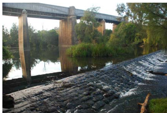
Menangle Rail bridge from Menangle Weir. Photo: M. Pearson 2008
