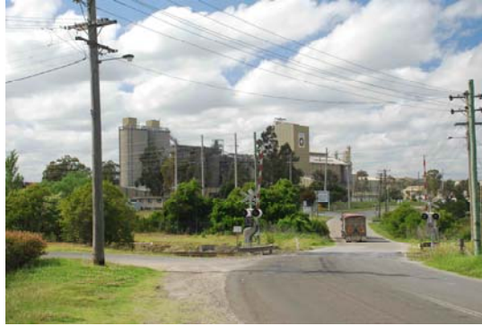
Maldon Cement Works. Photo: M. Pearson 2008
