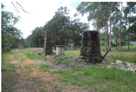
Nepean Tunnel above ground structures consist of survey plinths near former air shafts (these ones at eastern side of Wilton village)
