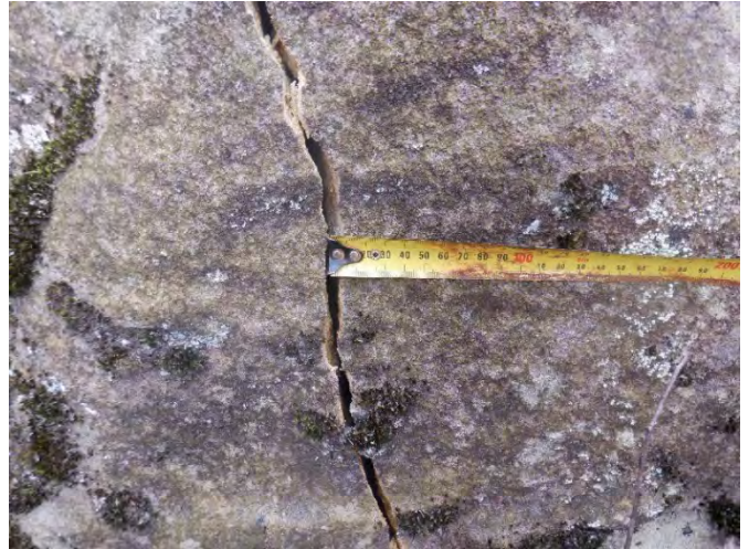
Photo 2: DA3C_LW21_012, maximum width of the rock fracture. Taken on 27/06/2023.
