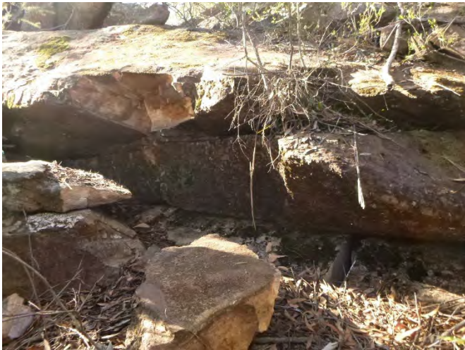
Photo 5: DA3C_LW21_007, fracturing and rock fall to outcrop. Taken on 15/06/2023.
