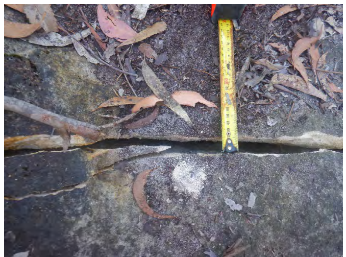
Photo 2: DA3C_LW21_008, maximum width of the rock fracture. Taken on 19/06/2023.
