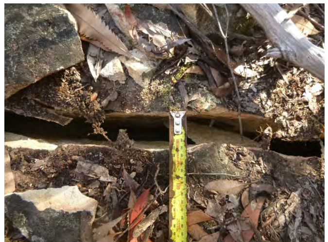
Photo 2: DA3C_LW21_005 , showing width of rock fracture. Taken on 15/06/2023
