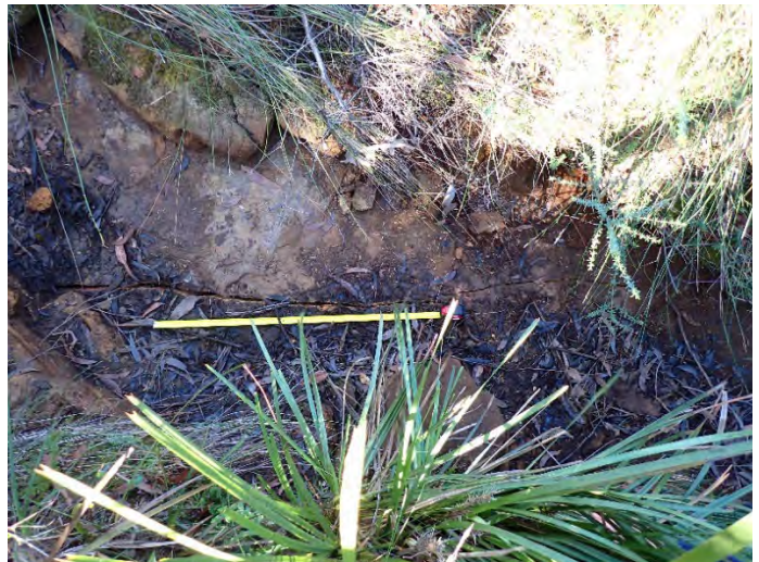
Photo 5: DA3C_LW21_015 , other section of rock fracturing. Taken on 11/07/2023.
