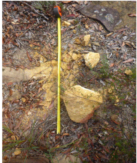
Photo 11: DA3C_LW21_003, showing rockfall debris. Taken on 06/06/2023.
