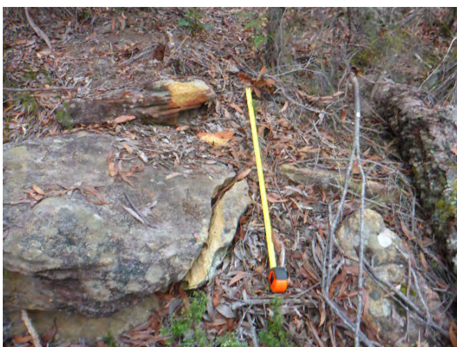
Photo 1: DA3C_LW21_001 , showing rock fracture. Taken on 06/06/2023.
