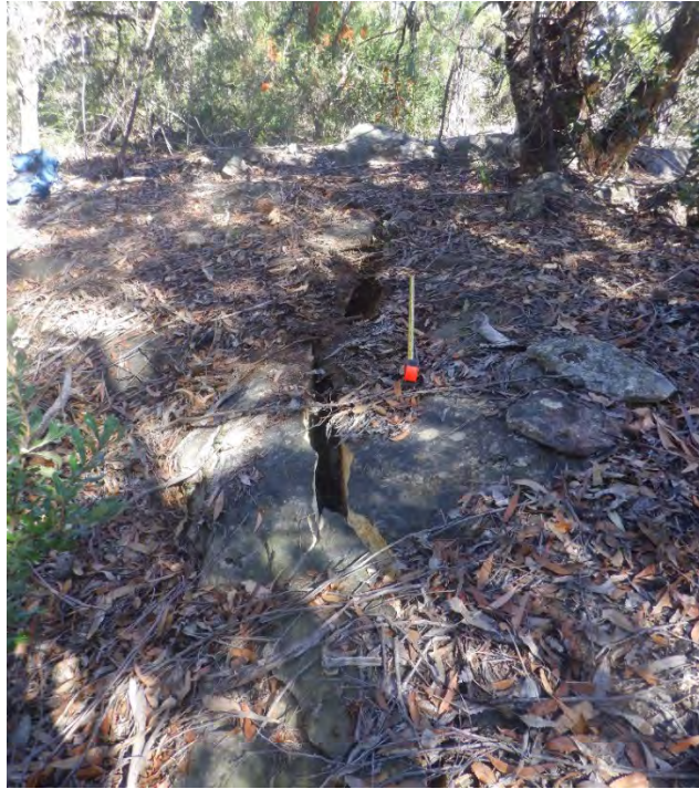
Photo 9: DA3C_LW21_010 , overview of the rock fracture. Taken on 19/06/2023.
