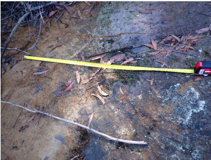
Photo 4: DA3C_LW21_015 , section of rock fracturing. Taken on 11/07/2023.
