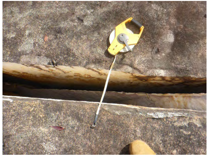
Photo 9: DA3C_LW21_003, width of rock fracture. Taken on 06/06/2023.
