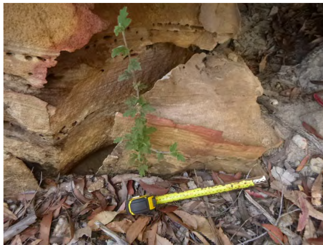
Photo 7: DA3C_LW21_007, rock fall. Taken on 15/06/2023.
