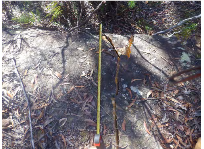
Photo 13: DA3C_LW21_011, section of rock fracturing and rock displacement. Taken on 19/06/2023.
