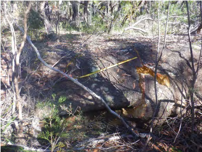
Photo 12: DA3C_LW21_011, section of rock fracturing and rock displacement. Taken on 19/06/2023.
