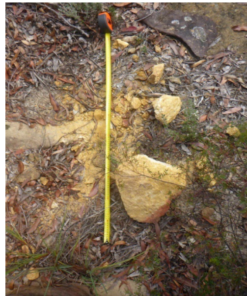
Photo 45: DA3C_LW21_003, showing rockfall debris. Taken on 06/06/2023.
