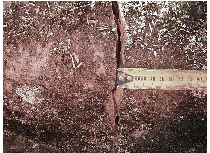
Photo 59: DA3C_LW21_009, maximum width of the rock fracture. Taken on 19/06/2023.
