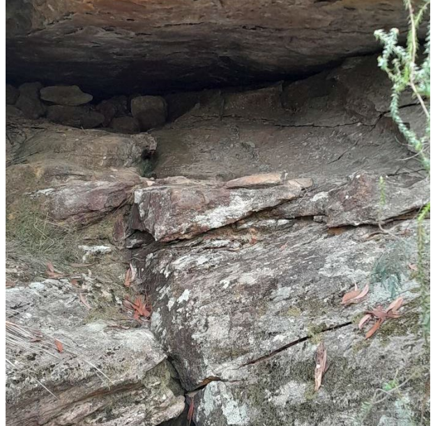
Photo 110: DA3C_LW21_032 , overview of fracturing to rock step/overhang. Taken 12/09/2023.
