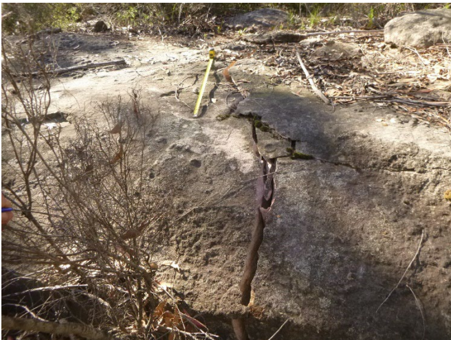
Photo 50: DA3C_LW21_006 , fracturing to rock outcrop. Taken on 15/06/2023.
