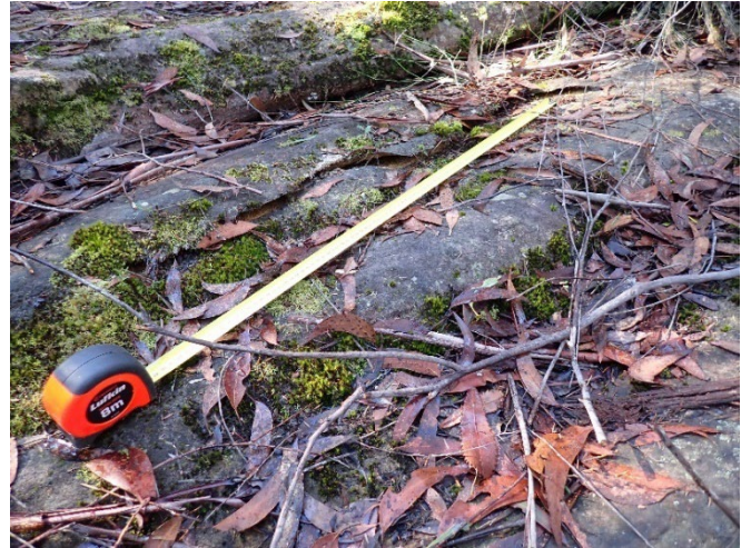
Photo 28: DA3C_LW21_017, section of rock fracturing. Taken on 26/07/2023.
