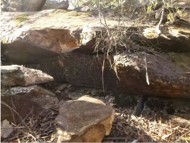
Photo 52: DA3C_LW21_007, fracturing and rock fall to outcrop. Taken on 15/06/2023.
