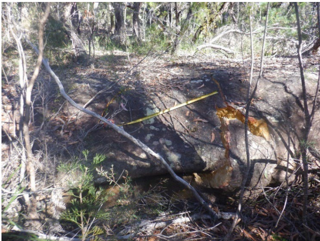
Photo 66: DA3C_LW21_011, section of rock fracturing and rock displacement. Taken on 19/06/2023.
