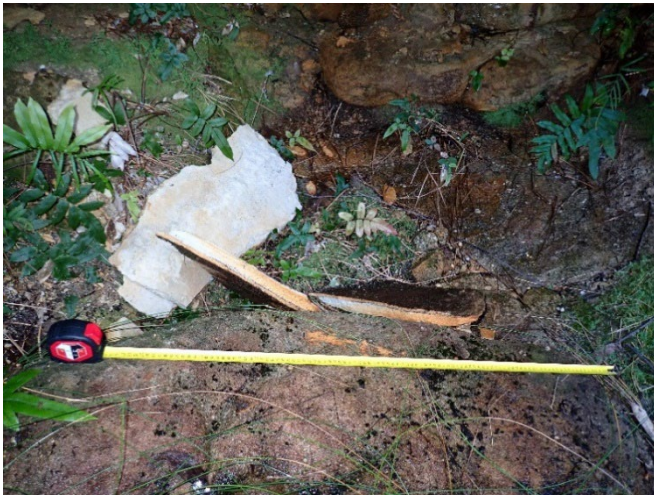
Photo 74: DA3C_LW21_016 , fragments of rockfall from step. Taken on 11/07/2023.
