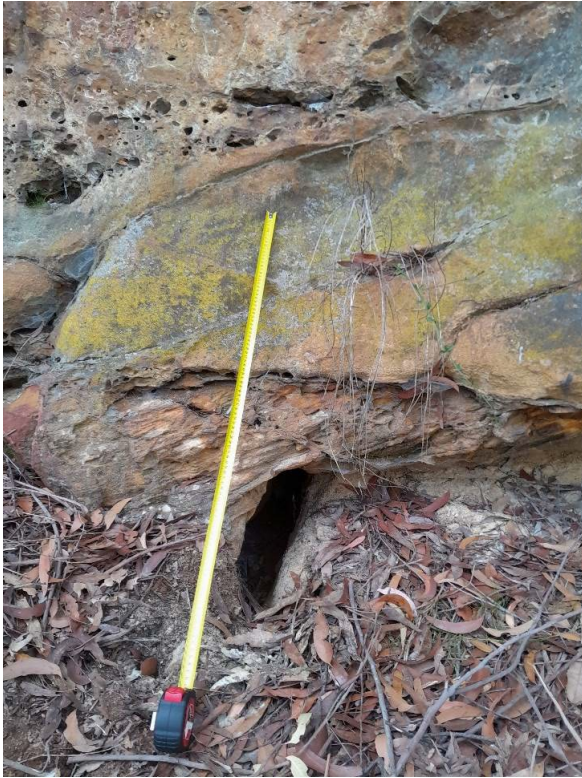
Photo 113: DA3C_LW21_034 overview of rock movement and soil crack. Taken: 12/09/2023.
