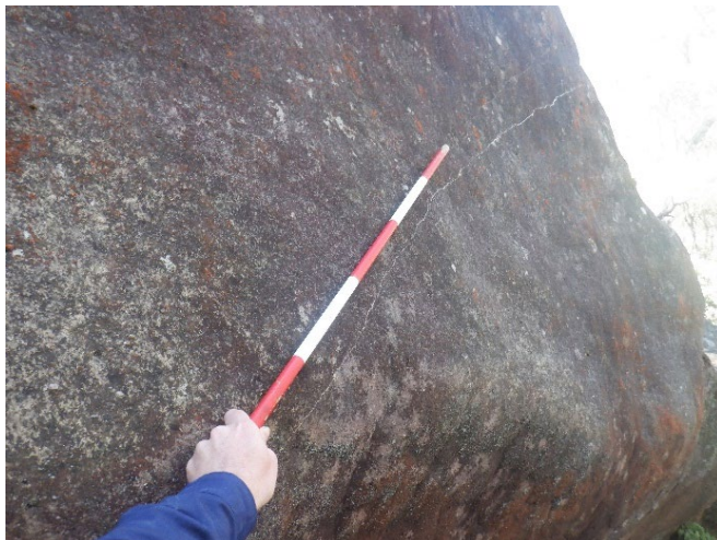
Photo 103: DA3C_LW21_029 , section of rock fracture. Taken 6/09/2023.
