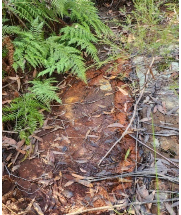
Photo 35: DA3C_LW21_020 , section of iron staining in WC24_Rockbar 15 . Taken on 1/08/2023.
