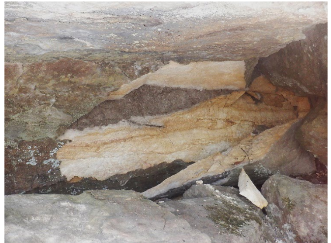
Photo 96: DA3C_LW21_026, close-up section of rockfall. Taken 06/09/2023.
