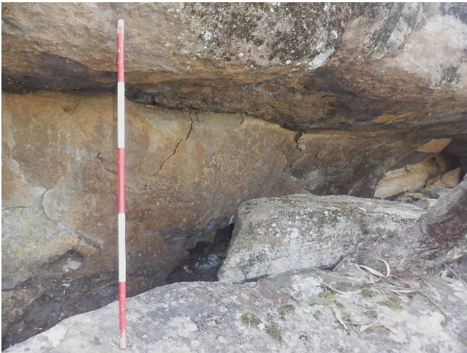
Photo 95: DA3C_LW21_026, section of rock fracture and rockfall. Taken 06/09/2023.
