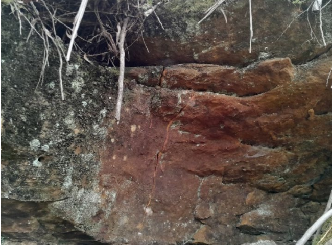
Photo 109: DA3C_LW21_032 , overview of fracturing to rock step/overhang. Taken 12/09/2023.
