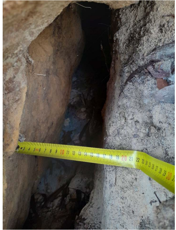
Photo 114: DA3C_LW21_034 width of soil crack. Taken 12/09/2023.
