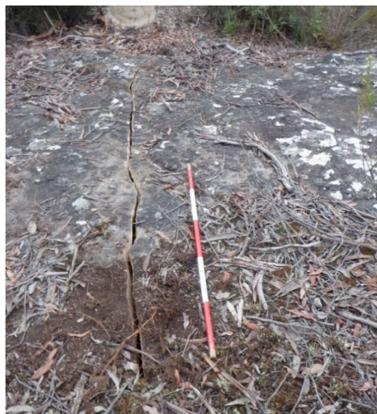
Photo 73: DA3C_LW21_013, overview of section of impact. Taken on 03/07/2023.
