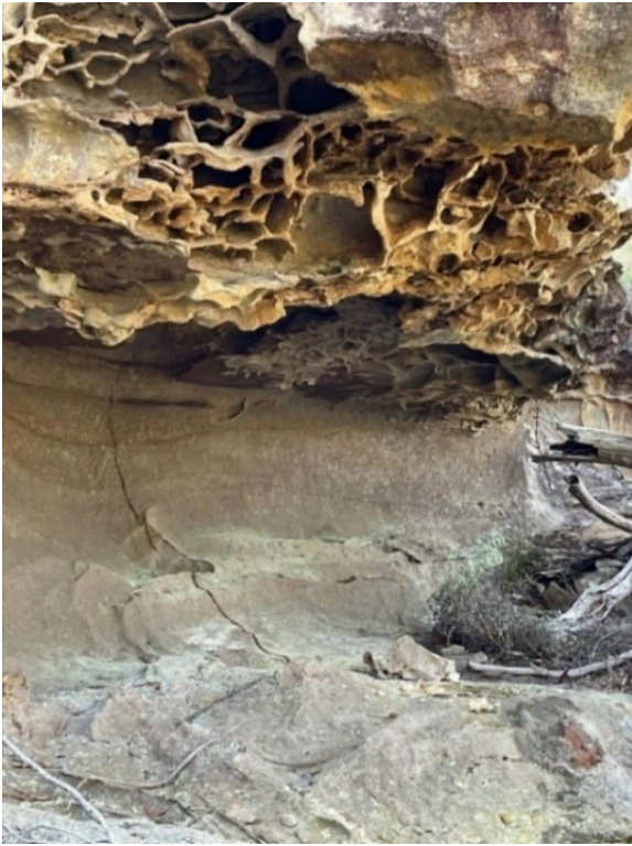
Photo 92: DA3C_LW21_025 , section of the rock fracture in overhang. Taken: 06/09/2023.
