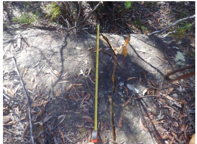
Photo 67: DA3C_LW21_011, section of rock fracturing and rock displacement. Taken on 19/06/2023.
