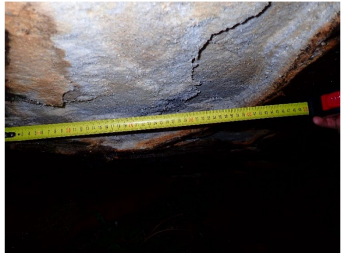
Photo 75: DA3C_LW21_016 , underside of step from which rock fragments fell. Taken on 11/07/2023.
