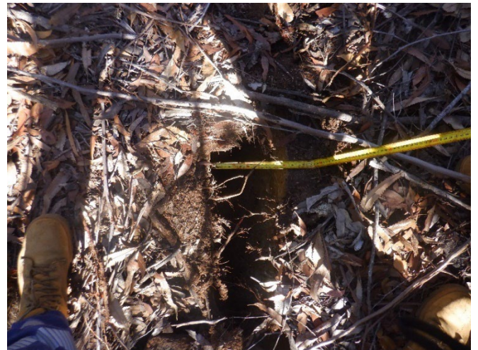
Photo 62: DA3C_LW21_010, maximum width of the rock fracture. Taken on 19/06/2023.
