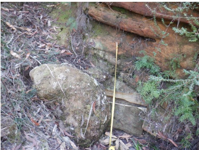
Photo 151: DA3A_LW19_053, showing area of rockfall. Taken on 4/5/2023.
