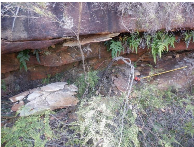
Photo 101: DA3A_LW19_027, section of rock fracturing and rockfall. Taken on 10/01/2023.
