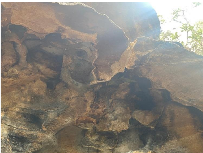
Photo 126: DA3A_LW19_038, section where rock fall occurred. Taken on 28/03/2023.
