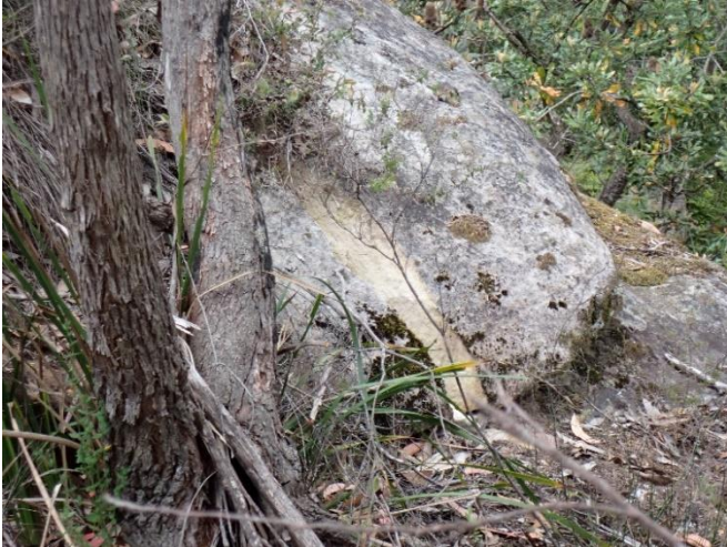
Photo 93: DA3A_LW19_024, section of rock fracturing. Taken on 20/12/2022.
