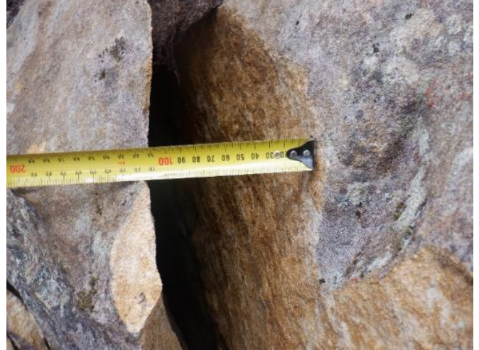
Photo 66: DA3A_LW19_013, width of rock fracturing. Taken on 7/11/2022.
