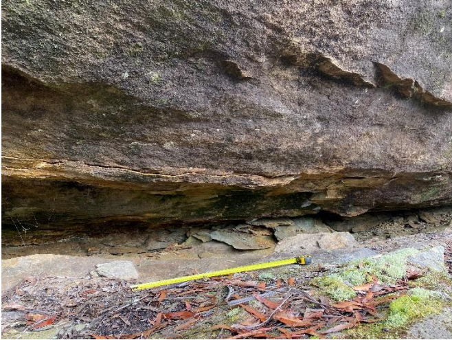
Photo 116: DA3A_LW19_037, rock fracturing. Taken on 28/03/2023.
