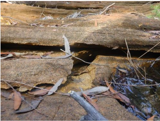
Photo 24: DA3A_LW19_043, looking at rock fracturing across rockbar. Taken 17/04/2023.
