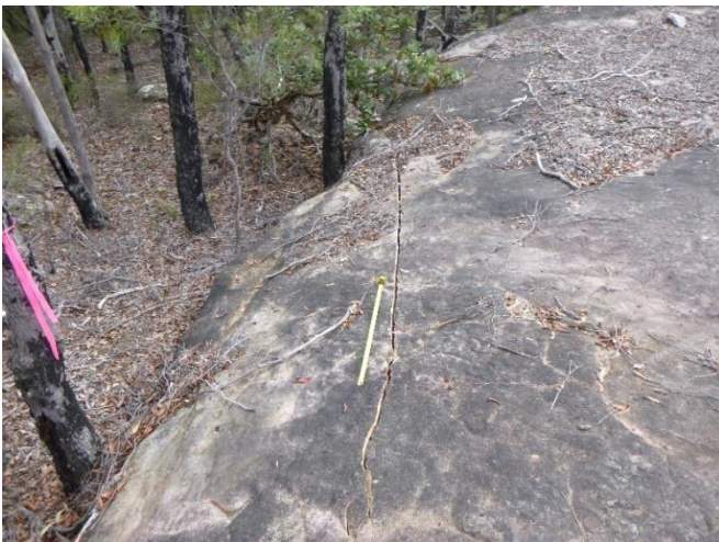
Photo 105: DA3A_LW19_030, rock fracturing to an outcrop. Taken on 15/2/2023.
