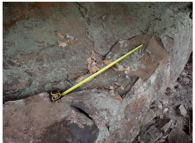
Photo 141: DA3A_LW19_042 looking at rockfall and associated fragments. Taken 12/04/2023.
