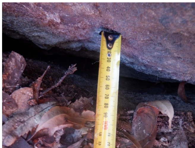
Photo 79: DA3A_LW19_019, width of rock displacement. Taken on 13/12/2022.
