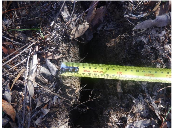
Photo 186: DA3A_LW19_049, showing width of soil crack. Taken on 27/04/2023.
