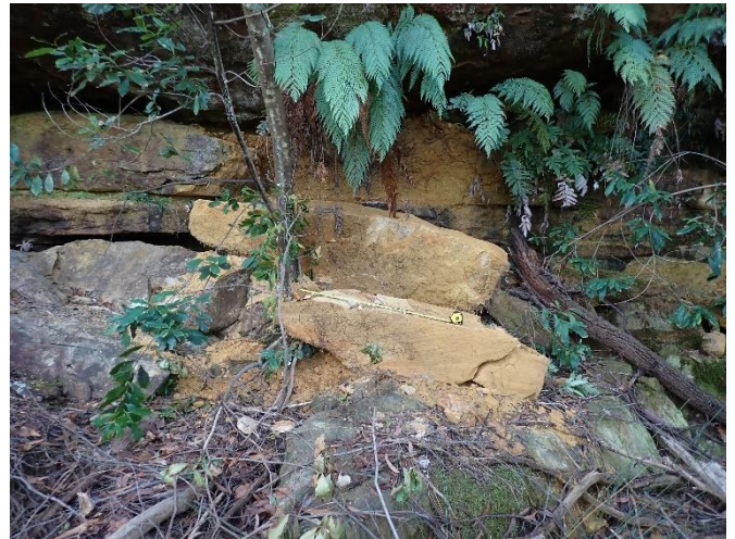
Photo 131: DA3A_LW19_039 , looking at the rockfall. Taken 12/04/2023
