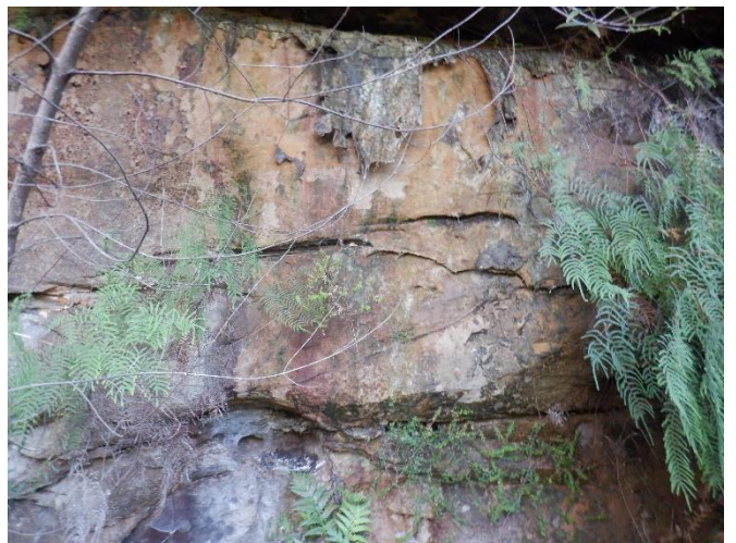
Photo 150: DA3A_LW19_052, showing area of rock fracturing. Taken on 4/5/2023.
