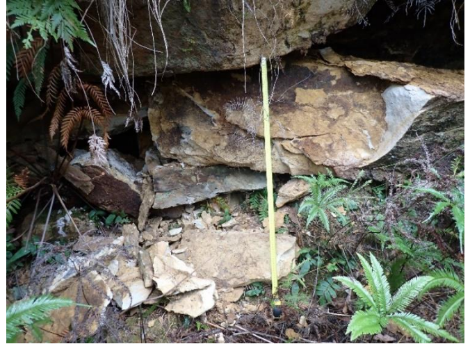
Photo 133: DA3A_LW19_040, looking at rockfall and fragments. Taken 12/04/2023.
