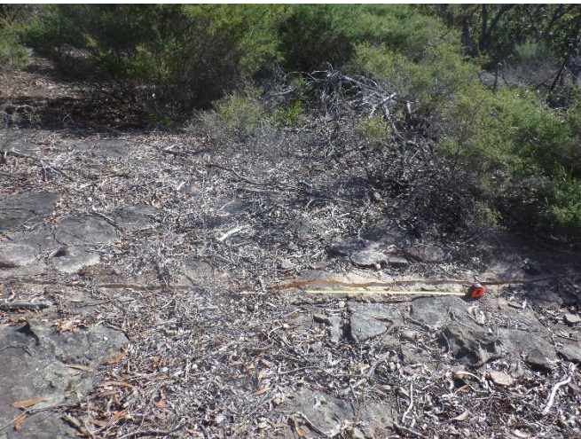
Photo 54: DA3A_LW19_008, section of rock fracturing taken on 09/05/2023.
