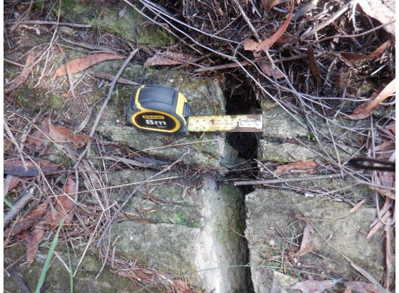
Photo 31: DA3A_LW19_051, showing width of rock fracture. Taken on 4/5/2023.
