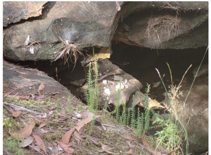
Photo 29: DA3A_LW8_003, looking at the rockfall and associated fragments. Taken on 12/04/2023.
