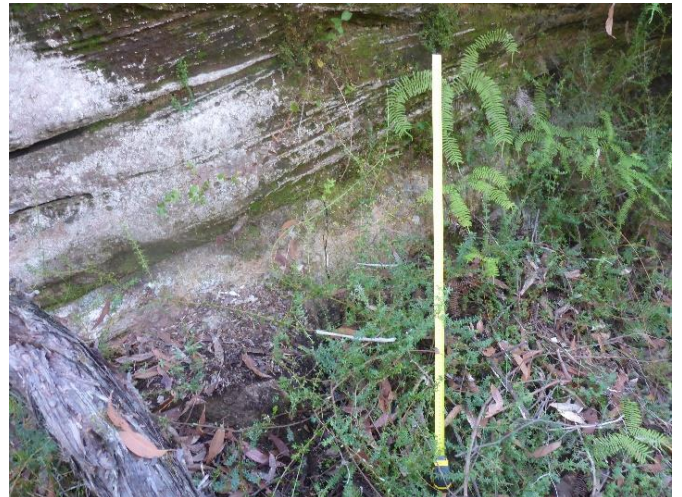
Photo 171: DA3A_LW19_062, showing extent of rock fracture. Taken on 05/05/2023.
