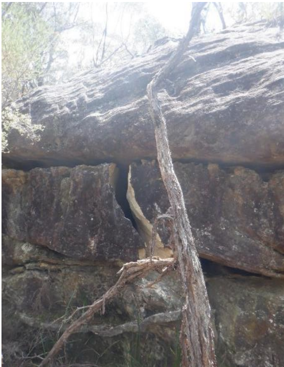
Photo 69: DA3A_LW19_015, section of rock fracturing. Taken on 7/11/2022.
