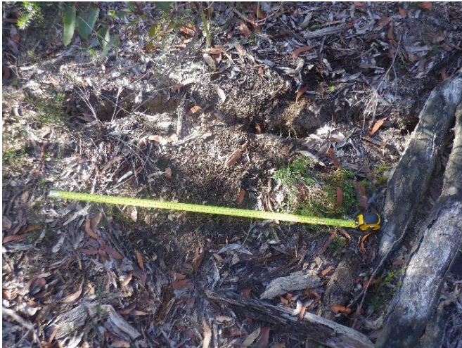
Photo 185: DA3A_LW19_049, showing extent of soil crack. Taken on 27/04/2023.
