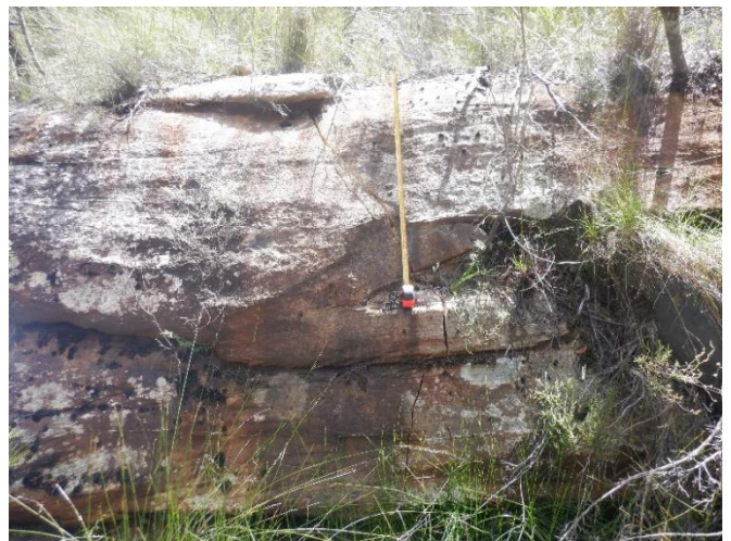
Photo 102: DA3A_LW19_027, section of rock fracturing. Taken on 10/01/2023.
