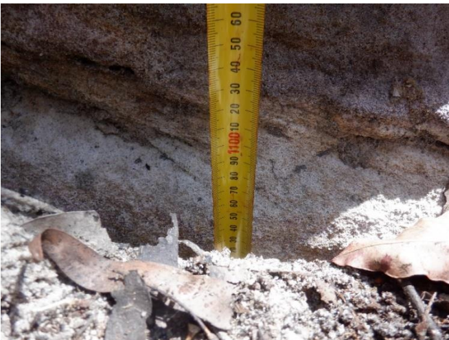
Photo 85: DA3A_LW19_021, depth of soil cracking. Taken on 13/12/2022.
