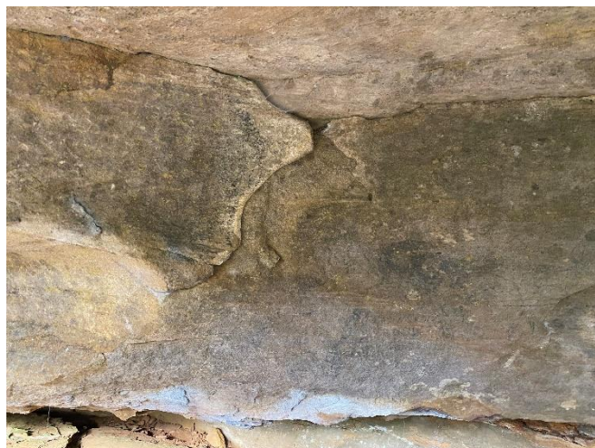
Photo 123: Sandy Creek 21 showing no impacts to artwork following Longwall 19. Taken on 28/03/2023.
