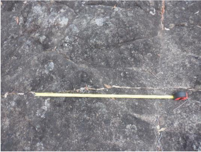
Photo 63: DA3A_LW19_012 , section of rock fracturing. Taken on 7/11/2022.
