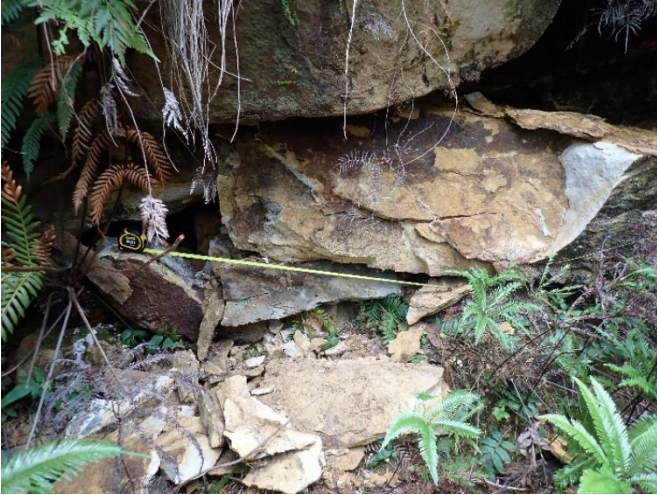
Photo 132: DA3A_LW19_040, looking at rockfall and fragments. Taken 12/04/2023.
