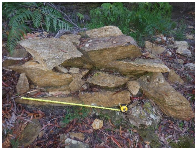
Photo 146: DA3A_LW19_046, showing debris area. Taken on 27/04/2023.
