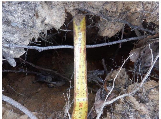
Photo 96: DA3A_LW19_024, width of soil crack after erosion. Taken 19/04/2023.
