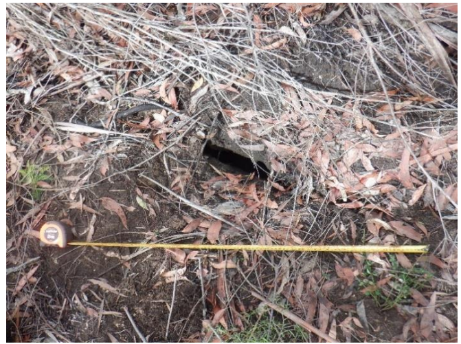
Photo 181: DA3A_LW19_036, soil cracking. Taken on 21/03/2023.
