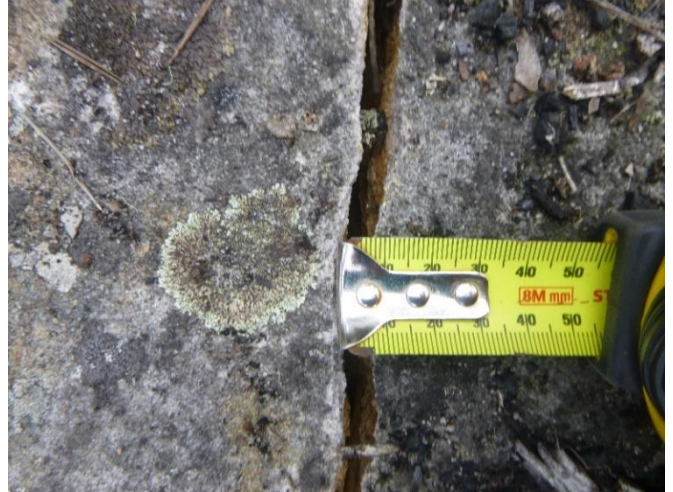
Photo 108: DA3A_LW19_031 , width of rock fracture on outcrop. Taken on 15/2/2023
