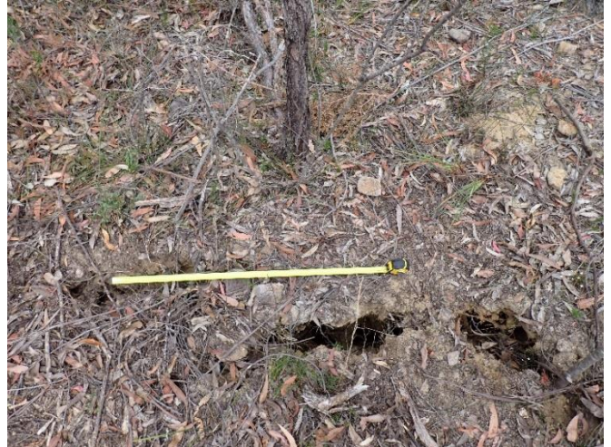
Photo 94: DA3A_LW19_024, section of soil cracking. Taken on 20/12/2022.
