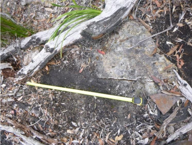
Photo 107: DA3A_LW19_031 , rock fracturing to an outcrop. Taken on 15/2/2023
