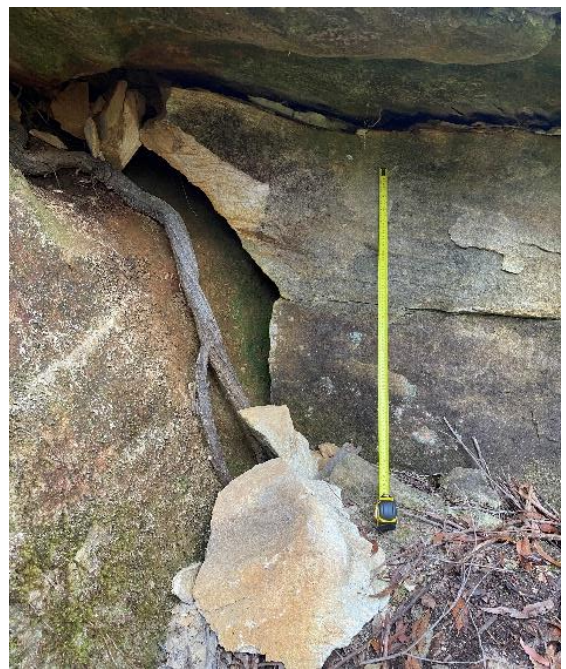
Photo 119: DA3A_LW19_037, rock fall. Taken on 28/03/2023.
