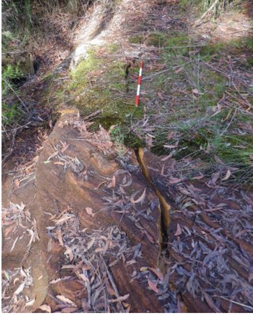
Photo 22: DA3A_LW19_043, looking at rock Fracturing on rockbar. Taken 17/04/2023.
