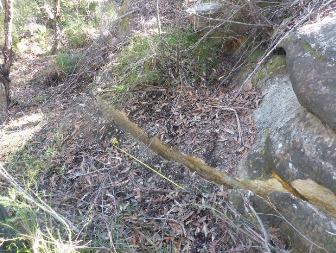
Photo 168: DA3A_LW19_061, showing extent of rock fracture. Taken on 05/05/2023.
