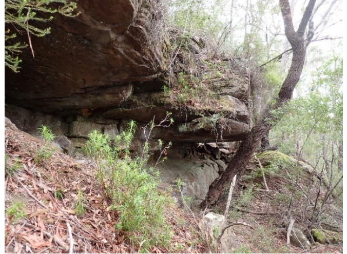
Photo 139: LW19_SS4 during its most recent inspection. Taken 12/04/2023.
