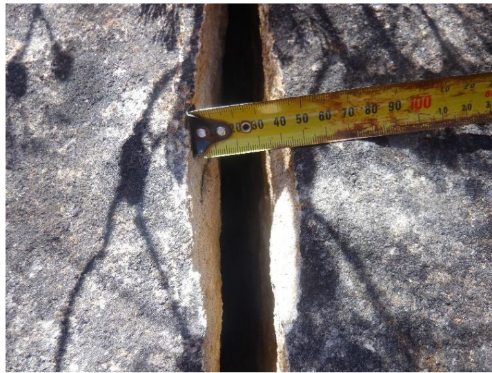
Photo 58: DA3A_LW19_009, width of rock fracturing. Taken on 09/05/2023.
