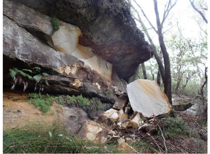
Photo 135: DA3A_LW19_041 looking at the rockfall at landscape site LW19_SS5 . Taken 12/04/2023.
