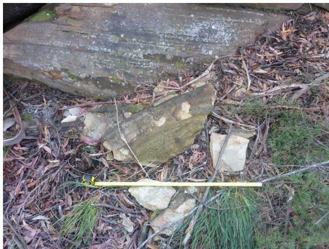
Photo 167: DA3A_LW19_060, showing rockfall. Taken on 5/05/2023
