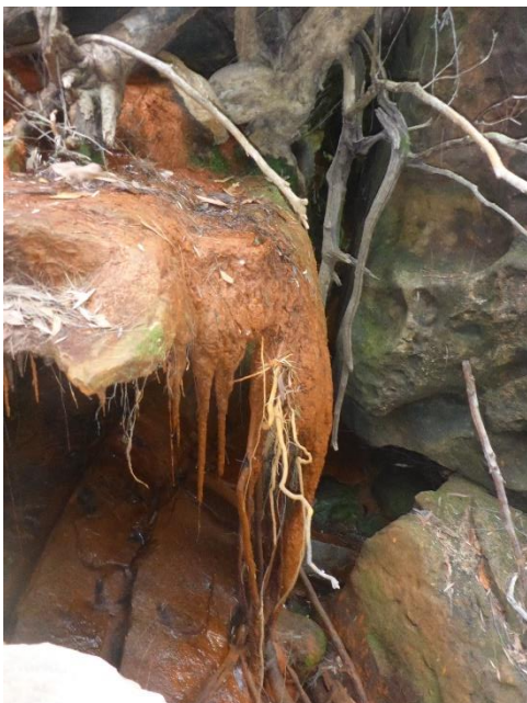
Photo 18: WC14_Step 3, looking at the iron staining. Taken on 28/01/2020.
