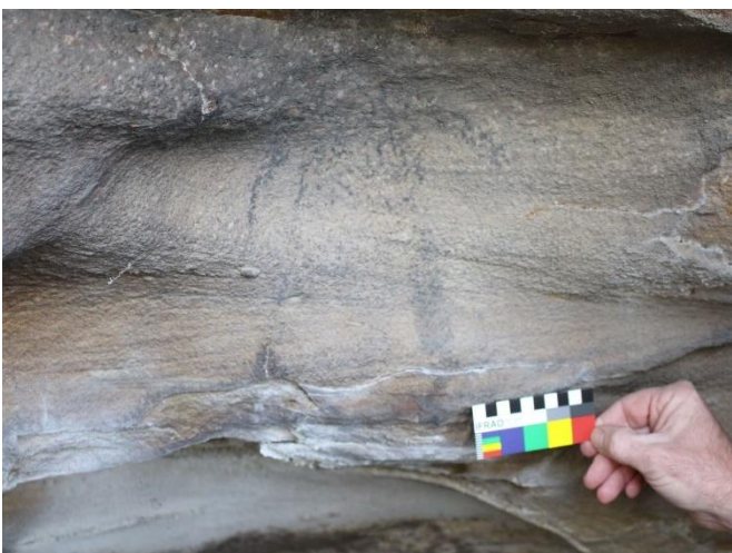
Photo 128: Art at DM15- baseline image displaying horizontal rock fracture identified prior to mining. Taken circa October 2020.
