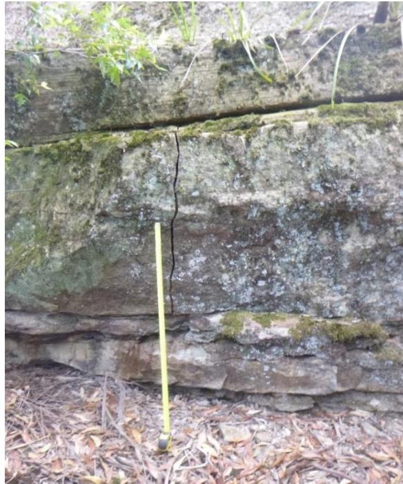
Photo 110: DA3A_LW19_032, rock fracturing on side of outcrop. Taken on 15/2/2023.
