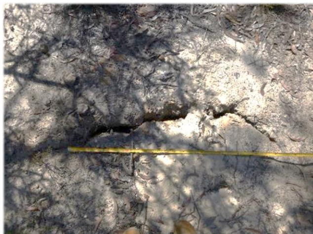
Photo 63: DA3B_LW13_032, soil cracking across Fire Road 6P. Taken 9 th April 2018.
