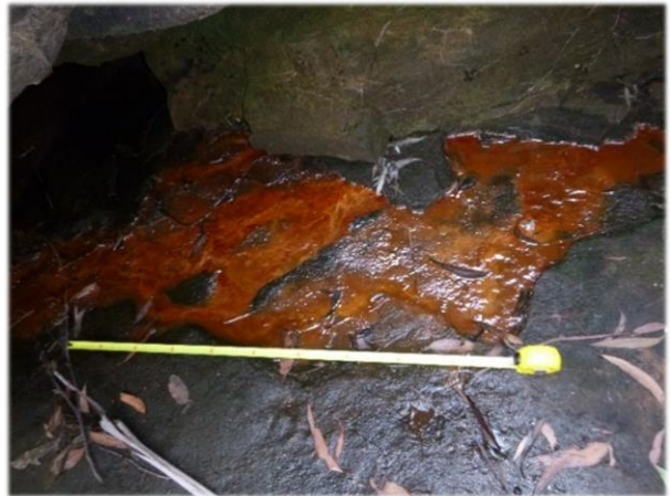
Photo 39: DA3B_LW13_042 , looking at a section of iron staining. Taken 16th May 2018.
