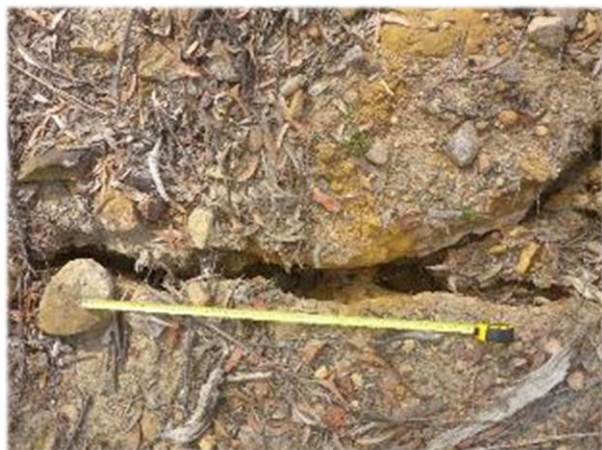
Photo 69: DA3B_LW13_024, looking across track. Taken 4 th March 2018.
