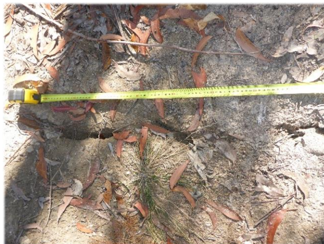
Photo 64: DA3B_LW13_012, largest section of surface cracking. Taken on 30/10/2017.
