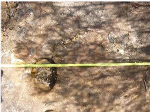
Photo 13: DA3B_LW13_021, looking at the small section plating. Taken 29 th March 2018.
