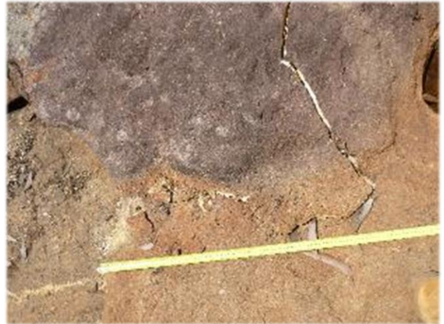
Photo 12: DA3B_LW13_021, looking at the widest section of fracturing. Taken 29 th March 2018.
