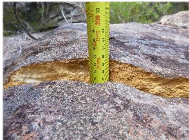
Photo 22: DA3B_LW13_023, closeup of the deepest section of fracturing. Taken 29 th March 2018.
