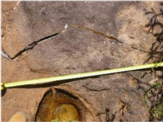
Photo 11: DA3B_LW13_021, looking at the widest section of fracturing. Taken 29 th March 2018.
