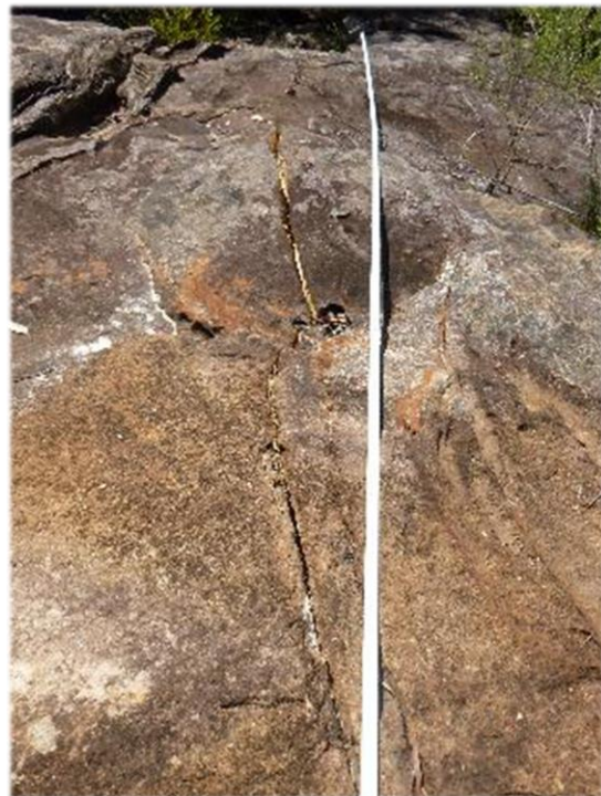
Photo 16: DA3B_LW13_022, looking downstream towards longest fracture. Taken 29 th March 2018.
