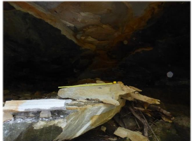
Photo 34: DA3B_LW13_041, looking the accumulation of rock that resulted from the rockfall. Taken 7 th May 2018
