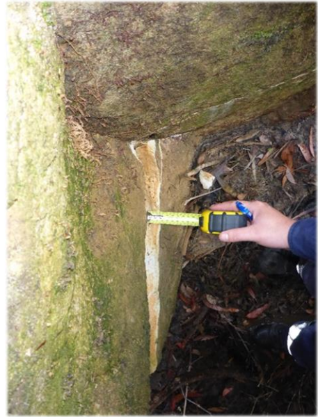
Photo 47: Impact DA3B_LW13_010 looking top-down at the displaced rock, taken 27/10/2017.
