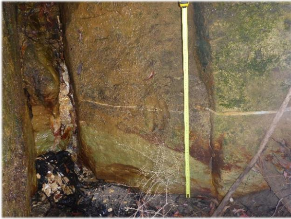
Photo 46: Impact DA3B_LW13_010 looking upstream, taken 27/10/2017.
