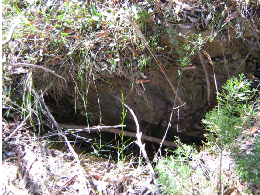
Photo 3 - Remnant 600 mm Wide Crack in Area 1 (2 years since mining of LWs 1 & 2)
