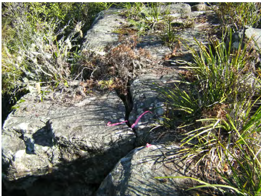
Photo 10 - Cliff Crest Cracking above Area 2 Steep Slope (SL1)
