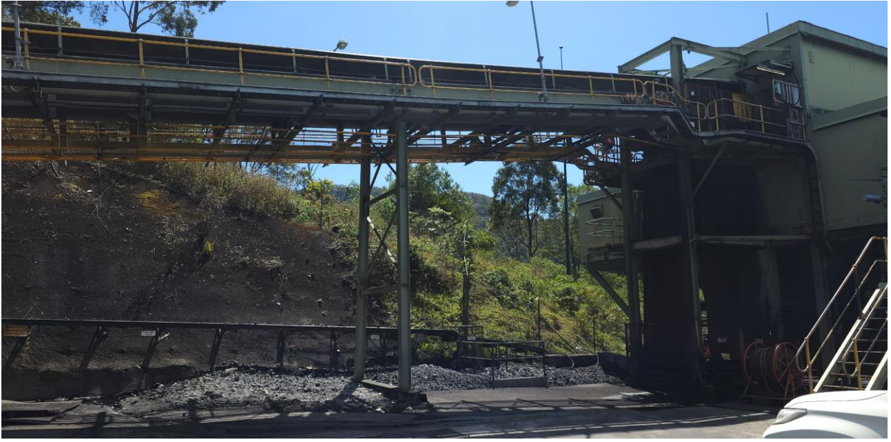
KVCLF – Stockpile, coal conveyor and rill tower
