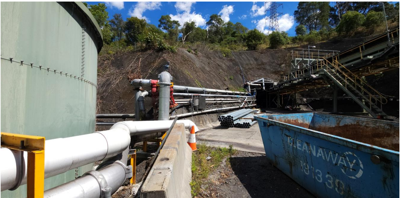
KVCLF – Groundwater pipeline and turbidity probe
