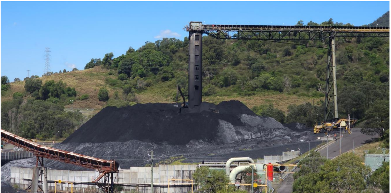
KVCLF – Stockpile, coal conveyor and rill tower
