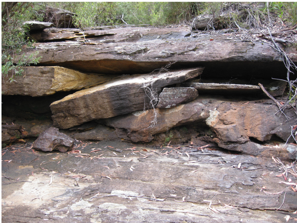
Photo 6 - Rock Shelf Collapse on Watercourse WC17 in Area 3A
