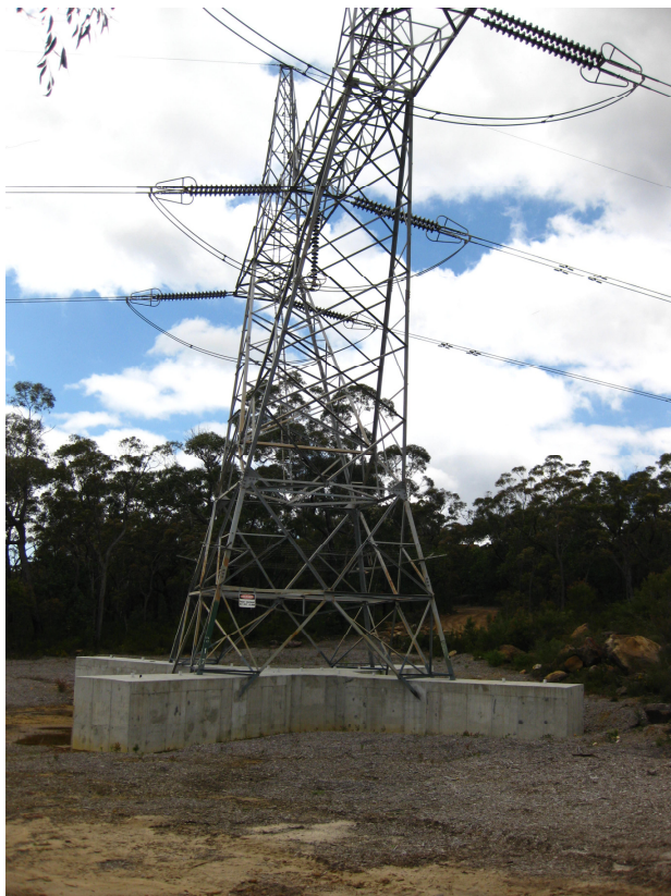
Photo 12 - Cruciform Footings Installed on Measured Subsidence Contours in Area 2
