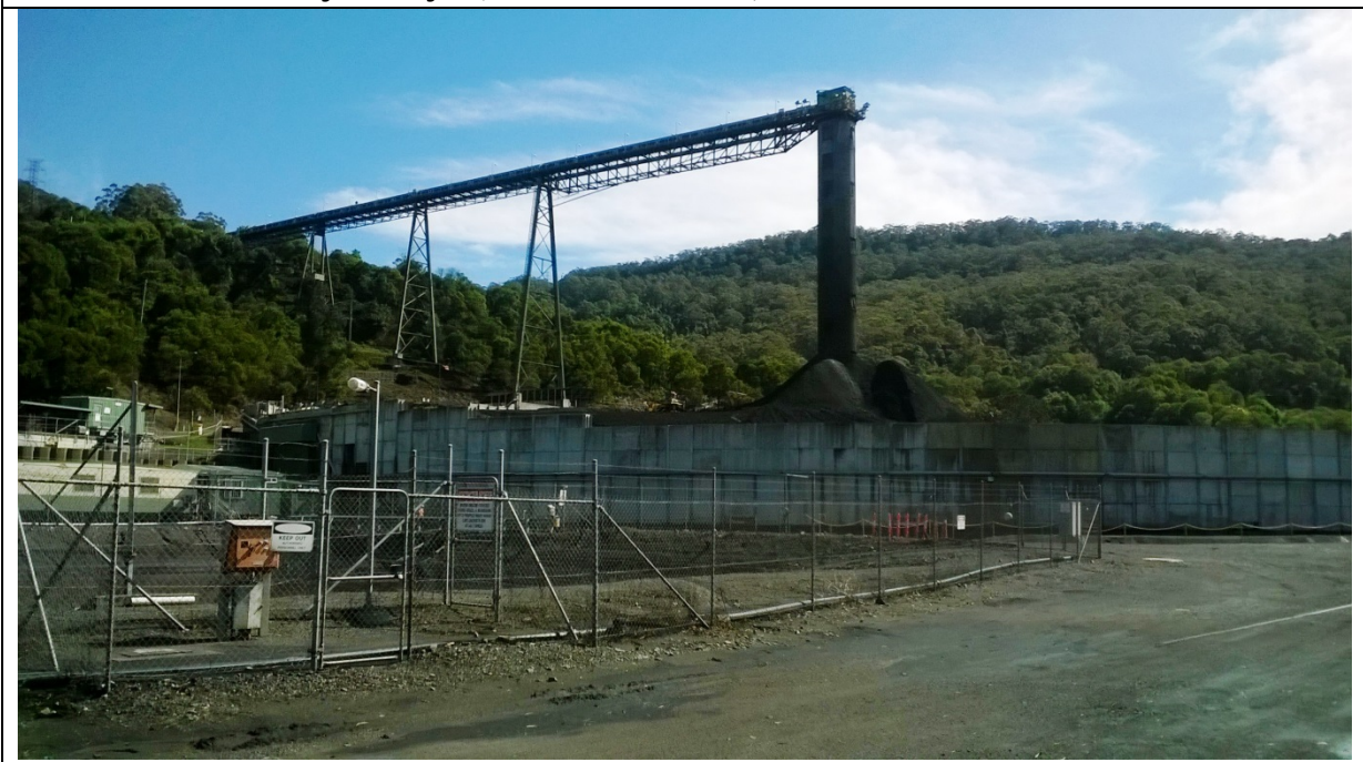
Picture E6: Kemira Valley Coal loading facility (view north to stockpile area)
