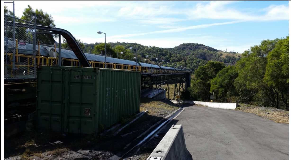
Picture E5: Kemira Valley conveyor (view east to rill tower)
