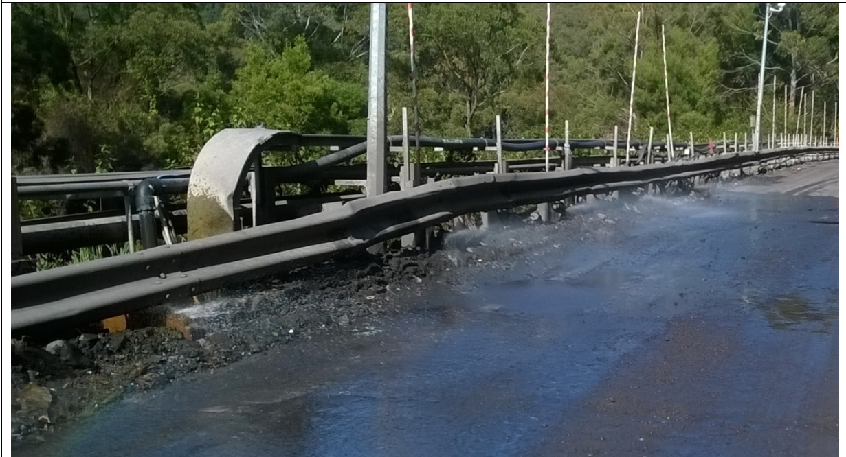
Picture E2: Dust suppression in operation (Dendrobium Colliery Pit top access road)
