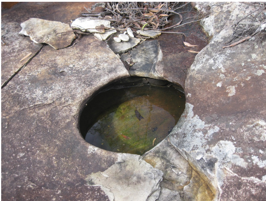
Photo 2 - Cracked Pond Rock Bar after recent rains along 1st Order Creek No. SC10C, Area 3A (>2 years since mining of LW 7)
