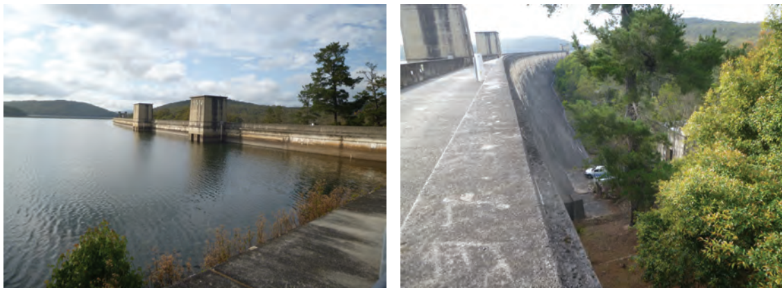
Fig. 6.9 Cordeaux Dam Wall
