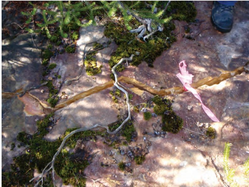
Fig. 5.15 Fracturing in the rockbar downstream of Swamp Den01 (Source: IMC)
