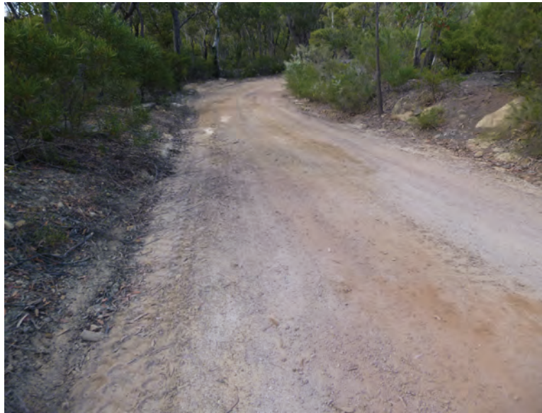
Fig. 6.1 Typical unsealed road
