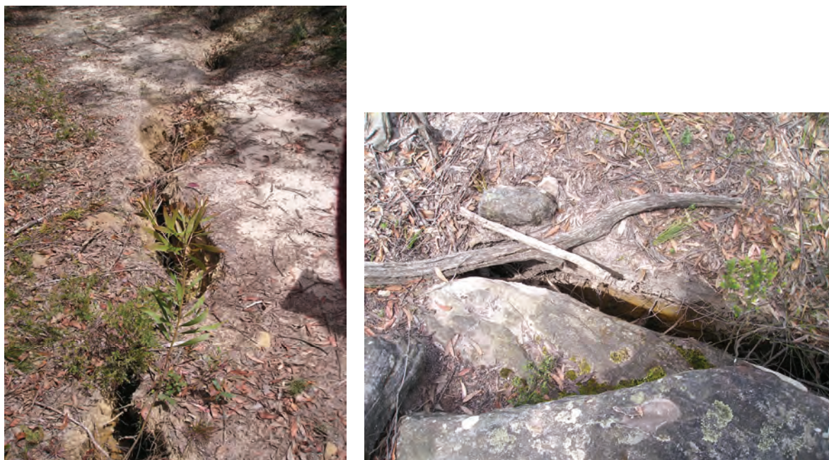
Fig. 5.12 Surface tension cracking due to downslope movements at Dendrobium Mine
