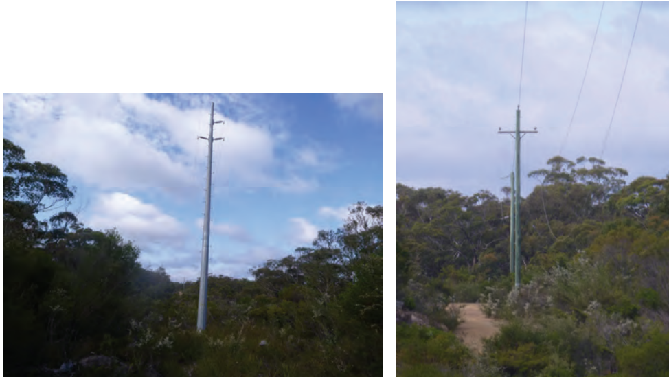
Fig. 6.4 33 kV powerline
