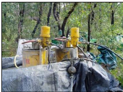
(a) Drilling into the bedrock
