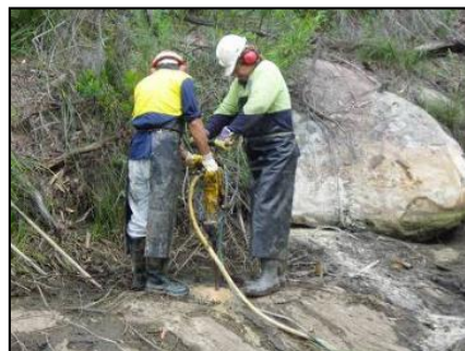
(b) Grout pump station setup
