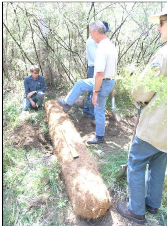
Figure 6-6 Round coir logs installed to spread water
