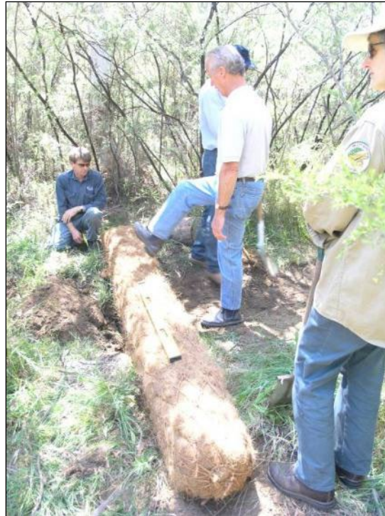
Figure 6-6 Round Coir Logs Installed to Spread Water
