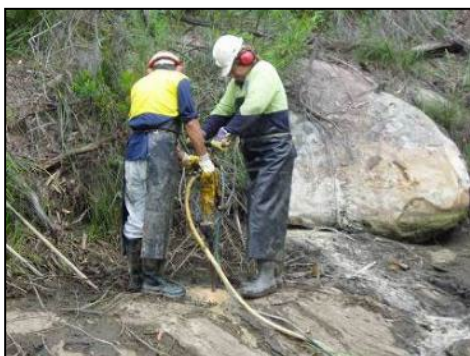
(a) Drilling into the bedrock
