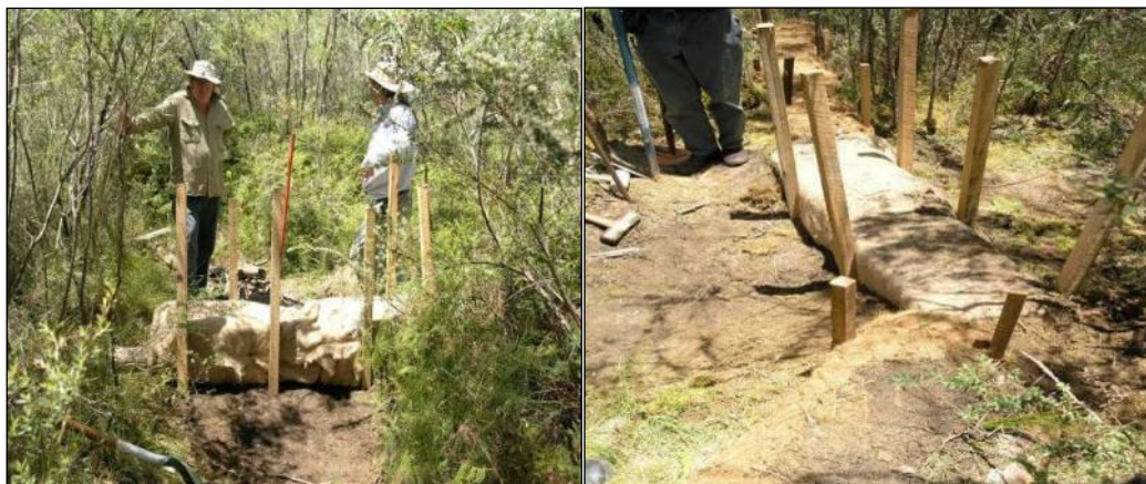
Figure 6-3 Installation of Square Coir Logs
