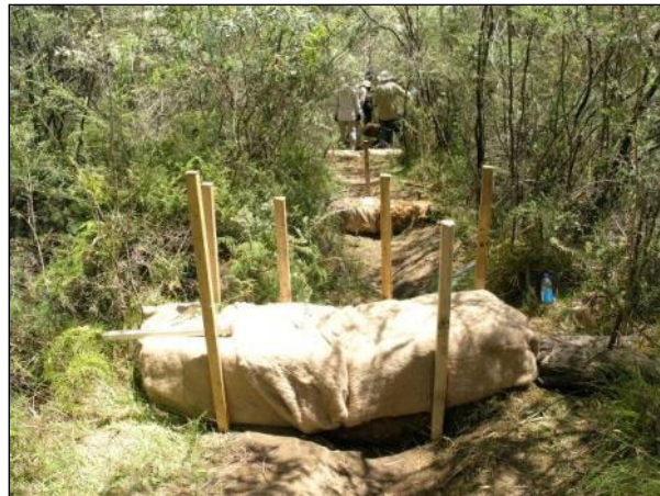
Figure 6-5 Small Coir Log Dams with Fibre Matting
