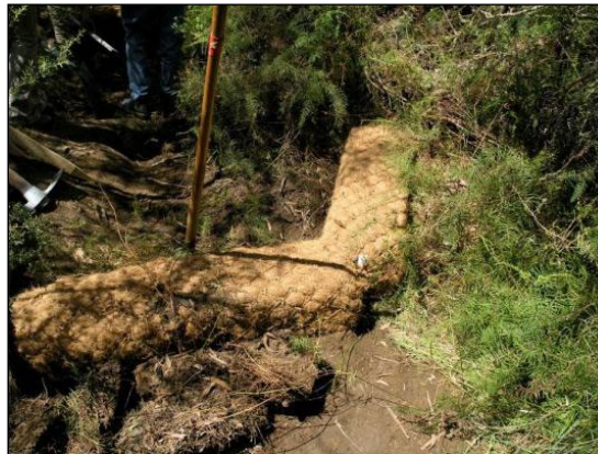
Figure 6-2 Square Coir Logs for Knick Point Control
