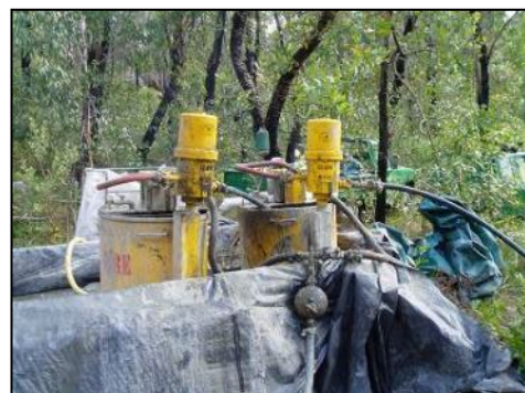
(b) Grout pump station setup
