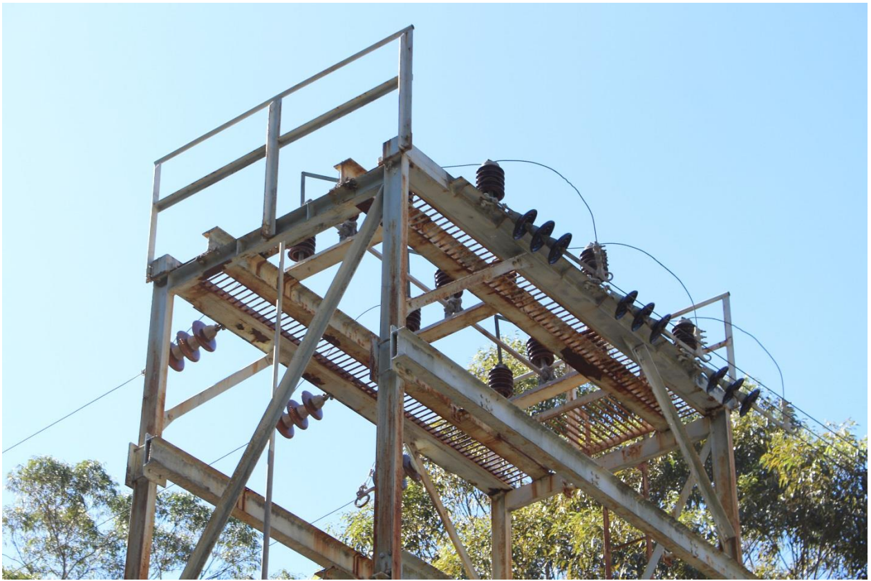
001 View of top of northern tower facing north west.
