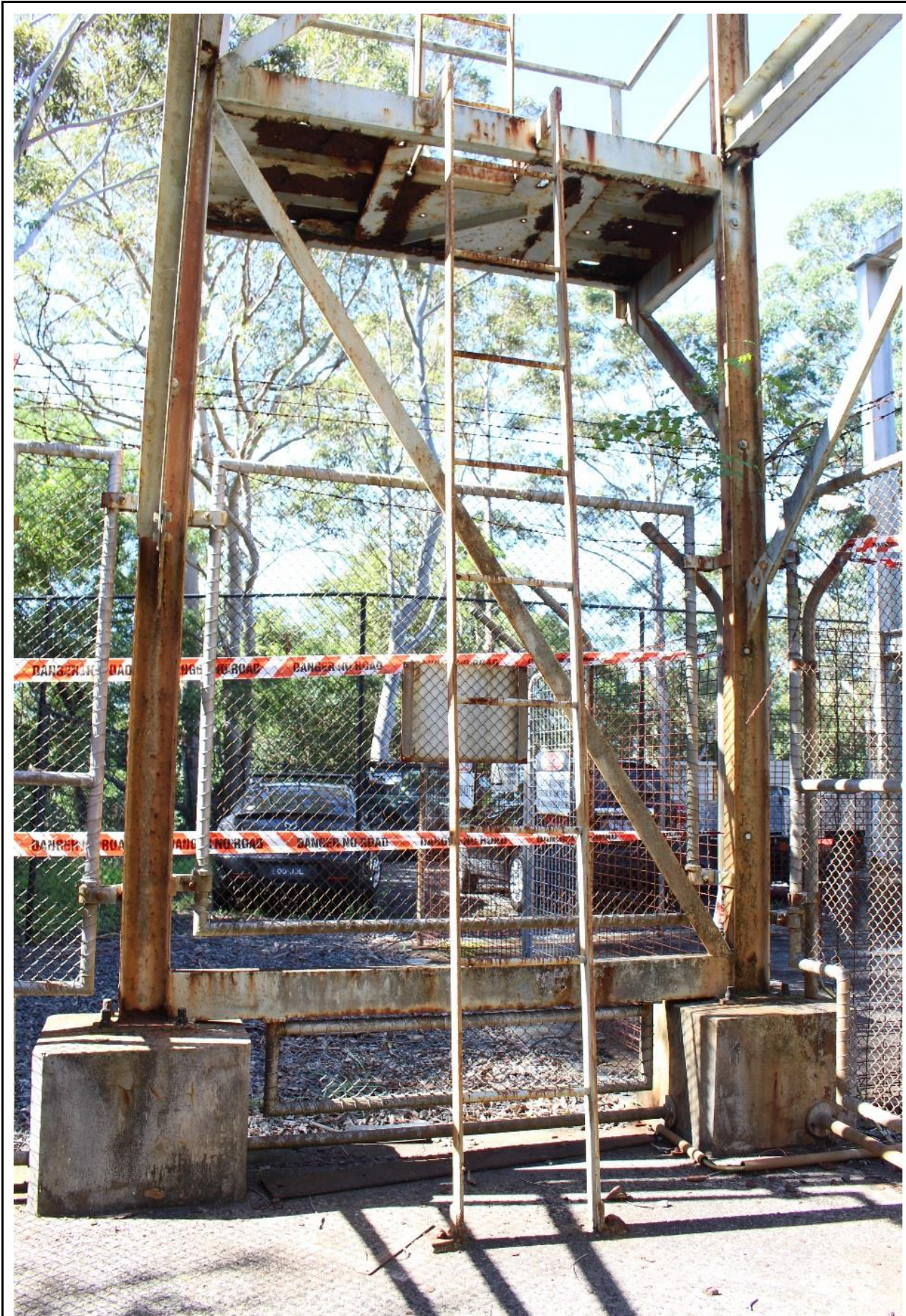
025 View inside of northern tower looking east
