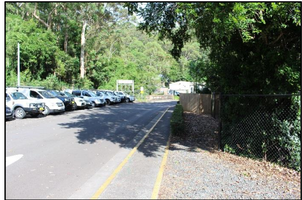
Plate 2: Eastern end of the substation view down access road to mine surface operations. East aspect. (Source: Niche 2018)
