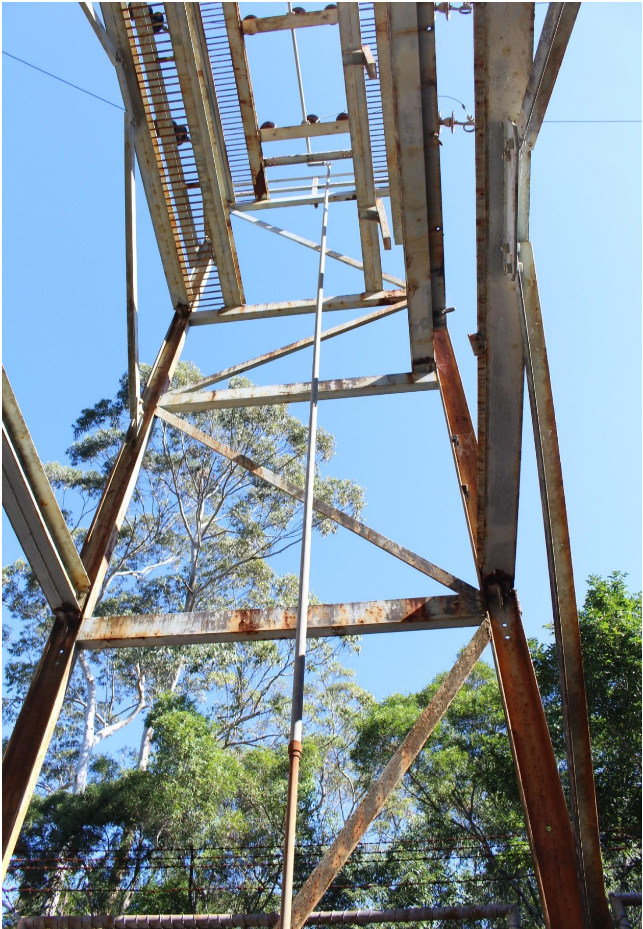
027 View inside of northern tower looking west
