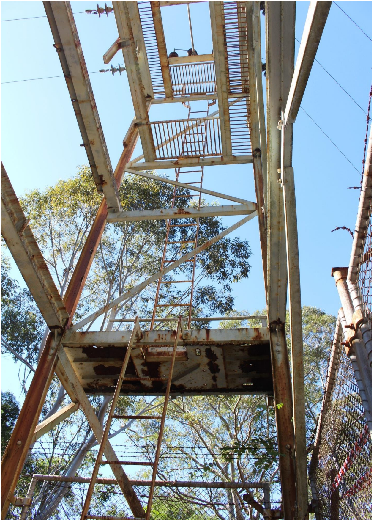
028 View inside of northern tower looking east
