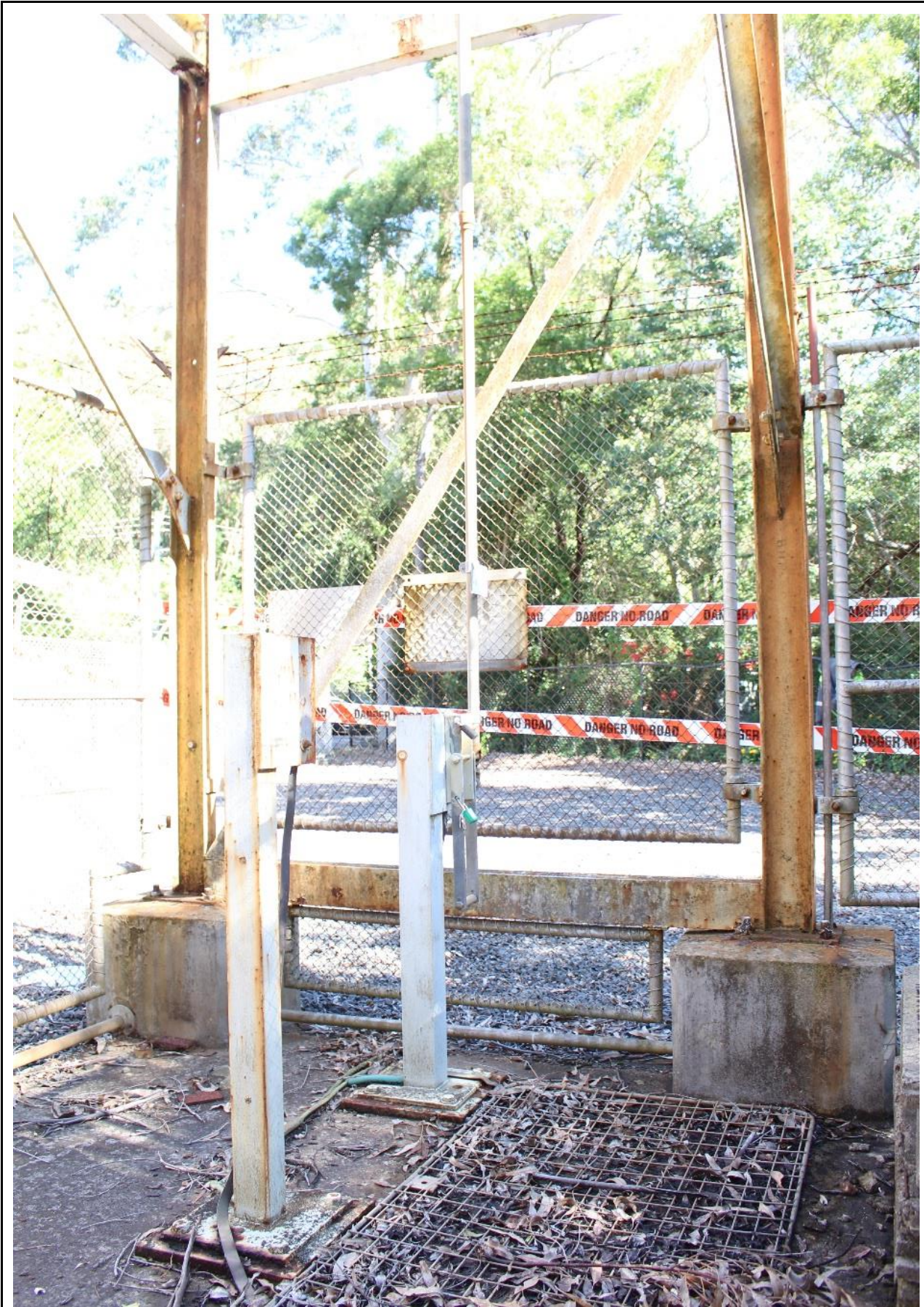
026 View inside of northern tower looking north
