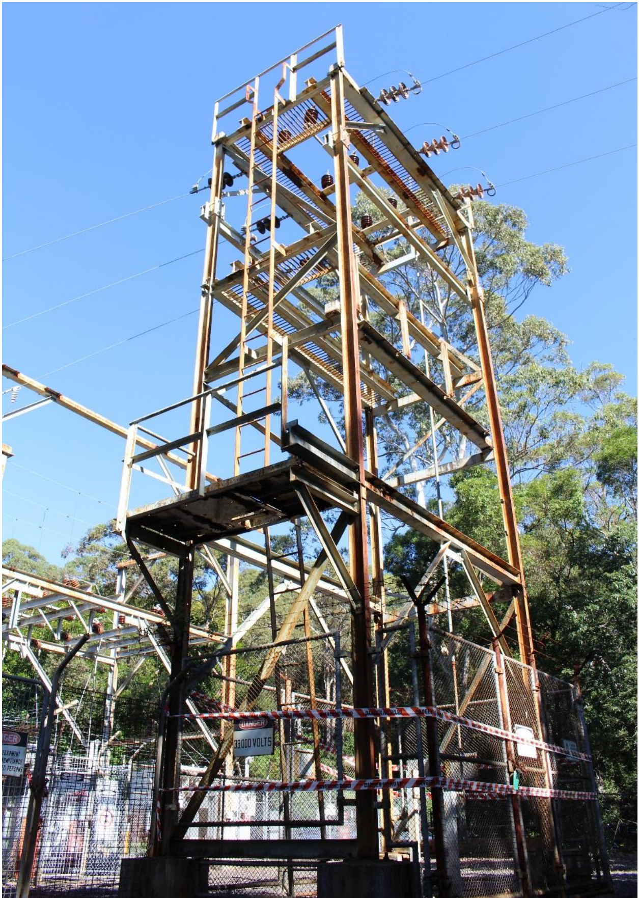
016 View of northern tower of 33kV Substation looking south west
