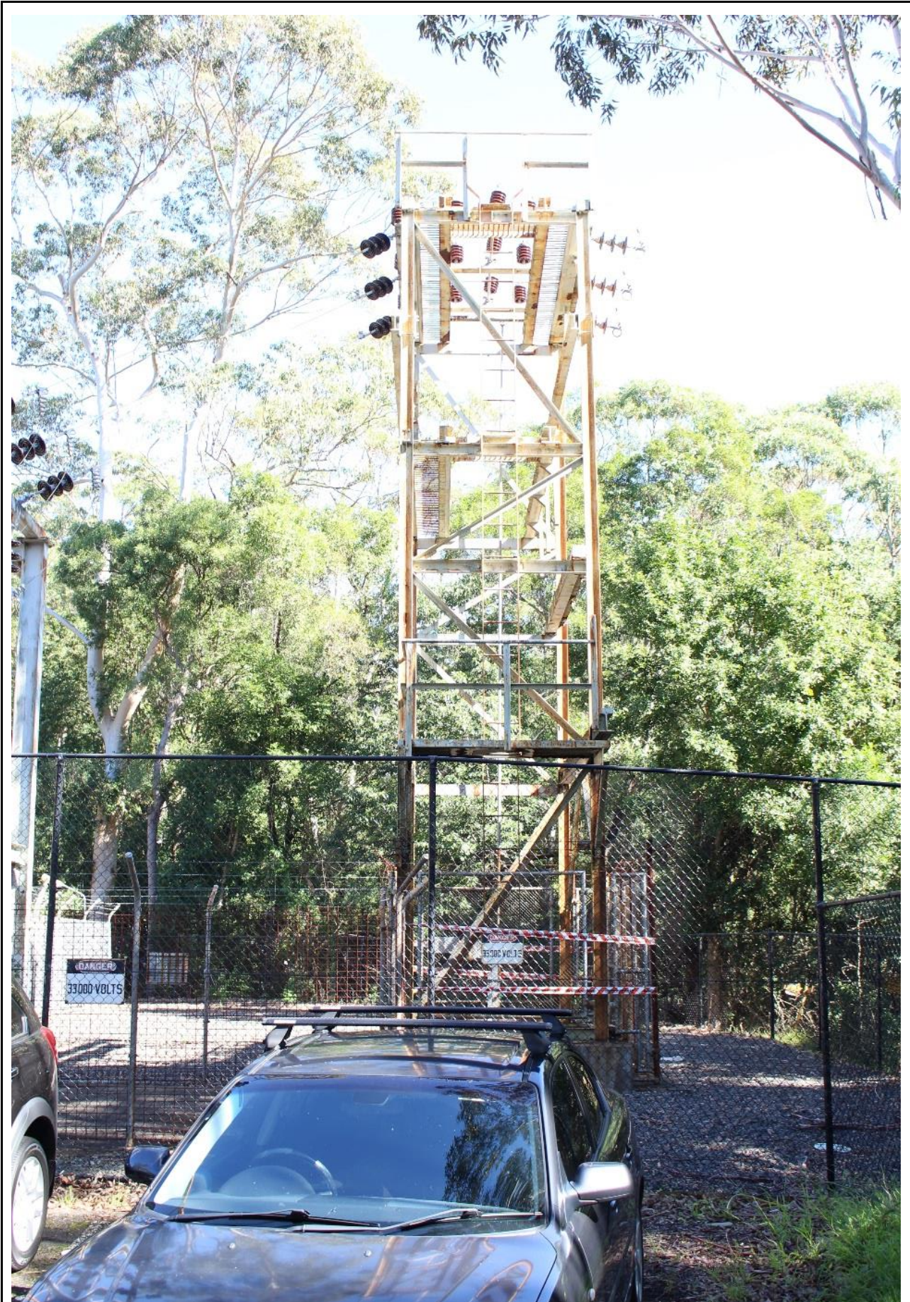
006 View of the northern tower facing west
