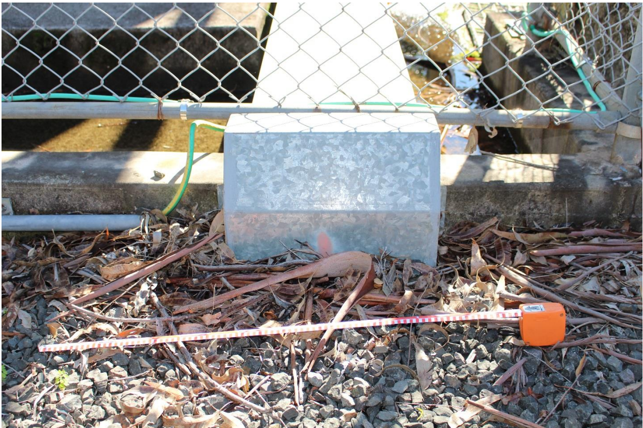
014 View of modern electrical addition to the substation looking west
