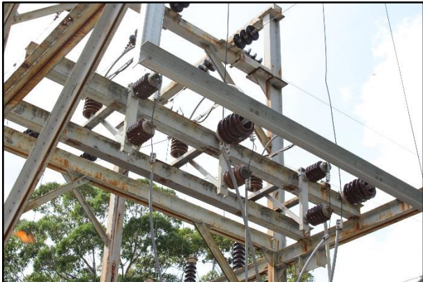
Plate 11: Example of orange brown ceramic transmission insulators, south east aspect (Source: Niche 2018)
