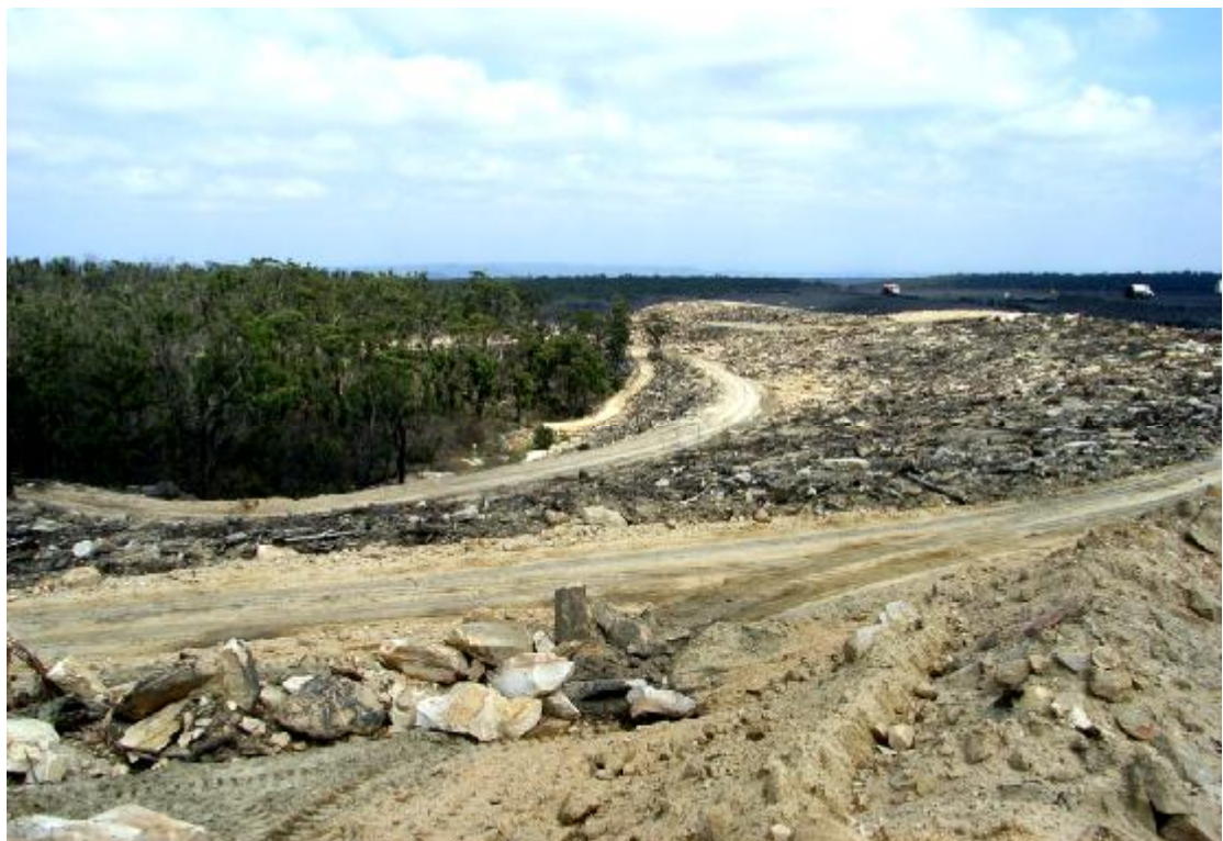
Figure 5 - Stage 2 Coal Wash Emplacement (Topsoiling at Front, Coal Wash Emplacement Occurring in Distance)
