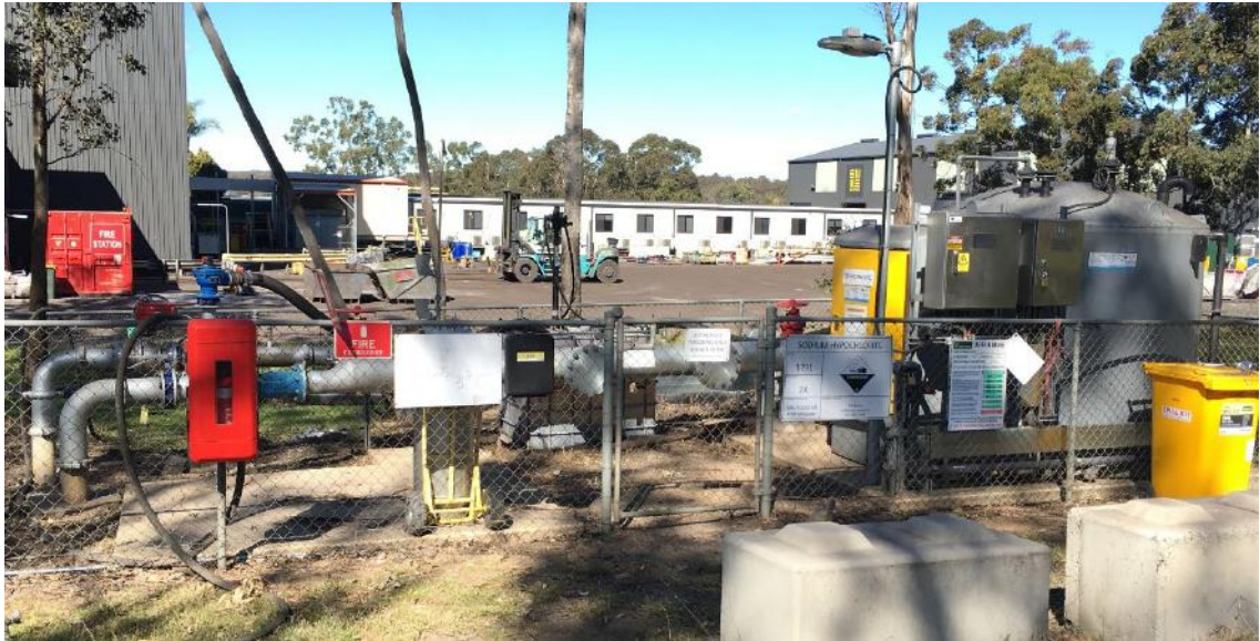
Plate 2: Recirculation Line Dosing System
