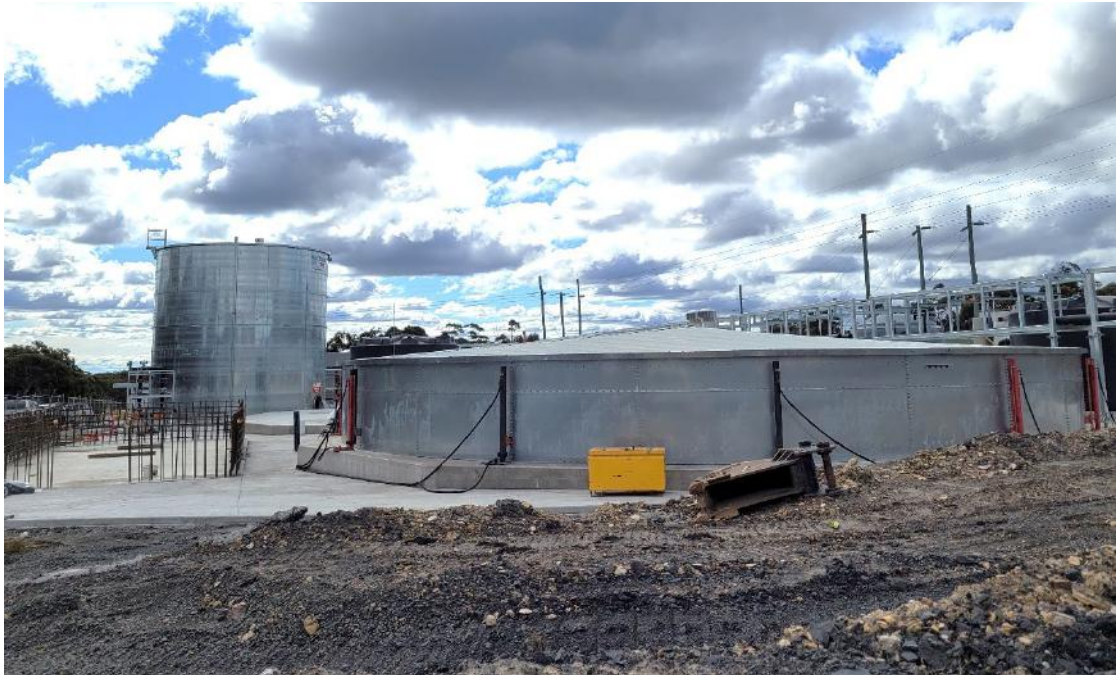
Plate 5: Appin North WTP construction as at August 2021
