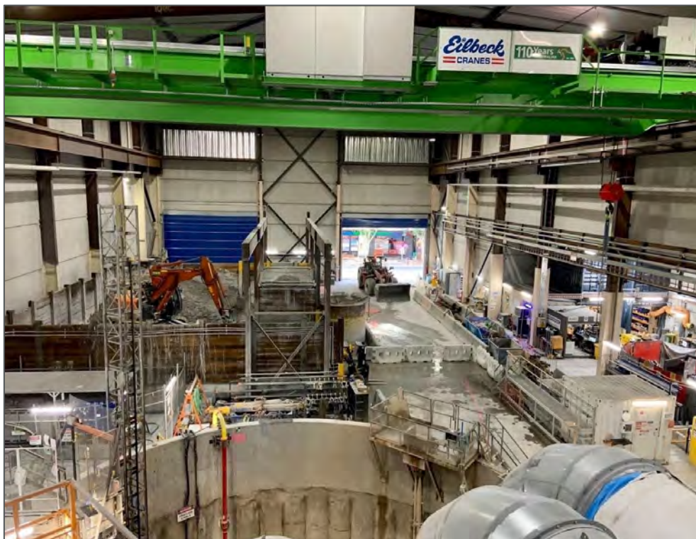
Figure 3-12 Acoustic shed example (internal view)
