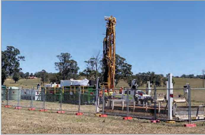
Typical geotechnical drill rig setup
