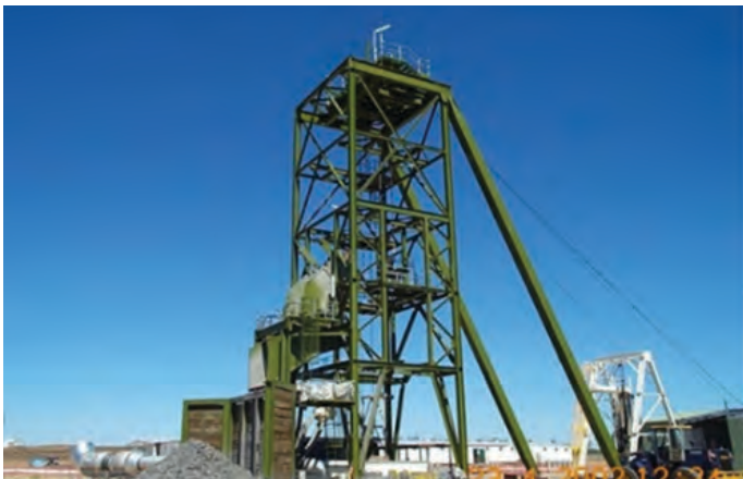
Example of a temporary headframe used in the Conventional Shaft Sinking method.
