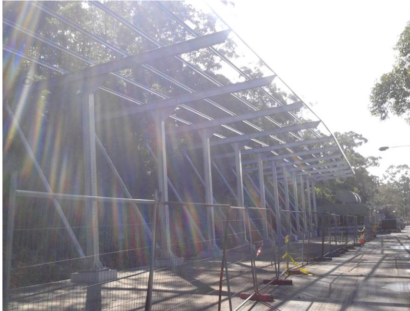
Figure 1: Bulk Storage Cover under Construction in August 2014.
