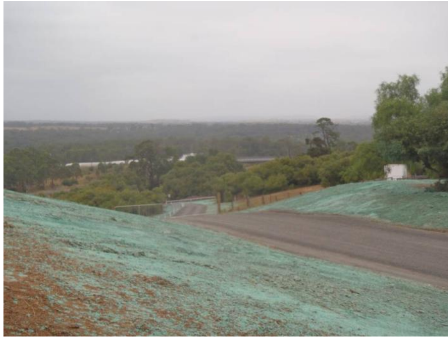
Figure 4.1. Progressive rehabilitation will include the battering down of constructed road verges and re-vegetating to promote soil stability as was done previously for the Longwall 704 Surface Gas Management Project.
