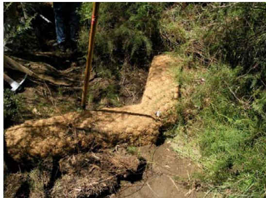
Plate 6-1 - Square Coir Logs for Knick Point Control
