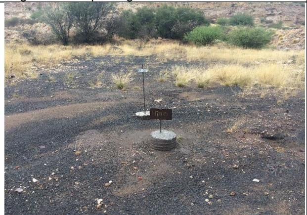
Figure 6: Prospecting Test Boreholes (sealed)
