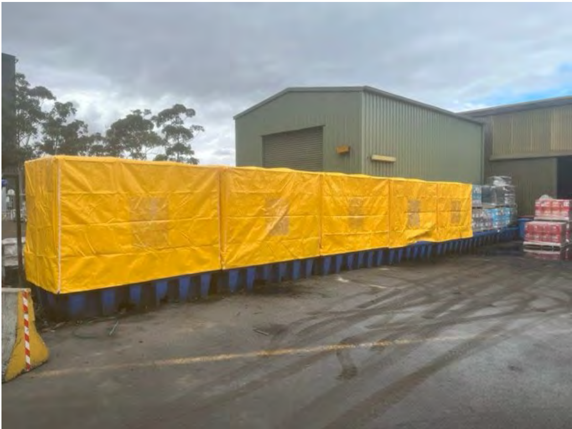
Plate 1: Weatherproof covers on storage bunds
