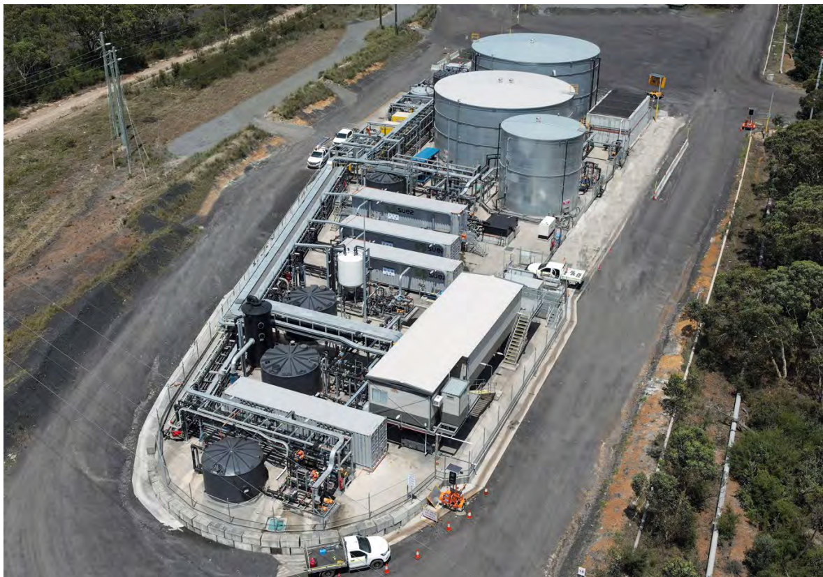
Plate 3: Appin North WTP
