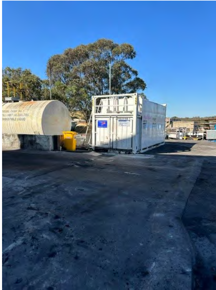
Plate 2: Upgrade of bulk solcenic refilling area with a concrete foundation
