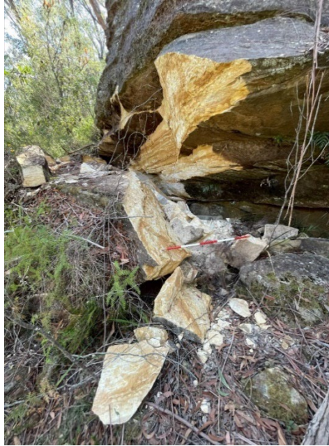
Photo 30: DA3C_LW21_027 , overview of rockfall. Taken 06/09/2023.
