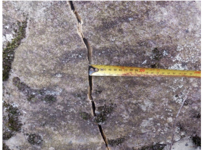
Photo 19: DA3C_LW21_012, maximum width of the rock fracture. Taken on 27/06/2023.
