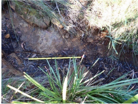
Photo 4: DA3C_LW21_015 , section of rock fracturing. Taken on 11/07/2023.
