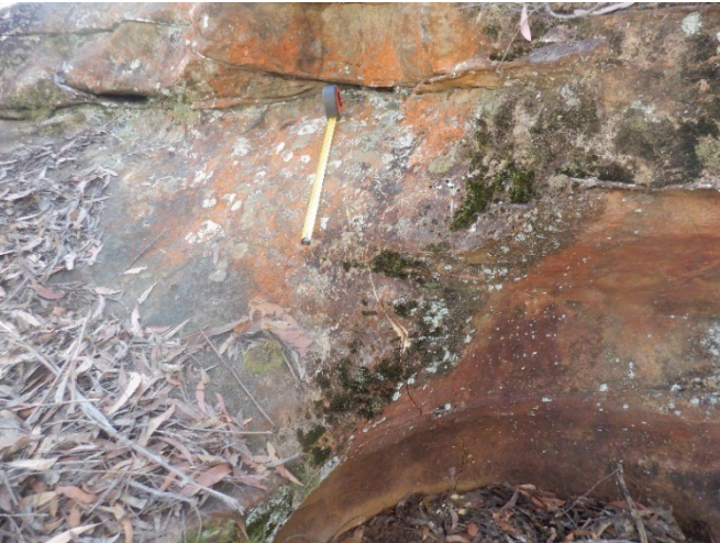
Photo 23: DA3C_LW21_018, section of rock fracturing. Taken on 26/07/2023.
