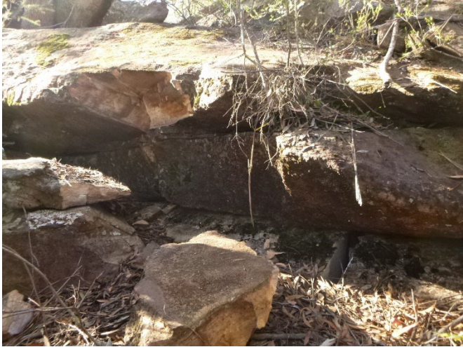
Photo 14: DA3C_LW21_007, fracturing and rock fall to outcrop. Taken on 15/06/2023.
