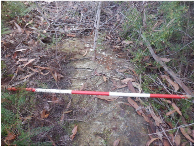
Photo 32: DA3C_LW21_029 , section of rock fracture. Taken 6/09/2023.
