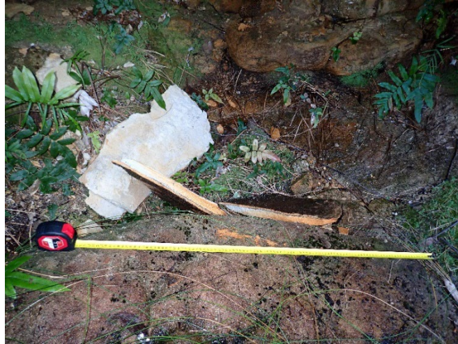
Photo 21: DA3C_LW21_016, fragments of rockfall from step. Taken on 11/07/2023.
