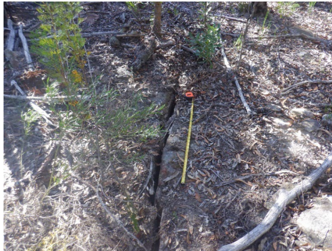
Photo 18: DA3C_LW21_011, section of rock fracturing. Taken on 19/06/2023.
