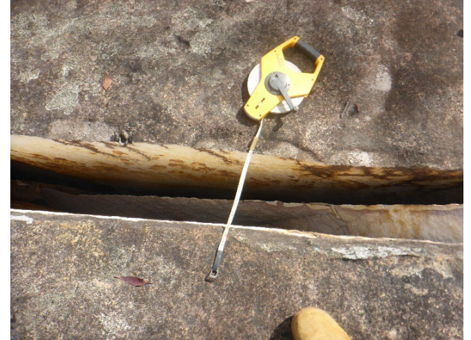
Photo 10: DA3C_LW21_003 , width of rock fracture. Taken on 06/06/2023.
