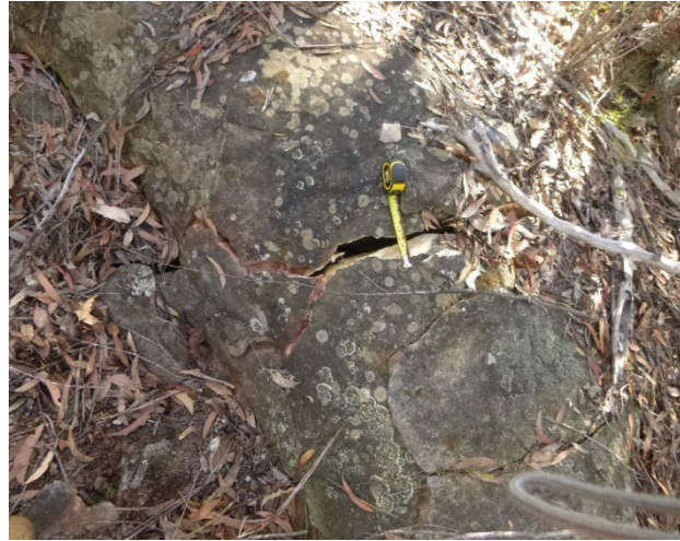
Photo 12: DA3C_LW21_005 , fracture to rock outcrop. Taken on 15/06/2023.
