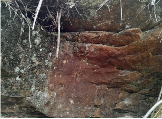
Photo 35: DA3C_LW21_032 , overview of fracturing to rock step/overhang. Taken 12/09/2023.
