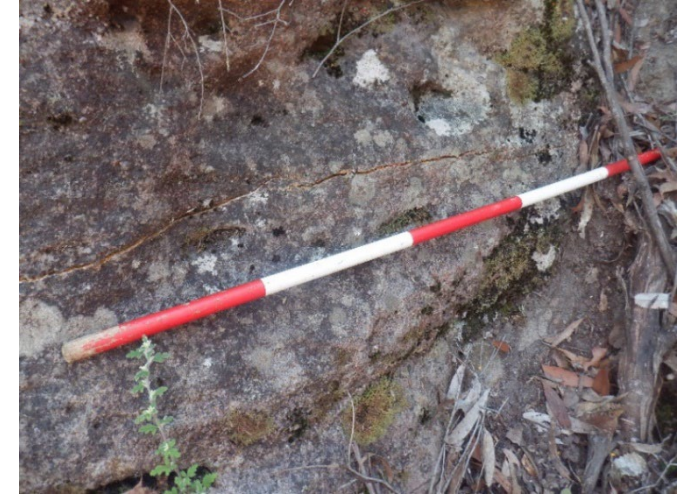
Photo 31: DA3C_LW21_028 , rock fracture. Taken 06/09/2023.
