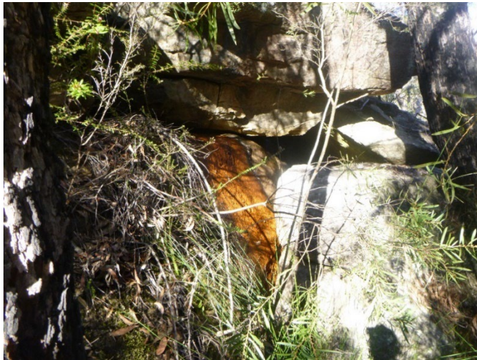
Photo 6: DA3C_LW21_021 , overview of the iron staining. Taken on 1/08/2023.
