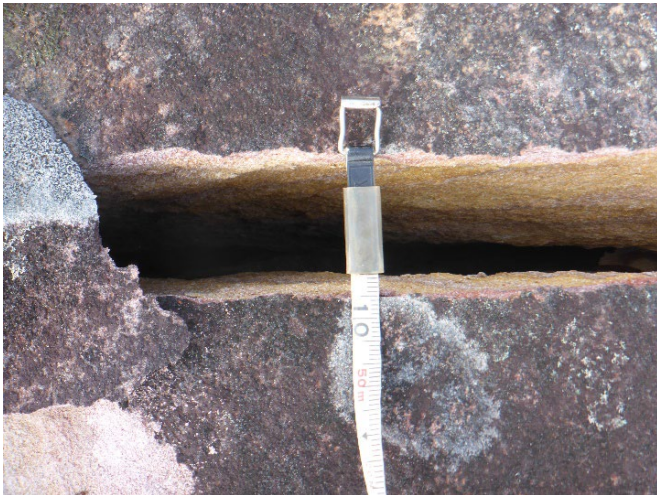
Photo 11: DA3C_LW21_004 , rock fracture width. Taken on 06/06/2023
