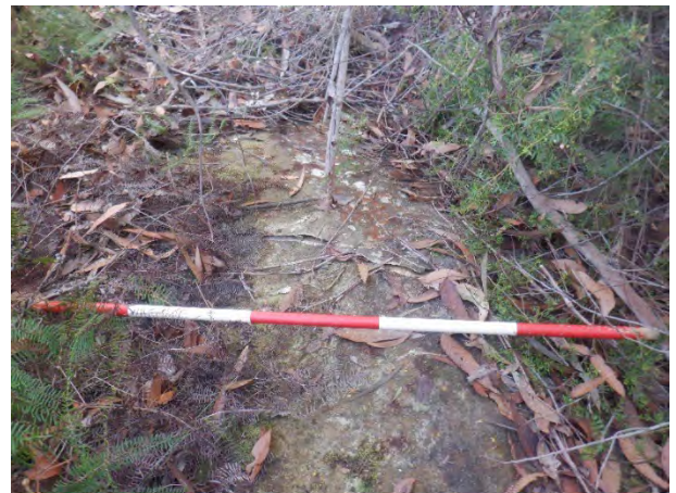
Photo 13: DA3C_LW21_029, section of rock fracture. Taken 6/09/2023
