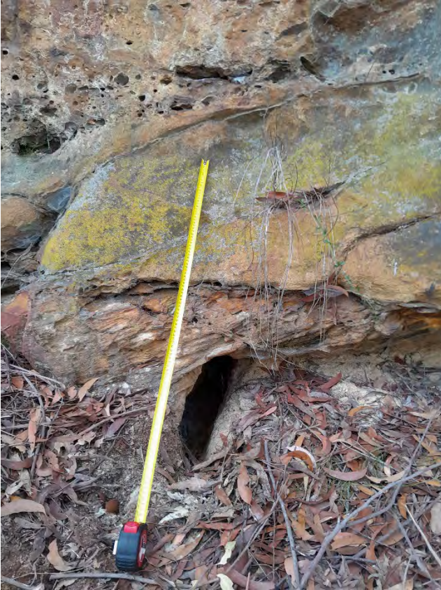
Photo 9: DA3C_LW21_034 overview of rock movement and soil crack. Taken: 12/09/2023.
