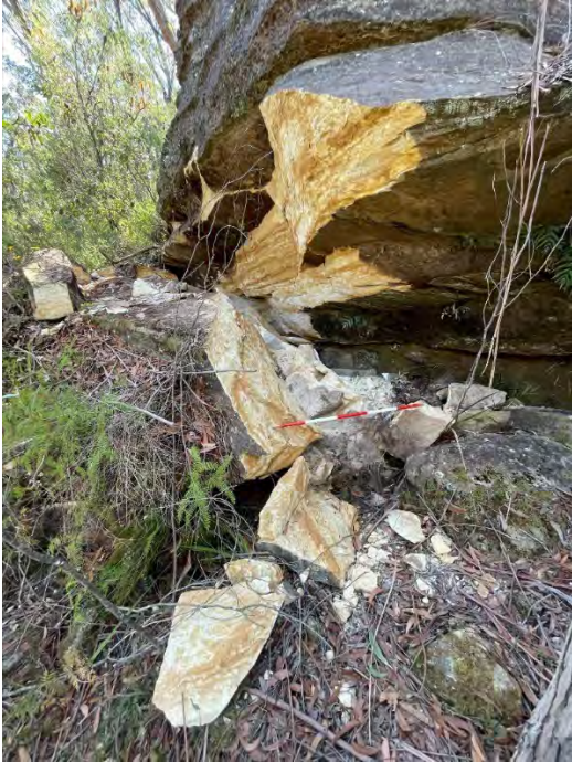
Photo 8: DA3C_LW21_027, overview of rockfall. Taken 06/09/2023
