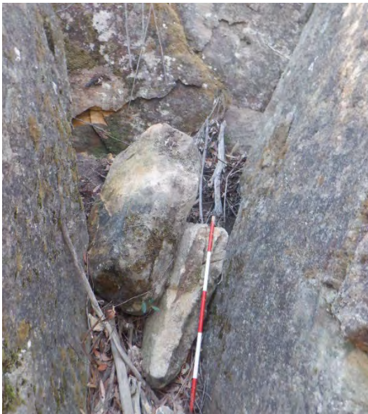
Photo 6: DA3C_LW21_026, section of rock fracture and rockfall. Taken 06/09/2023
