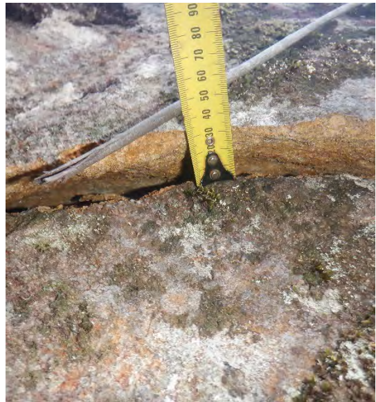
Photo 7: DA3C_LW21_026, Width of rock fracture. Taken 06/09/2023
