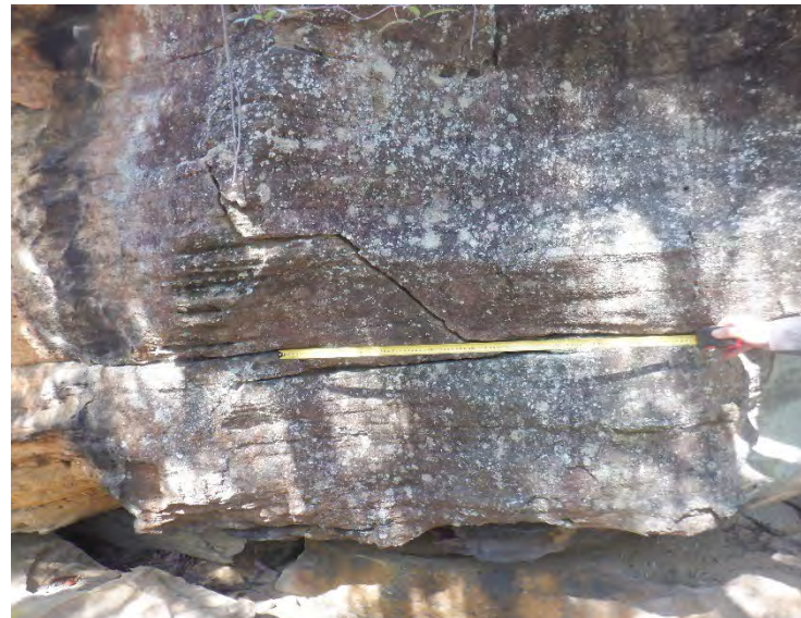
Photo 2: DA3C_LW21_019, looking at the rock fracture. Taken on 1/08/2023.
