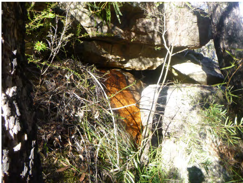
Photo 8: DA3C_LW21_021 , overview of the iron staining. Taken on 1/08/2023.
