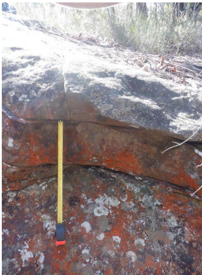
Photo 7: DA3C_LW21_018, overview of rock fracturing. Taken on 26/07/2023.
