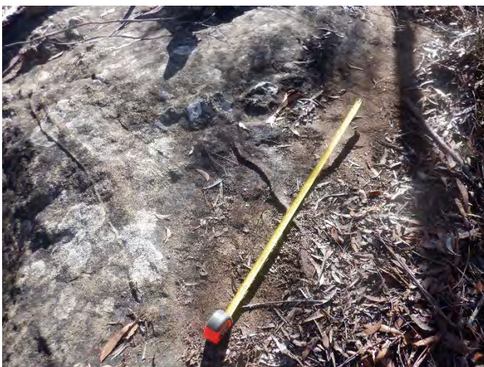
Photo 9: DA3C_LW21_018, section of rock fracturing. Taken on 26/07/2023.
