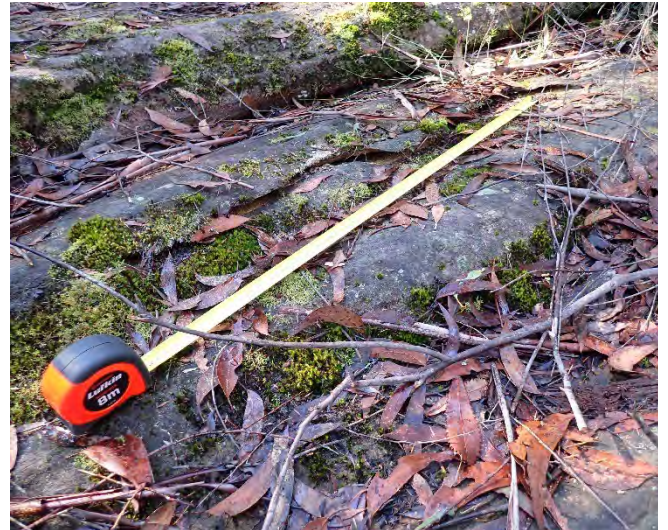
Photo 4: DA3C_LW21_017 , section of rock fracturing. Taken on 26/07/2023.
