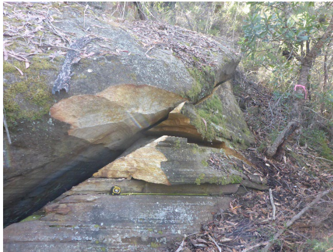
Photo 53: DA3A_LW19_060, showing rock fracturing and rockfall. Taken on 05/05/2023.
