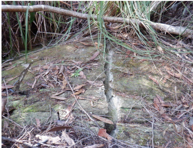
Photo 6: DA3A_LW19_051, showing rock fracturing on WC14. Taken on 04/05/2023.
