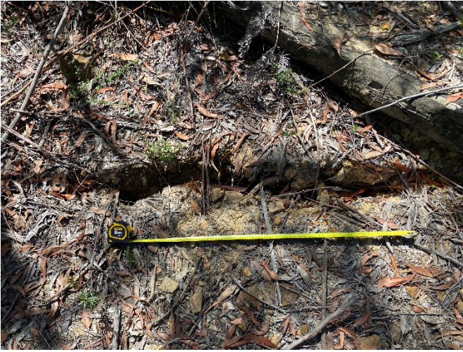
Photo 66: DA3A_LW19_035, showing soil cracking on a closed vehicle access track. Taken on 16/03/2023.
