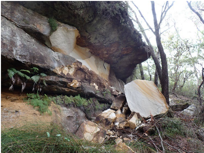
Photo 40: DA3A_LW19_041, showing rockfall at landscape monitoring site LW19_SS5. Taken on 12/04/2023.
