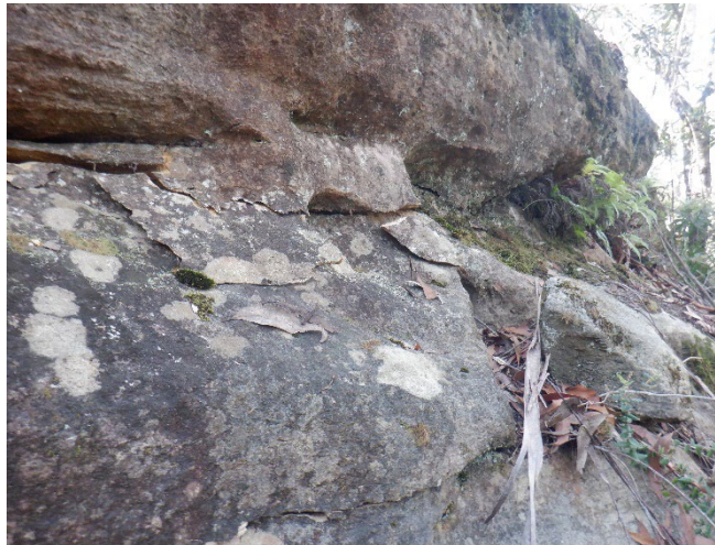
Photo 47: DA3A_LW19_054, showing rock fracturing and fragmentation. Taken on 04/05/2023.
