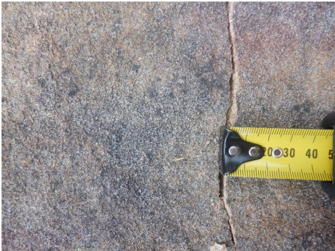
Photo 16: DA3A_LW19_011, showing rock fracturing. Taken on 7/11/2022.
