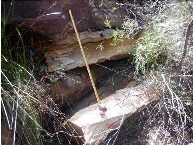
Photo 31: DA3A_LW19_027, showing rock fracturing and rockfall. Taken on 10/01/2023.
