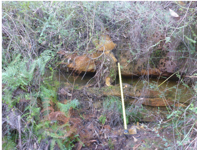
Photo 50: DA3A_LW19_057, showing rockfall. Taken on 05/05/2023.
