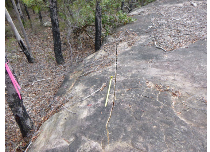
Photo 33: DA3A_LW19_030, showing rock fracturing. Taken on 15/02/2023.
