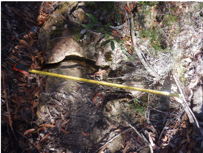
Photo 28: DA3A_LW19_023, showing rock fracturing. Taken on 09/05/2023.
