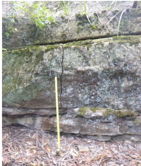
Photo 35: DA3A_LW19_032, showing rock Fracturing. Taken on 15/02/2023.
