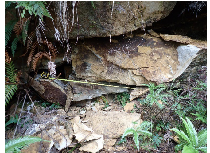
Photo 39: DA3A_LW19_040, showing rock fall and fragmentation. Taken on 12/04/2023.
