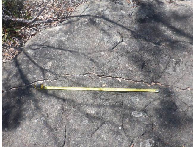
Photo 32: DA3A_LW19_028, showing rock fracturing. Taken on 06/02/2023.
