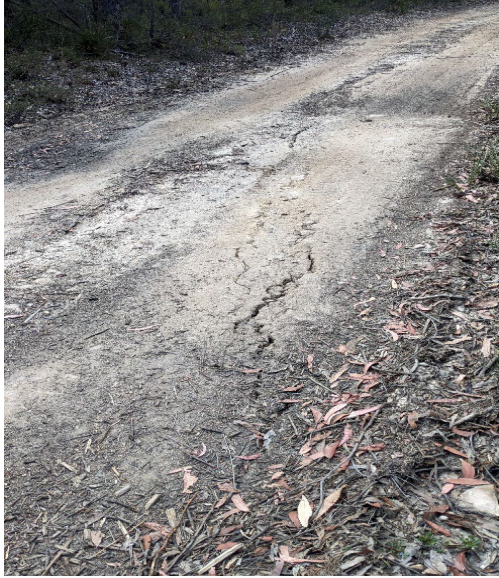
Photo 62: DA3A_LW19_026, showing soil cracking on Fire Road 6F. Taken on 16/06/2022
