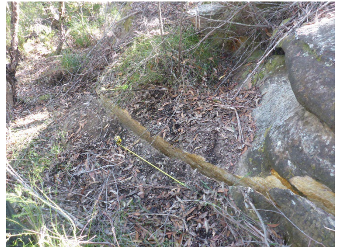
Photo 54: DA3A_LW19_061, showing rock fracturing. Taken on 05/05/2023.
