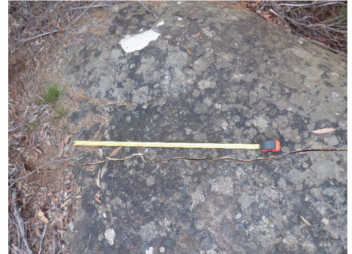
Photo 15: DA3A_LW19_010, showing rock fracturing. Taken on 7/11/2022.
