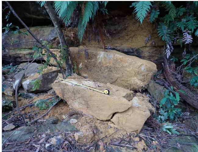
Photo 38: DA3A_LW19_039, showing rockfall. Taken on 12/04/2023.
