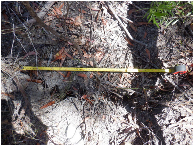
Photo 25: DA3A_LW19_020, showing soil cracking. Taken on 13/12/2022.
