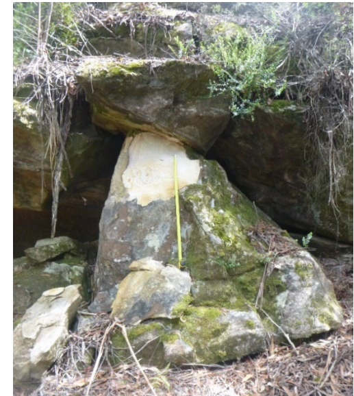
Photo 36: DA3A_LW19_033, showing rock fracturing. Taken on 15/02/2023.
