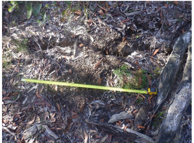
Photo 65: DA3A_LW19_049, showing soil cracking on a closed vehicle access track. Taken on 27/04/2023.
