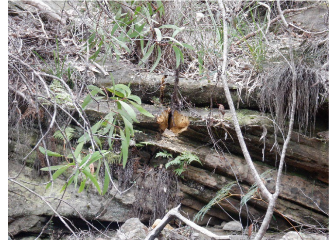
Photo 9: DA3A_LW19_004, showing rock fracturing and fragmentation. Taken on 19/08/2022.
