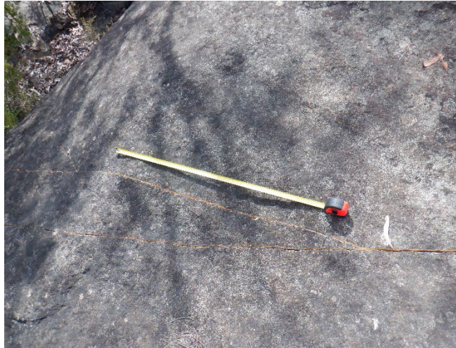
Photo 14: DA3A_LW19_009, showing rock fracturing. Taken on 7/11/2022.
