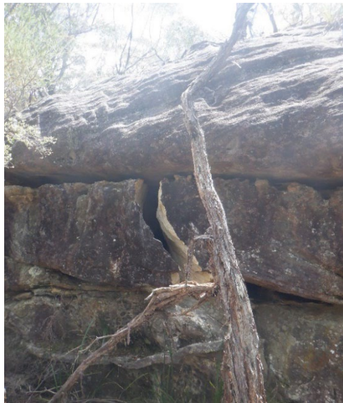
Photo 20: DA3A_LW19_015, showing rock fracturing. Taken on 7/11/2022.
