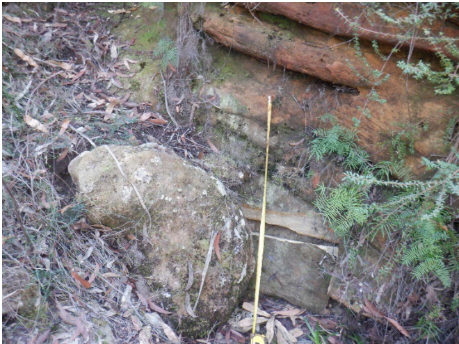
Photo 46: DA3A_LW19_053, showing rock fracturing and rockfall. Taken on 04/05/2023.
