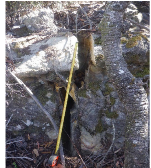
Photo 27: DA3A_LW19_022, showing rock fracturing. Taken on 09/05/2023.
