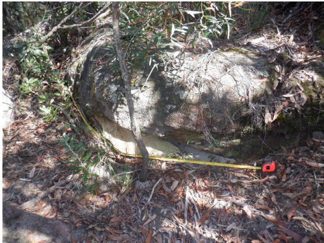
Photo 10: DA3A_LW19_005, showing rockfall. Tape set at 2.7m. Taken on 19/04/2023.
