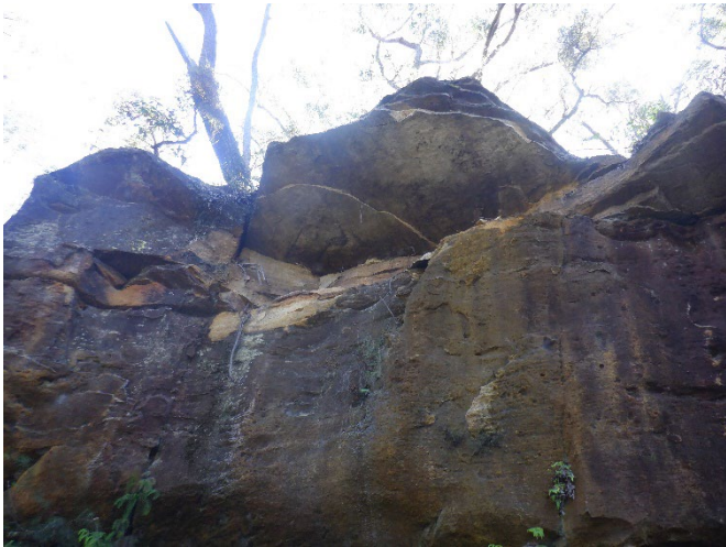
Photo 43: DA3A_LW19_046, showing rockfall. Taken on 27/04/2023.
