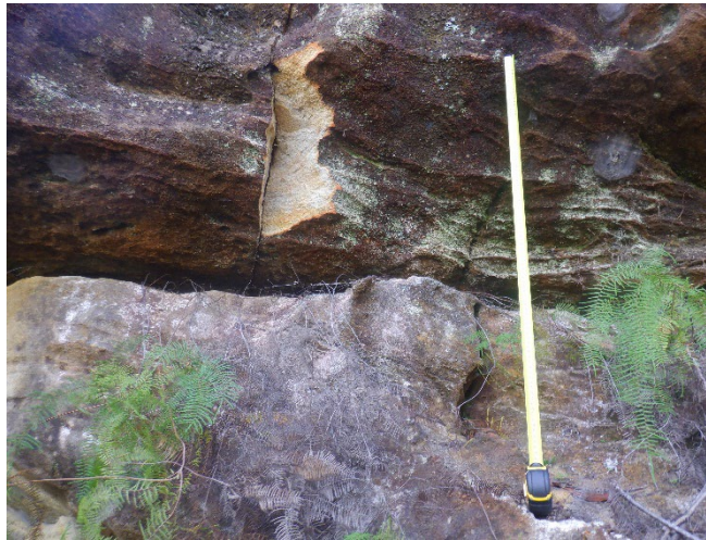
Photo 44: DA3A_LW19_047, showing rockfall. Taken on 27/04/2023.
