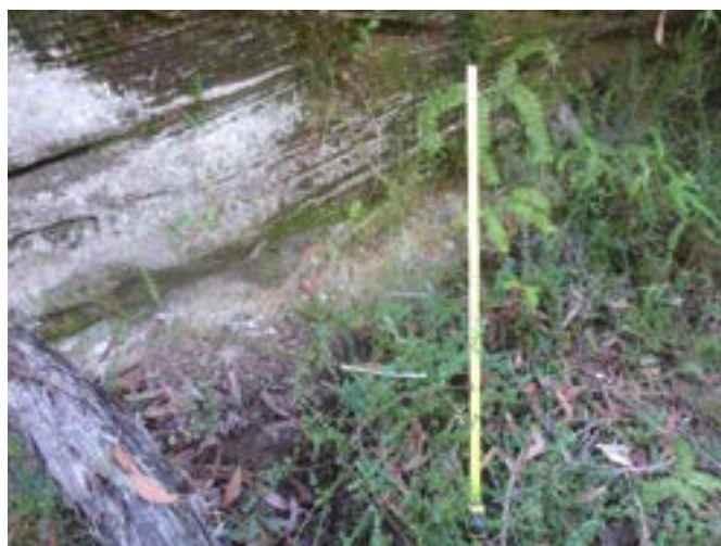
Photo 25: DA3A_LW19_061 , showing extent of rock fracture. Taken on 05/05/2023.
