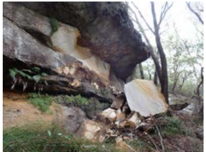
Photo 10: DA3A_LW19_041 looking at the rockfall at landscape site LW19_SS5. Taken 12/04/2023.
