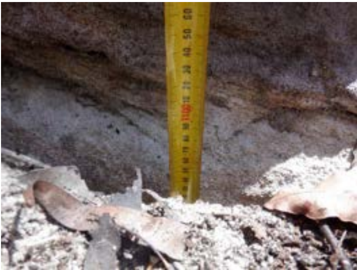
Photo 11: DA3A_LW19_021, depth of soil cracking. Taken on 13/12/2022.
