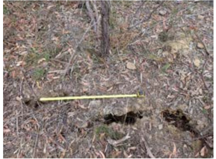
Photo 2: DA3A_LW19_024, section of soil cracking. Taken on 20/12/2022.
