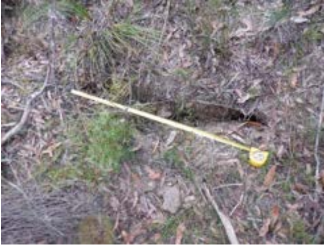
Photo 1: DA3A_LW19_007, section of soil cracking. Taken on 18/10/2022.
