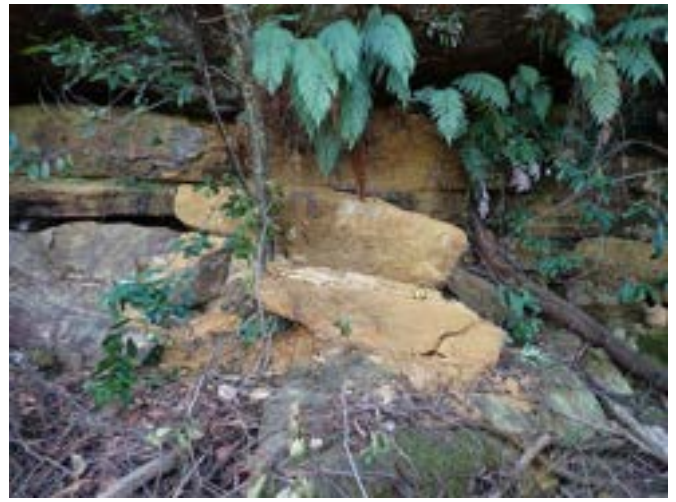
Photo 6: DA3A_LW19_039 , looking at the rockfall. Taken 12/04/2023
