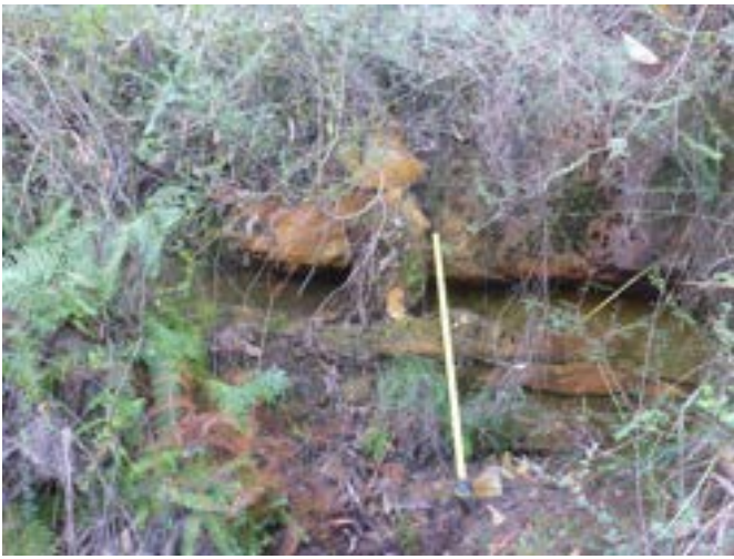
Photo 13: DA3A_LW19_057 , showing step where rocks detached. Taken on 5/05/2023.
