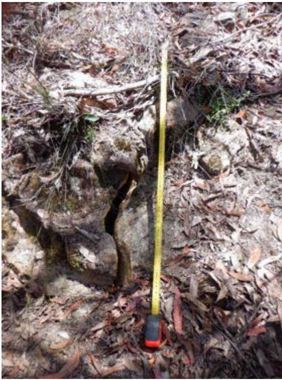
Photo 17: DA3A_LW19_023 , section of rock displacement. Taken on 13/12/2022.
