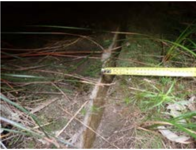
Photo 1: DA3A_LW8_003, looking at the width of rock fracturing. Taken 12/04/2023.
