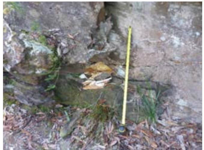
Photo 18: DA3A_LW19_059 , showing fallen debris. Taken on 5/05/2023.
