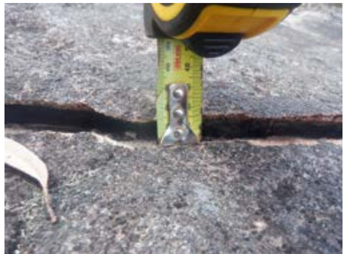
Photo 2: DA3A_LW19_028, width of rock fracturing. Taken on 6/02/2023.
