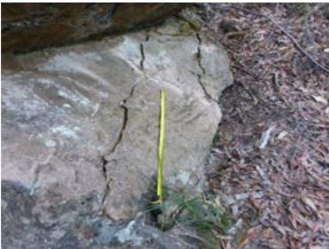
Photo 17: DA3A_LW19_059 , showing rock fracturing. Taken on 5/05/2023.
