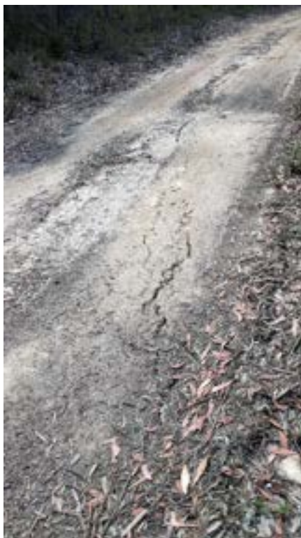
Photo 7: DA3A_LW19_026 , section of soil cracking. Taken on 21/12/2022.
