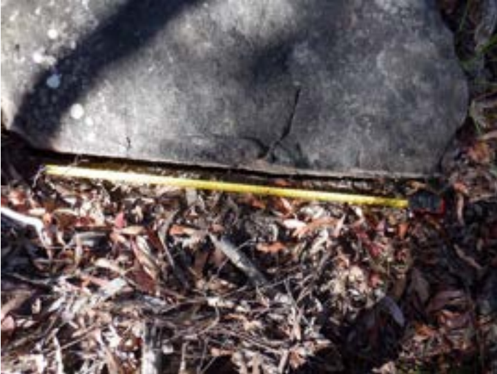
Photo 3: DA3A_LW19_018 , section of rock displacement. Taken on 13/12/2022.
