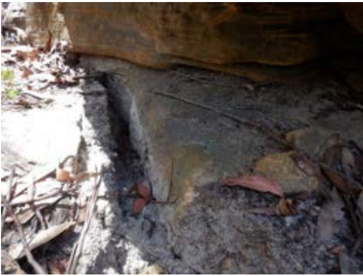
Photo 9: DA3A_LW19_021, section of soil cracking. Taken on 13/12/2022.
