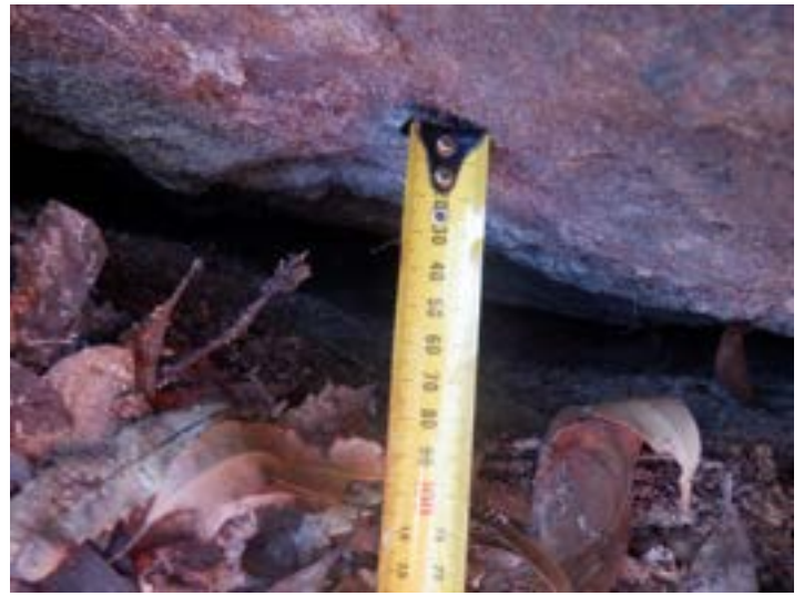
Photo 6: DA3A_LW19_019, width of rock displacement. Taken on 13/12/2022.
