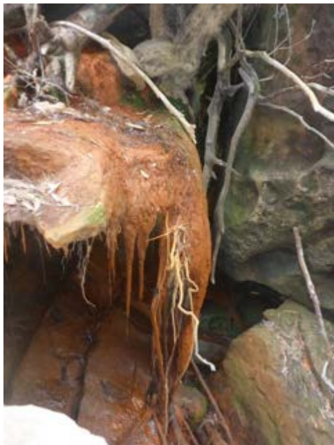
Photo 13: WC14_Step 3, looking at the iron staining. Taken on 28/01/2020.
