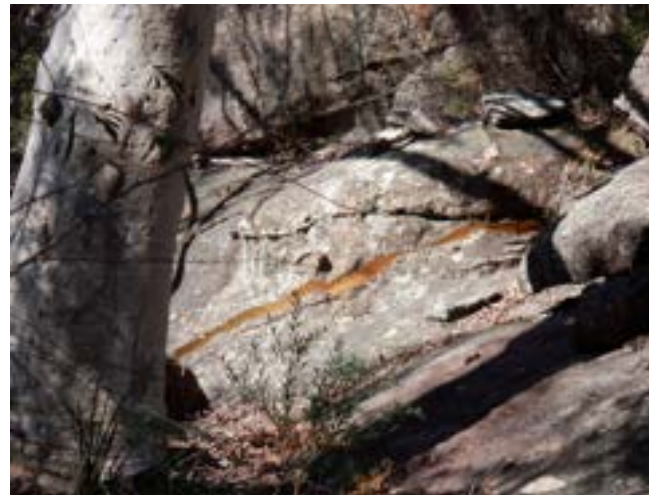
Photo 3: DA3A_LW19_002, showing a section of rock fracturing. Taken 3/08/2022.
