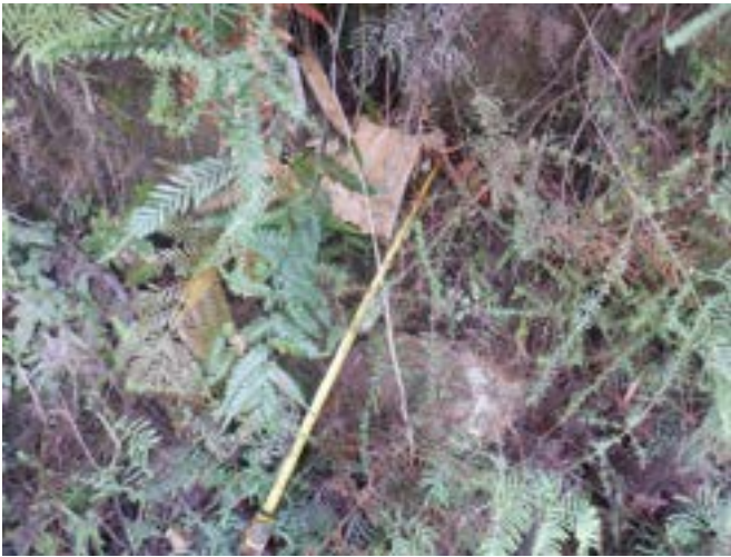
Photo 3: DA3A_LW19_052, showing area of rockfall. Taken on 4/5/2023.
