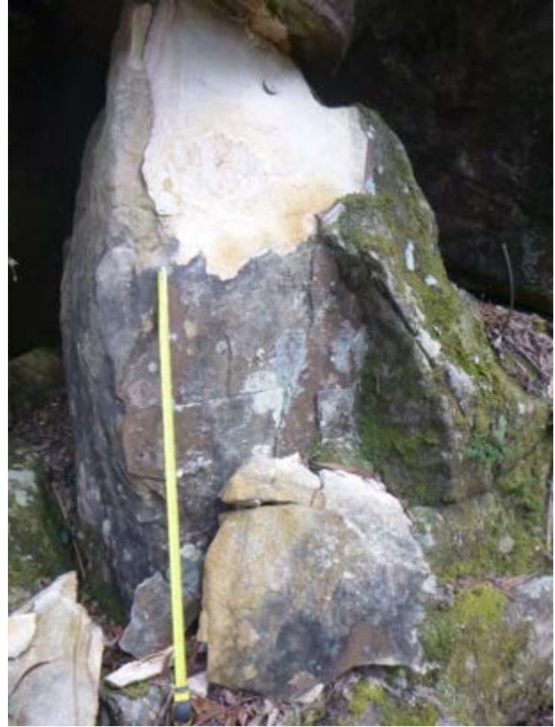
Photo 9: DA3A_LW19_033, rock fall from edge of steep slope. Taken on 15/2/2023.
