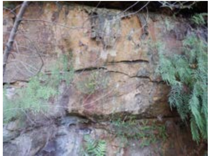
Photo 4: DA3A_LW19_052, showing area of rock fracturing. Taken on 4/5/2023.
