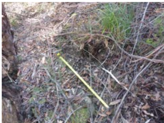
Photo 23: DA3A_LW19_061 , showing extent of soil crack. Taken on 05/05/2023.
