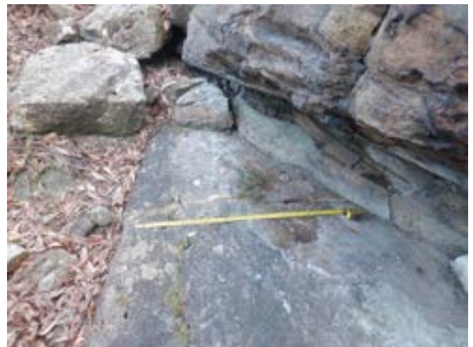
Photo 10: DA3A_LW19_055 , showing rock fracturing. Taken on 4/5/2023.
