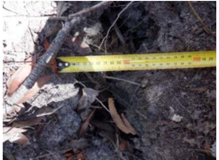
Photo 8: DA3A_LW19_020, width of soil cracking. Taken on 13/12/2022.
