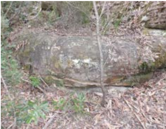
Photo 2: DA3A_LW19_005, looking at section of rock fracturing. Taken on 19/08/2022.
