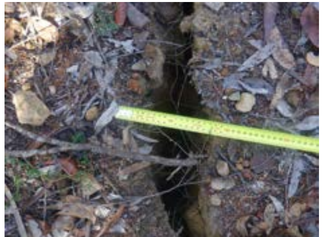
Photo 14: DA3A_LW19_050, showing width of soil crack. Taken on 27/04/2023.
