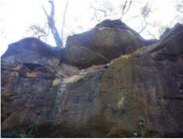
Photo 3: DA3A_LW19_046, showing steep slope/step face where rocks detached. Taken on 27/04/2023.
