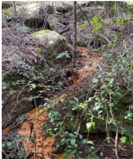
Photo 6: DA3A_LW19_044, looking at extent of iron staining. Taken 19/04/2023.
