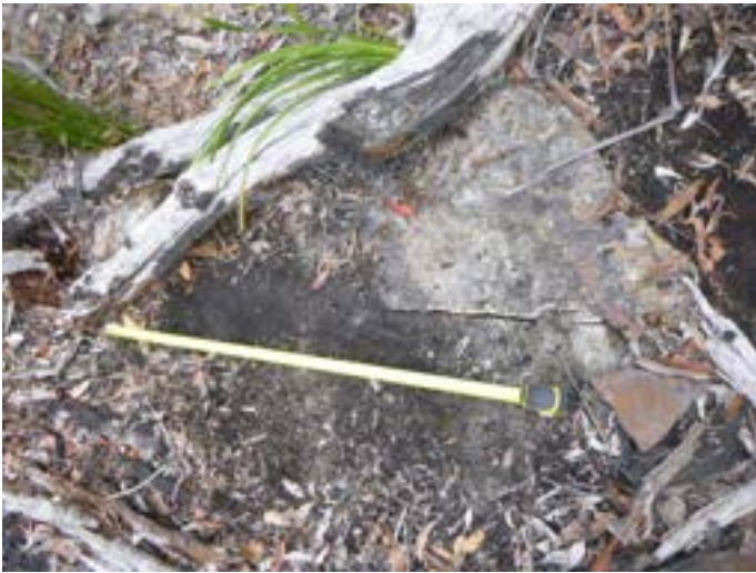
Photo 3: DA3A_LW19_031, rock fracturing to an outcrop. Taken on 15/2/2023
