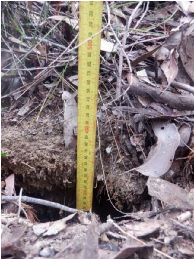
Photo 3: DA3A_LW19_007, depth of soil cracking. Taken on 18/10/2022.
