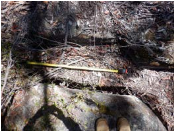
Photo 15: DA3A_LW19_022, section of rock displacement. Taken on 13/12/2022.
