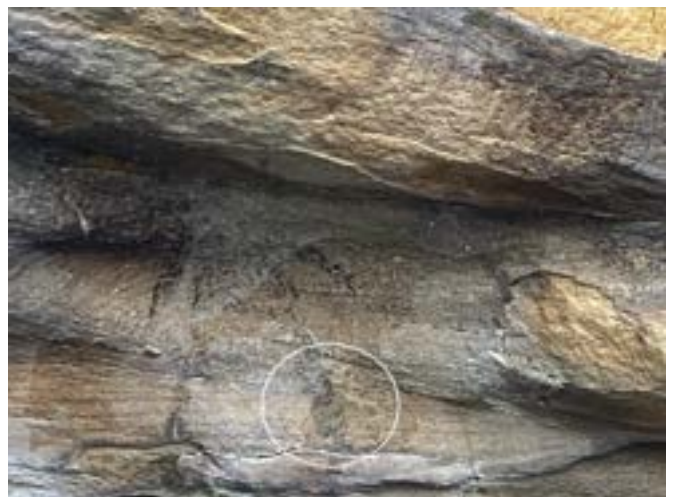
Photo 14: Art at DM15- image taken in latest inspection showing current fracturing. Recent fracture is circled. Taken on 28/03/2023.
