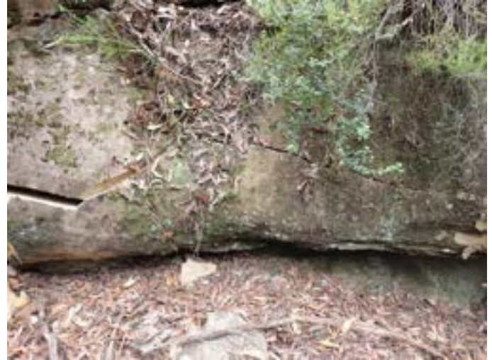
Photo 14: DA3A_LW19_016 , width of rock fracturing. Taken on 20/12/2022.
