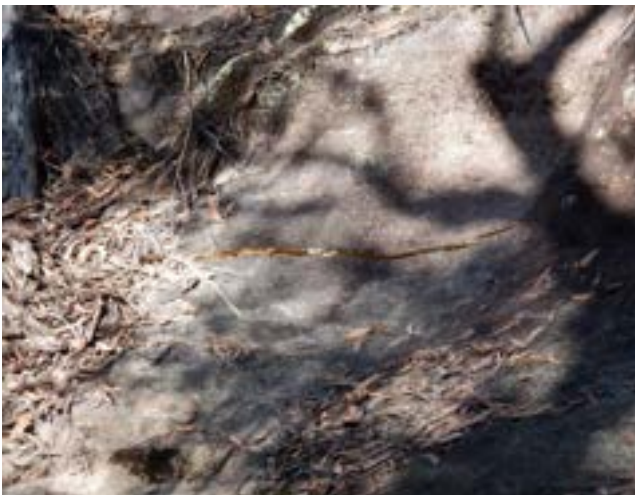
Photo 4: DA3A_LW19_002, showing a section of rock fracturing. Taken 3/08/2022.
