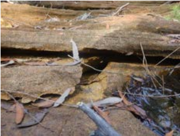
Photo 3: DA3A_LW19_043, looking at rock fracturing across rockbar. Taken 17/04/2023.
