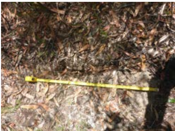
Photo 8: DA3A_LW19_025, showing soil cracking. Taken on 17/01/2023
