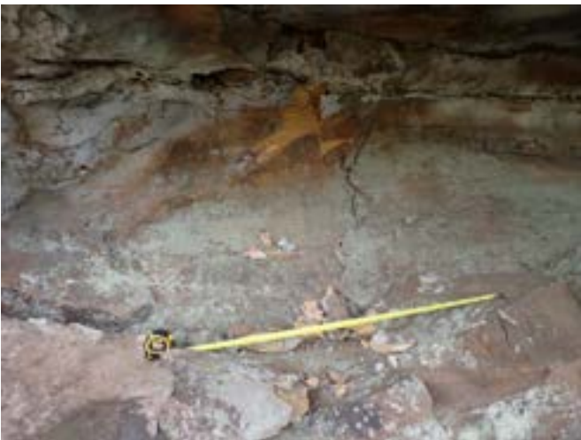
Photo 15: DA3A_LW19_042 looking at rockfall and associated fragments. Taken 12/04/2023.
