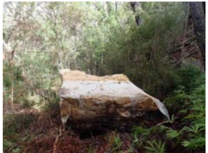
Photo 12: DA3A_LW19_041 looking at boulder that has dislodged and rolled downhill from steep slope.
