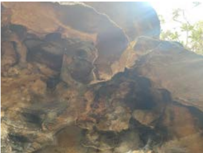
Photo 11: DA3A_LW19_038, section where rock fall occurred. Taken on 28/03/2023.
