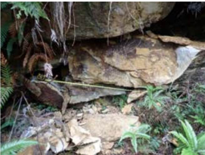
Photo 7: DA3A_LW19_040 , looking at rockfall and fragments. Taken 12/04/2023.
