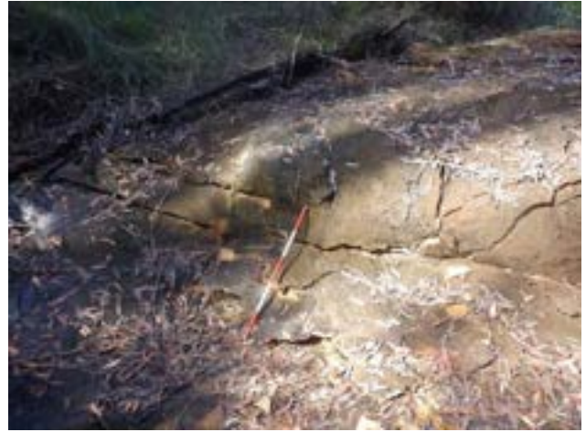
Photo 2: DA3A_LW19_043, looking upstream at rock fracturing on rockbar. Taken 17/04/2023.
