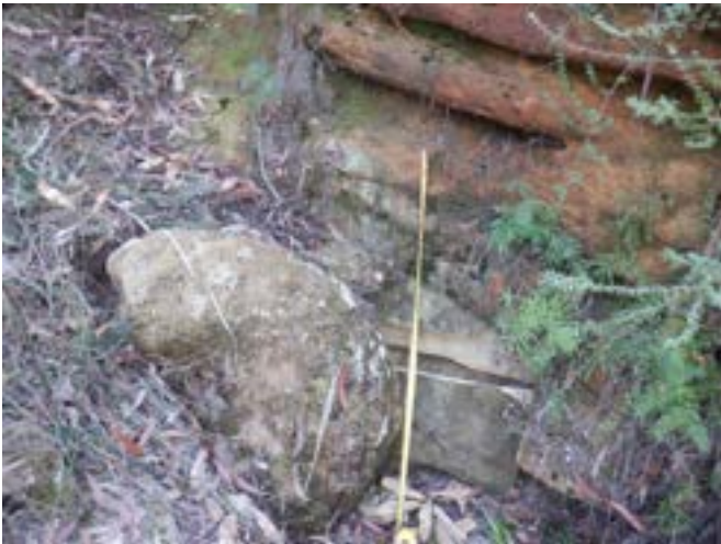
Photo 5: DA3A_LW19_053 , showing area of rockfall. Taken on 4/5/2023.
