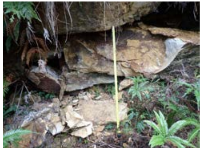
Photo 8: DA3A_LW19_040 , looking at rockfall and fragments. Taken 12/04/2023.
