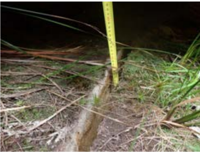
Photo 3: DA3A_LW8_003, looking at the depth of rock fracturing. Taken 12/04/2023.
