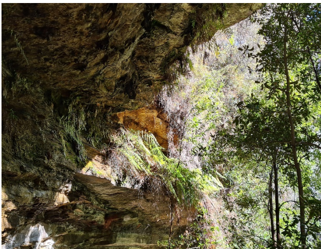
Photo 1: DA3B_LW17_041 , showing site of rock fall. Taken 2/08/2022.
