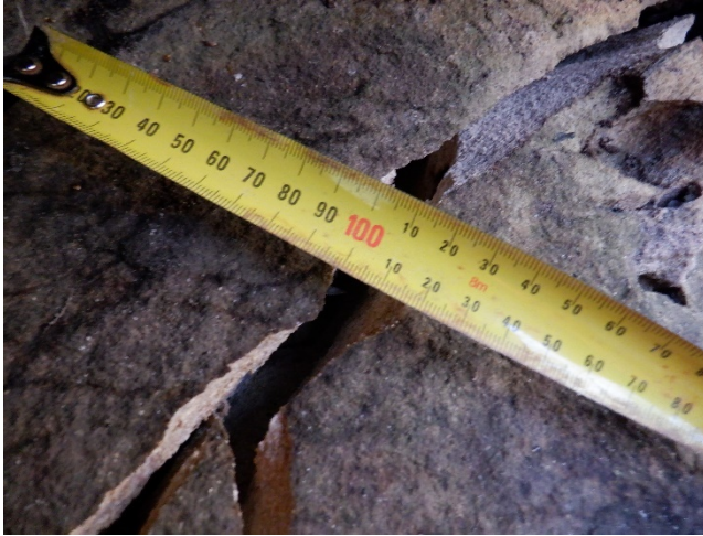
Photo 7: DA3B_LW18_009 , showing width of rock fracturing. Taken 9/06/2022.
