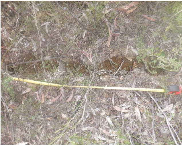
Photo 27: DA3B_LW18_023, showing section of soil cracking. Taken 16/08/2022.
