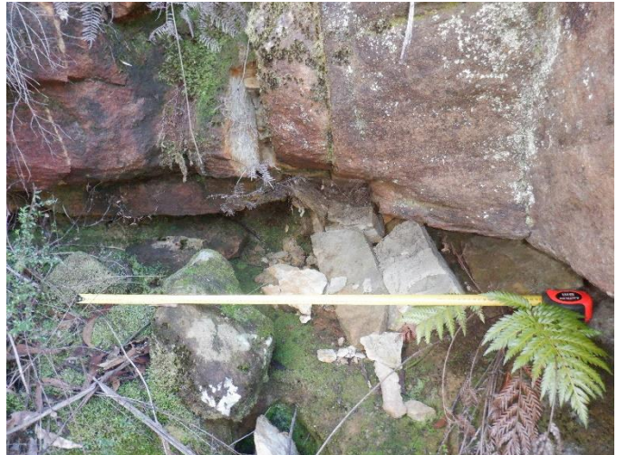
Photo 12: DA3B_LW18_017, showing rockfall. Taken 16/08/2022.
