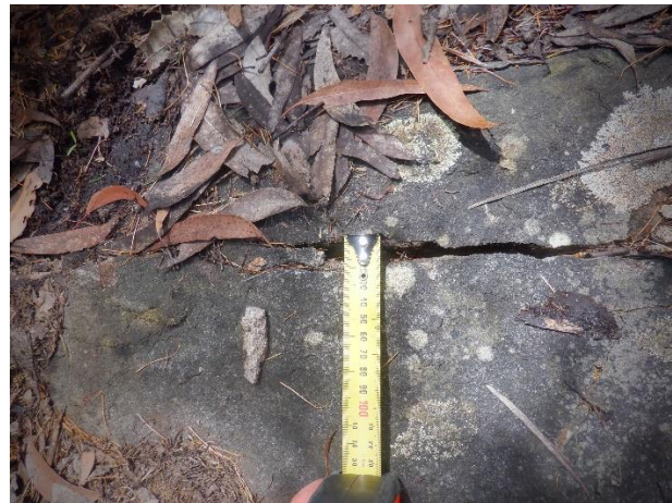
Photo 2: DA3B_LW18_001 , showing the width of the fracturing. Taken 14/12/2021.
