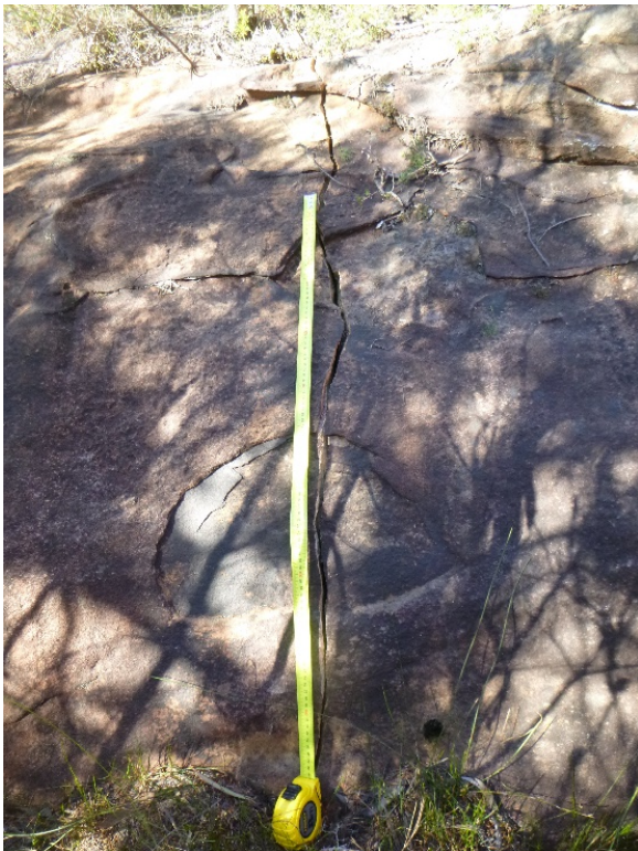
Photo 1: DA3B_LW18_007 , showing a section of rock fracturing. Taken 8/06/2022.
