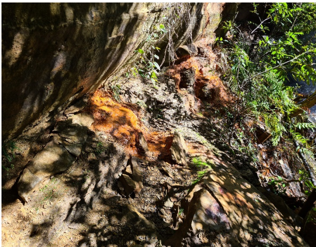
Photo 5: DA3B_LW17_041, showing a section of iron staining. Taken 2/08/2022.
