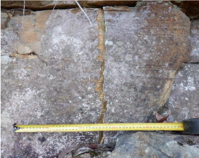
Photo 7: DA3B_LW18_015 , showing overview of rock fracture. Taken 16/08/2022.
