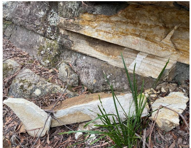
Photo 14: DA3B_LW18_018 , showing section of rockfall. Taken 16/08/2022.
