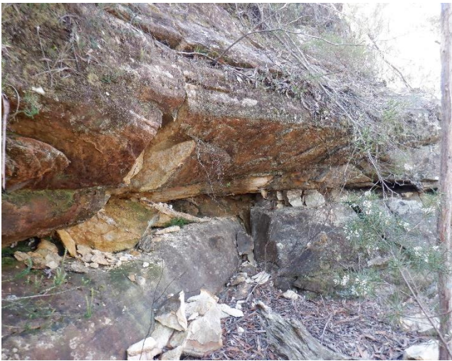
Photo 13: DA3B_LW18_018 , showing section of rockfall and rock fracturing. Taken 16/08/2022.
