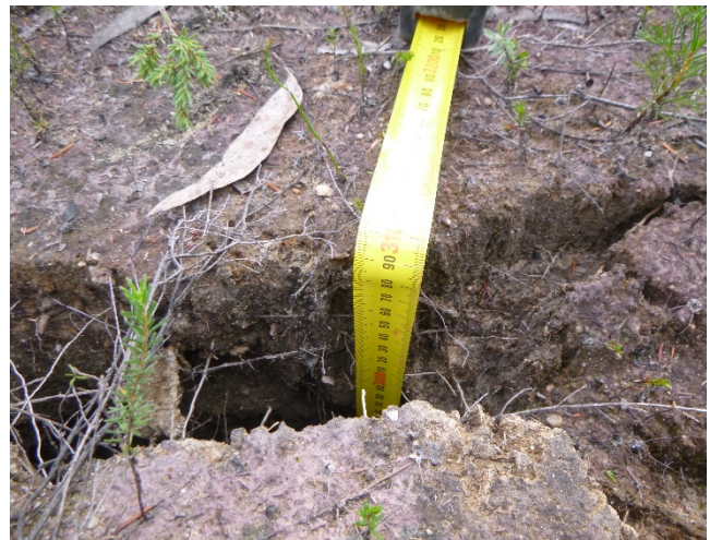
Photo 2: DA3B_LW18_005, showing the depth of soil cracking. Taken 30/06/2022.
