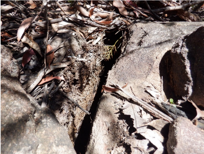
Photo 3: DA3B_LW18_005, showing a section of displacement. Taken 9/02/2022.
