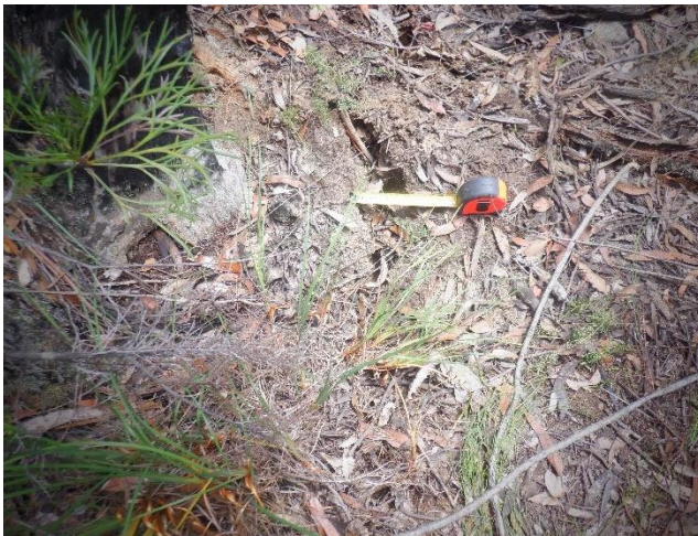
Photo 1: DA3B_LW18_006 , showing a section of soil cracking. Taken 15/02/2022.
