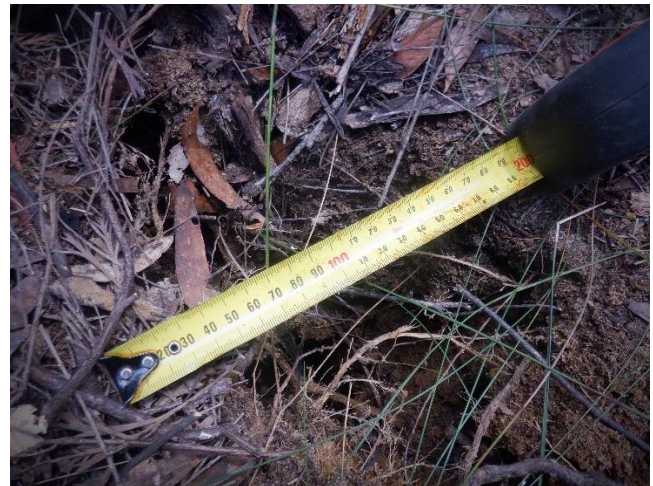
Photo 2: DA3B_LW18_006 , showing the width of the soil cracking. Taken 15/02/2022.
