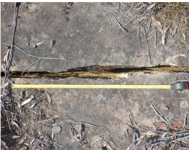
Photo 21: DA3B_LW18_021 , showing section of rock fracturing. Taken 16/08/2022.
