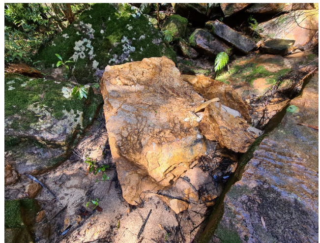
Photo 2: DA3B_LW17_041 , showing a section of potential rock fall. Taken 2/08/2022.
