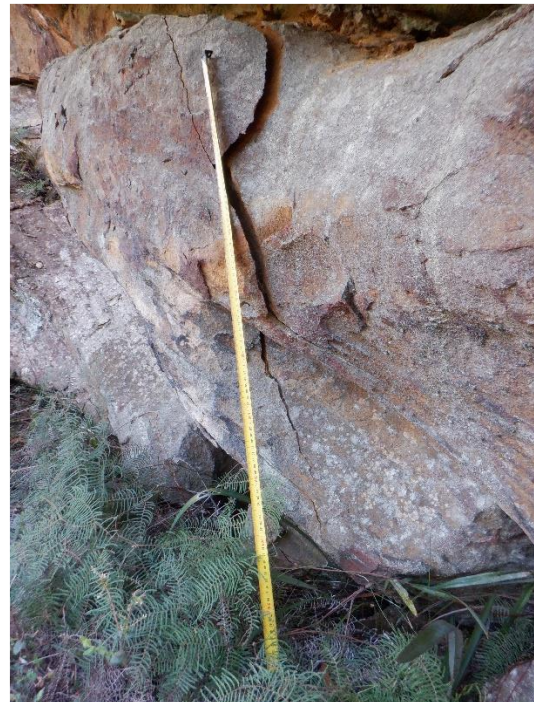
Photo 16 DA3B_LW18_018 , showing section of rock fracturing. Taken 16/08/2022.
