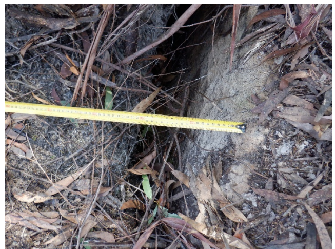
Photo 6: DA3B_LW18_009 , showing the width of rock displacement. Taken 9/06/2022.
