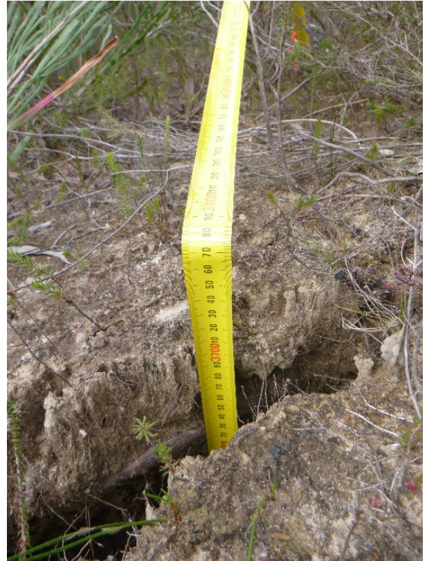
Photo 4: DA3B_LW18_012, showing depth of soil cracking. Taken 30/06/2022.
