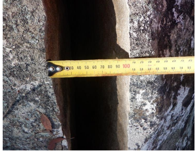
Photo 10: DA3B_LW18_016, showing maximum width of rock fracturing. Taken 16/08/2022
