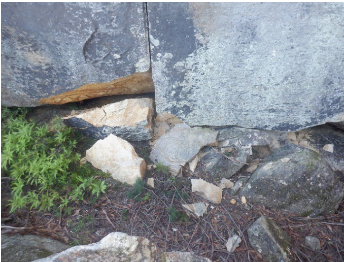
Photo 43: DA3B_LW18_010 , showing rock fall and fragmentation. Taken 10/06/2022.
