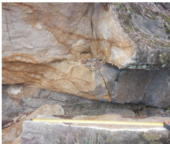
Photo 74: DA3B_LW18_022 , showing section of rockfall/debris. Taken 16/08/2022.
