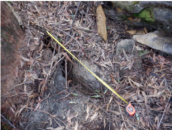
Photo 39: DA3B_LW18_009, showing a section of rock displacement. Taken 9/06/2022.
