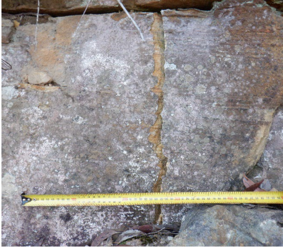
Photo 55: DA3B_LW18_015 , showing overview of rock fracture. Taken 16/08/2022.
