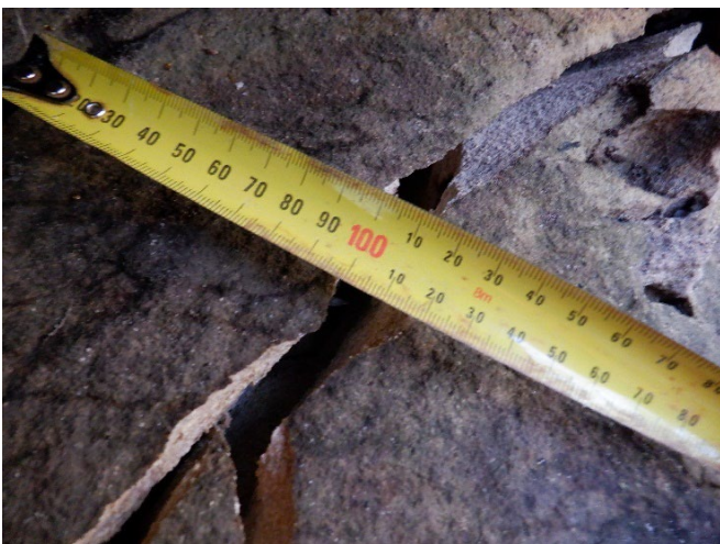
Photo 41: DA3B_LW18_009, showing width of rock fracturing. Taken 9/06/2022.
