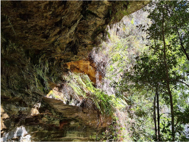
Photo 11: DA3B_LW17_041 , showing site of rock fall. Taken 2/08/2022.
