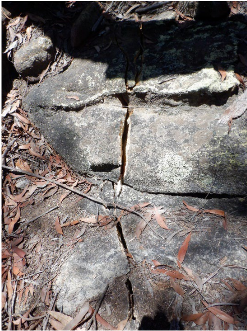
Photo 25: DA3B_LW18_004 , showing the length of rock fracturing. Taken 9/02/2022.
