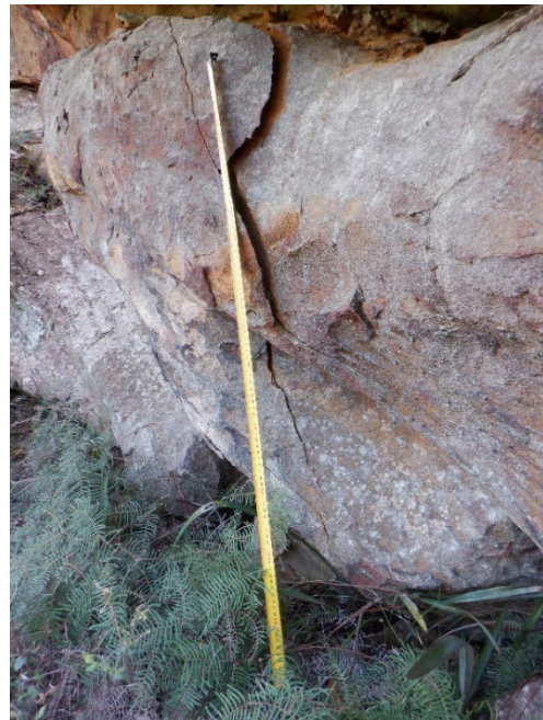
Photo 64: DA3B_LW18_018 , showing section of rock fracturing. Taken 16/08/2022.
