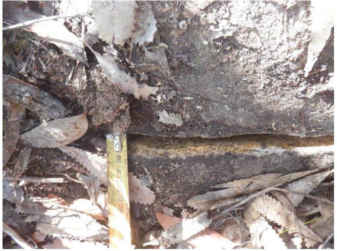
Photo 20: DA3B_LW18_002 , showing the width of the fracturing. Taken 31/01/2022.
