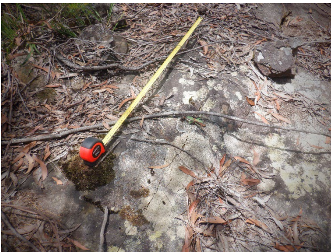
Photo 17: DA3B_LW18_001, showing a section of rock fracturing. Taken 14/12/2021.
