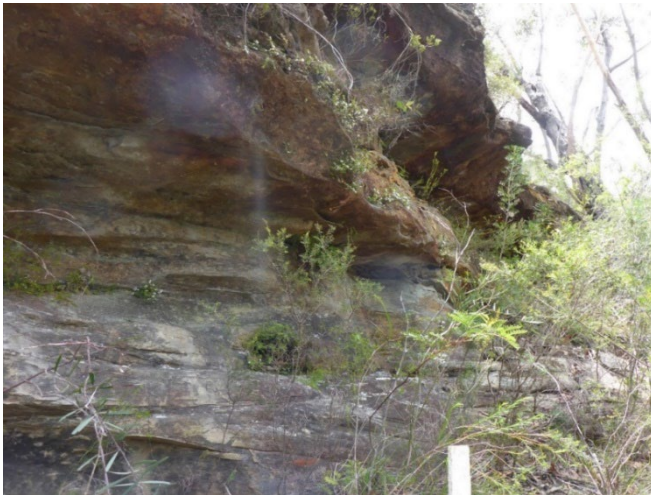
Photo 1: A3b-SS20, baseline inspection. Taken on 5/12/2017.
