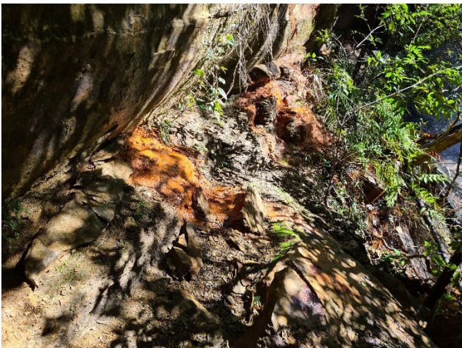
Photo 15: DA3B_LW17_041 , showing a section of iron staining. Taken 2/08/2022.
