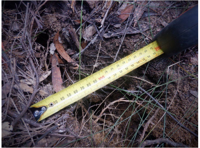
Photo 33: DA3B_LW18_006 , showing the width of soil cracking. Taken 15/02/2022.
