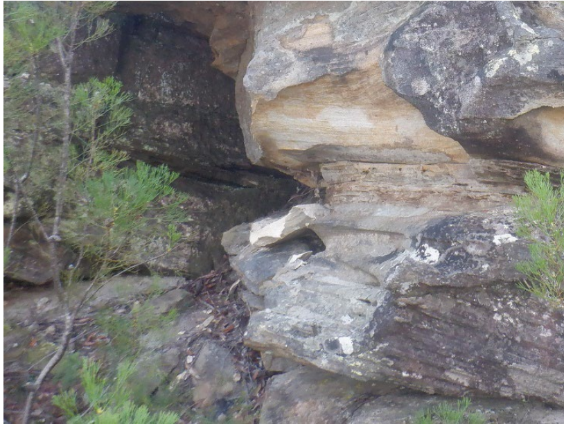
Photo 45: DA3B_LW18_011 , showing rock fall. Taken 10/06/2022.
