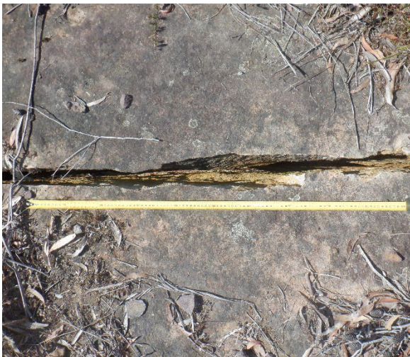
Photo 69: DA3B_LW18_021 , showing section of rock fracturing. Taken 16/08/2022.
