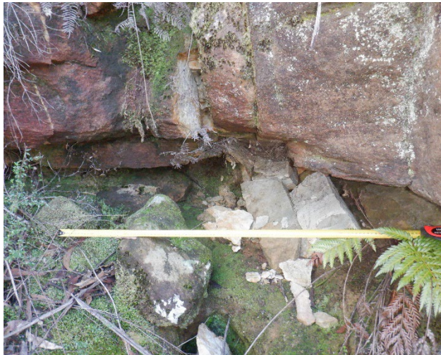
Photo 60: DA3B_LW18_017, showing rockfall. Taken 16/08/2022.
