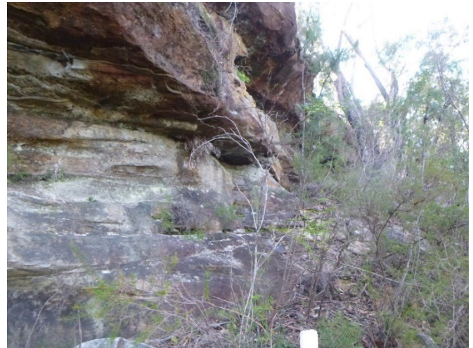
Photo 2: A3b-SS20, post-mining inspection. Taken on 6/08/2022.
