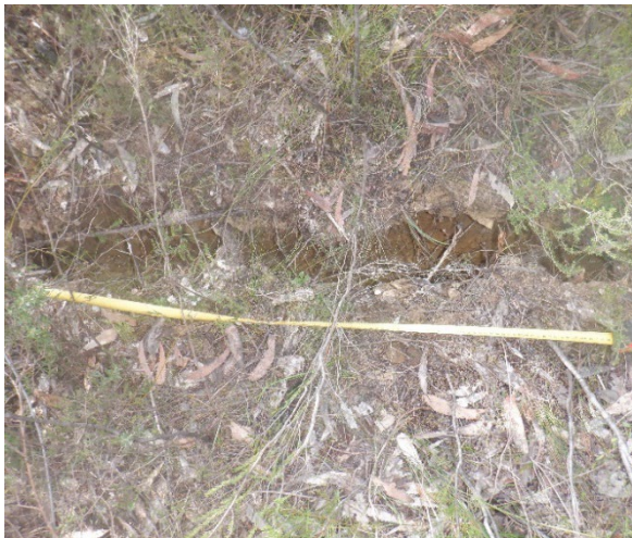
Photo 75: DA3B_LW18_023, showing section of soil cracking. Taken 16/08/2022.
