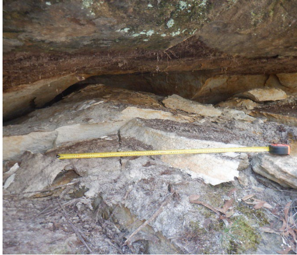
Photo 68: DA3B_LW18_020 , showing rockfall closer up. Taken 16/08/2022.
