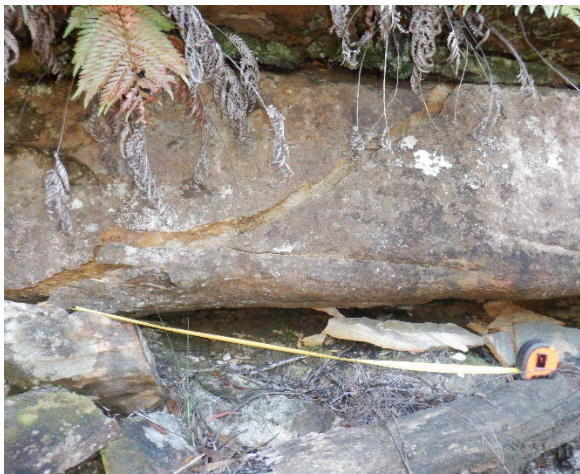
Photo 53: DA3B_LW18_014 , showing section of rock fracturing. Taken 16/08/2022.
