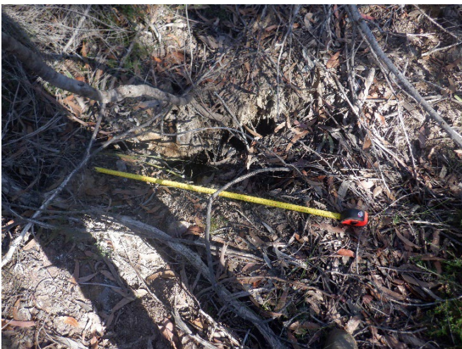
Photo 37: DA3B_LW18_008 , showing a section of soil cracking. Taken 9/06/2022.
