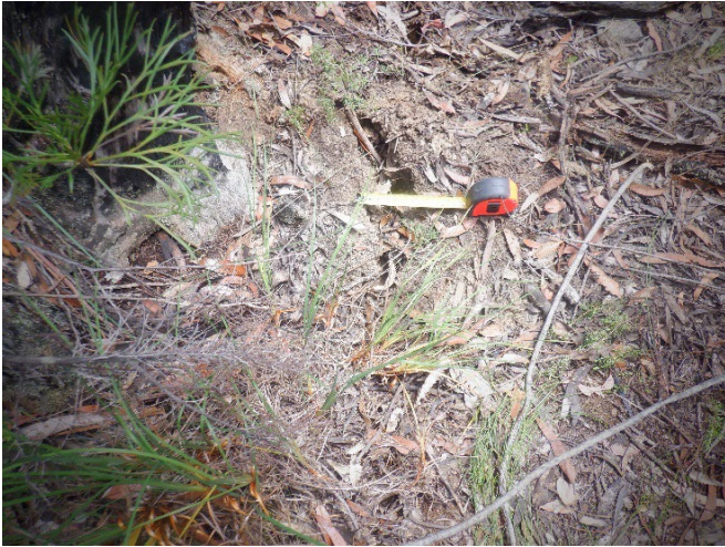
Photo 32: DA3B_LW18_006 , showing a section of soil cracking. Taken 15/02/2022.
