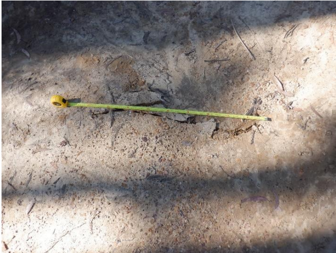
Photo 32: DA3B_LW17_015 , soil cracking on access track. Taken on 18/05/2021.
