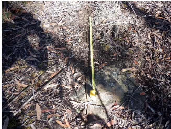
Photo 18: DA3B_LW17_016, rock fracturing west of Fire Road 6A. Taken on 25/05/2021.
