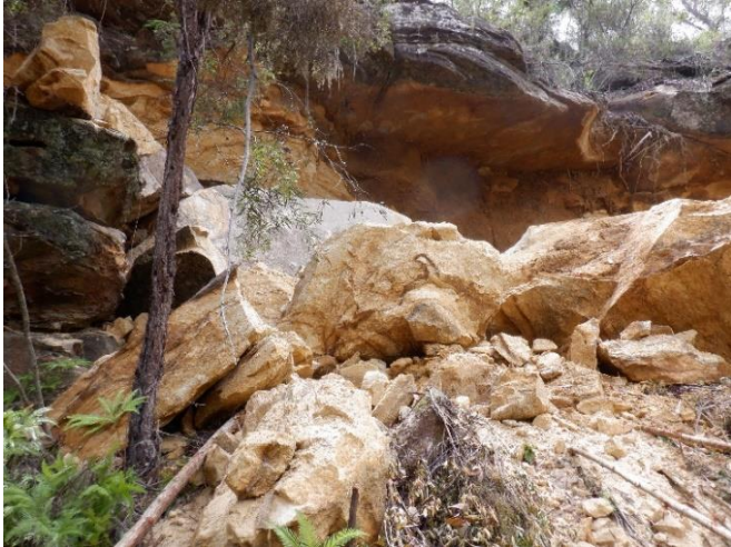
Photo 14: DA3B_LW17_008, rockfall north of LA2. Taken on 10/03/2021.
