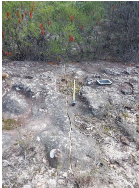
Photo 24: DA3B_LW17_024 , rock fracturing adjacent to Fire Road 6A . Taken on 24/06/2021.
