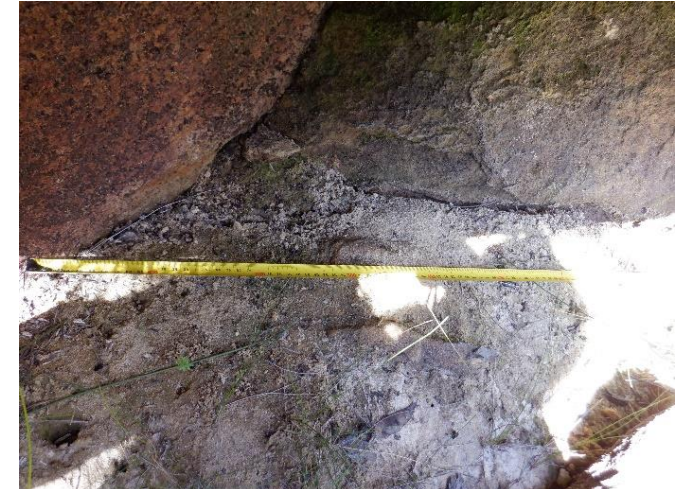
Photo 25: DA3B_LW17_032 , rock displacement east of Fire Road 6A . Taken on 17/08/2021.
