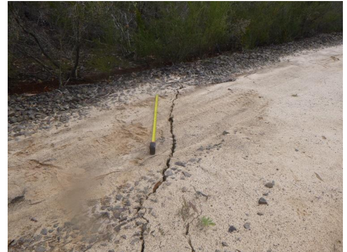
Photo 37: DA3B_LW17_029 , soil cracking on railway corridor. Taken on 26/07/2021.
