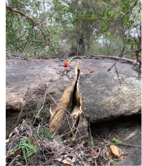
Photo 28: DA3B_LW17_037 , rock fracturing west of Fire Road 6A . Taken on 15/09/2021.
