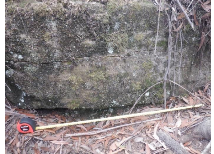
Photo 16: DA3B_LW17_010, rock fracturing north of LA2. Taken on 10/09/2021.
