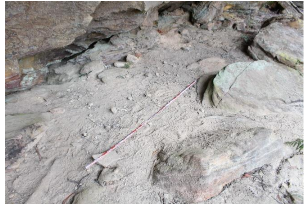
Plate 10: General photo of shelter floor, facing north from Niche (2021) monitoring survey for the Longwall 16 End of Panel report. Photo taken: 20 January 2021
