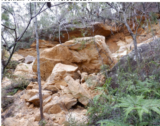
Photo 55: DA3B_LW17_008, looking at a section of rockfall. Taken on 10/03/2021.
