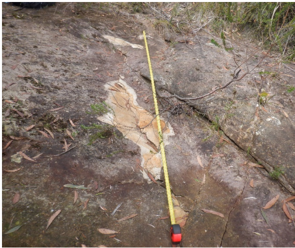
Photo 9: DA3B_LW17_004, looking at a section of rock fracturing. Taken on 10/09/2021.
