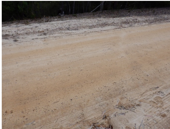
Photo 110: DA3B_LW17_018 – soil crack naturally remediated. Taken 16/09/2021
