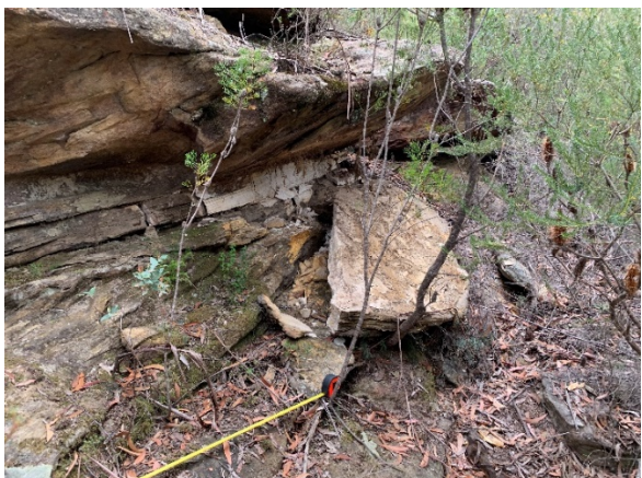
Photo 87: DA3B_LW17_035, showing the rockfall associated with rock fracturing. Taken 15/9/2021.
