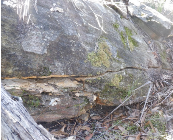
Photo 74: DA3B_LW17_021, looking at a section of rock fracturing. Taken on 8/06/2021
