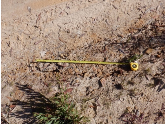
Photo 111: DA3B_LW17_020- soil crack on Fire Road 6A. Taken on 8/06/2021
