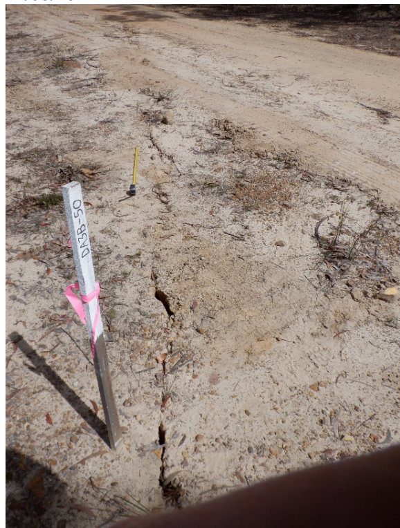
Photo 120: DA3B_LW17_030- soil cracking on Fire Road 6A has been remediated, soil cracking to the side of the fire road remains. Taken on 21/09/2021.
