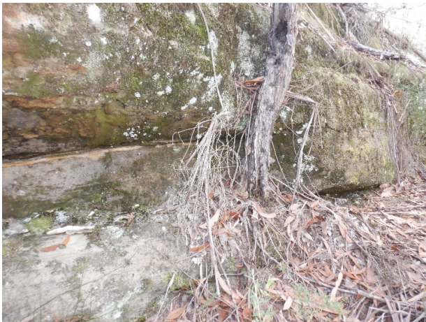
Photo 61: DA3B_LW17_010, fracturing along step. Taken on 13/04/2021.
