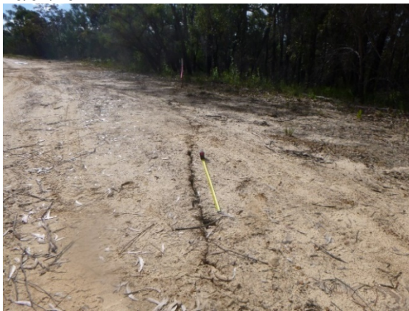
Photo 119: DA3B_LW17_030- soil cracking on Fire Road 6A. Taken on 26/07/2021.
