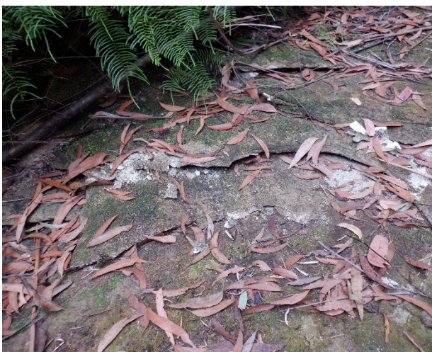
Photo 16: DA3B_LW17_007, looking at a section of rock fracturing. Taken on 10/03/2021.
