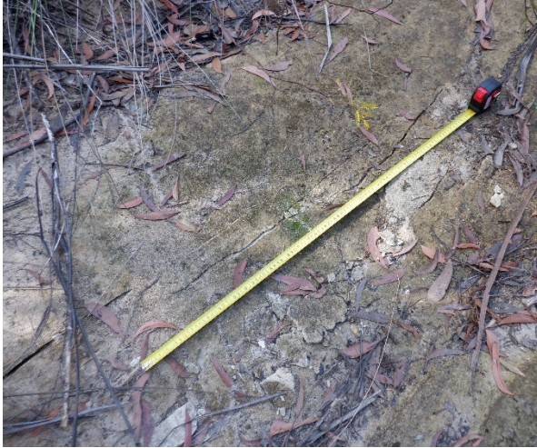
Photo 11: DA3B_LW17_005, looking at a section of rock fracturing. Taken on 10/03/2021.
