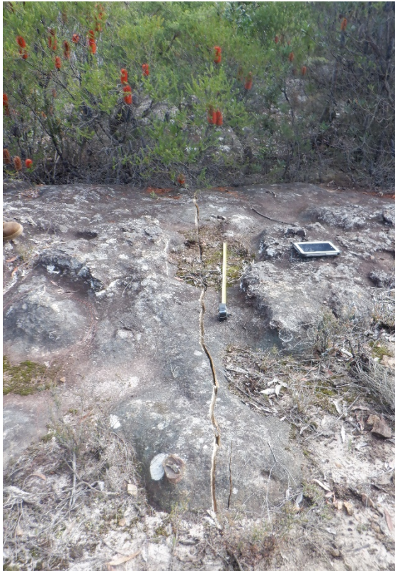
Photo 82: DA3B_LW17_024 , looking at a section of rock fracturing. Taken on 24/06/2021
