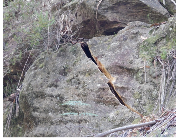
Photo 64: DA3B_LW17_011, zoomed in photo of fracture to step. Taken on 13/04/2021.
