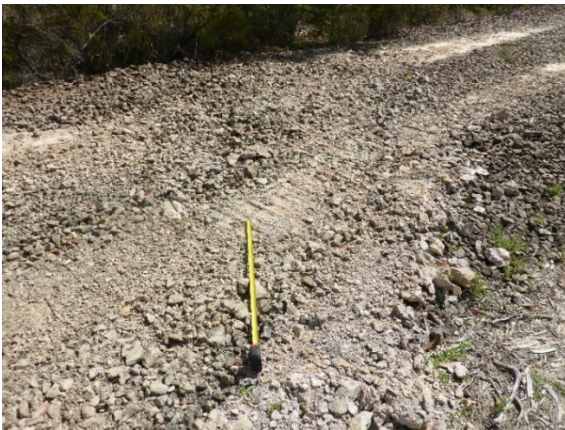
Photo 114: DA3B_LW17_26, Remediated crack on railway corridor. Taken on 22/09/2021.
