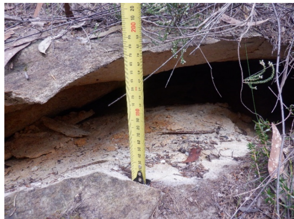
Photo 19: DA3B_LW17_002, looking at the width of rock fracturing. Taken on 10/09/2021.
