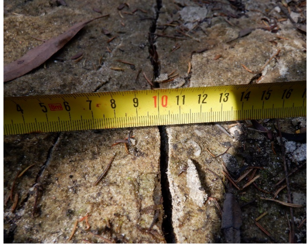
Photo 12: DA3B_LW17_005, looking at the maximum width of the rock fracturing. Taken on 10/03/2021.
