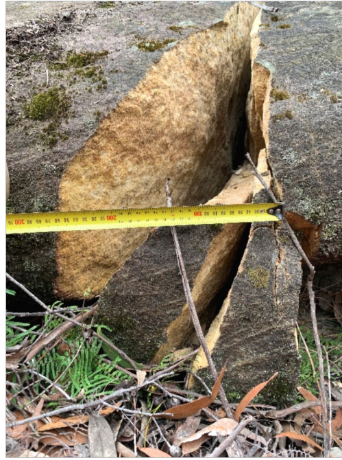
Photo 93: DA3B_LW17_037, looking at a section of rock fracturing, showing width. Taken 15/9/2021.
