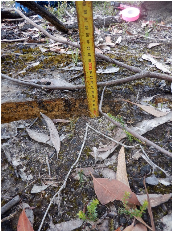
Photo 104: DA3B_LW17_040, showing the depth of the rock fracturing. Taken 21/10/2021.
