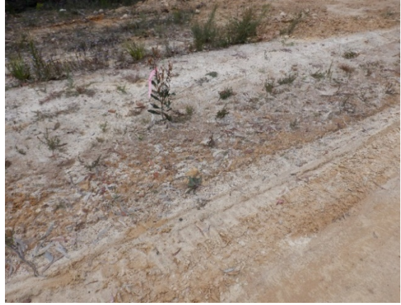
Photo 112: DA3B_LW17_020- Soil crack on Fire Road 6A naturally remediated. Taken on 16/09/2021.
