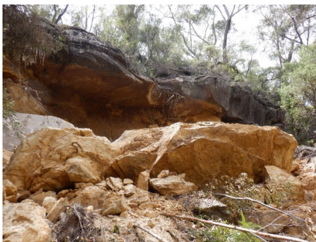
Photo 53: DA3B_LW17_008, looking at a section of rockfall. Taken on 10/03/2021.
