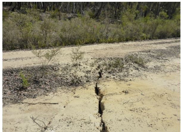
Photo 124: DA3B_LW17_014- soil cracking extending across Fire Road 6A and adjacent area. Taken on 18/05/2021.
