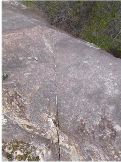
Photo 7: DA3B_LW16_010, an overview of the rock fracture. Taken on 27/04/2020.
