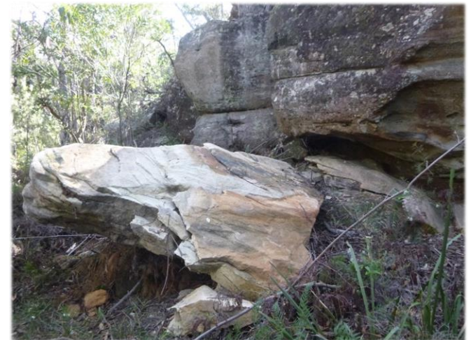
Photo 18: DA3B_LW16_029, rockfall from step, looking at main large rock fragment. Taken on 31/08/2020.
