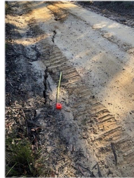
Photo 39: DA3B_LW16_019, looking at length of soil cracking on FR6A . Taken on 23/06/2020.
