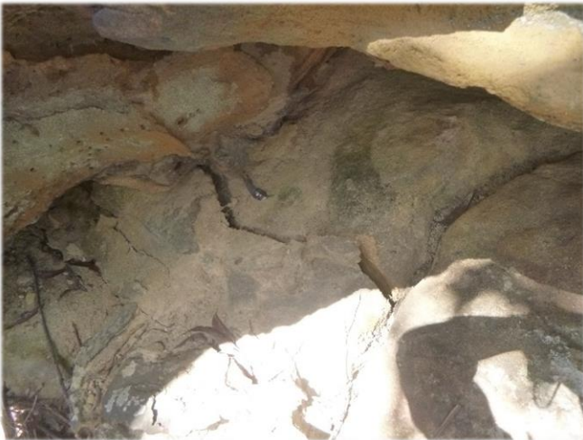
Photo 22: DA3B_LW16_036, looking at a section of rock fracturing. Taken on 28/09/2020.
