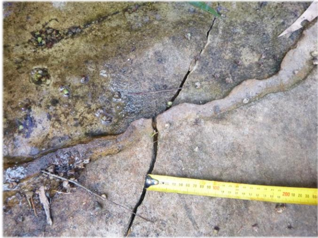
Photo 1: DA3B_LW16_028, rock fracture across rockbar. Taken on 31/08/2020.
