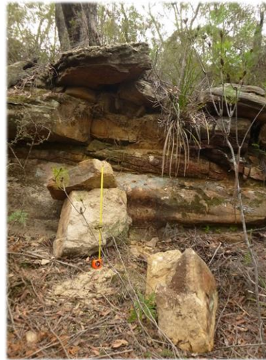
Photo 11: DA3B_LW16_016, overview of the rockfall. Taken on 15/05/2020.
