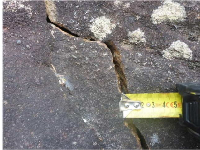
Photo 26: DA3B_LW16_047, looking at the rock fracture. Taken on 25/11/2020.
