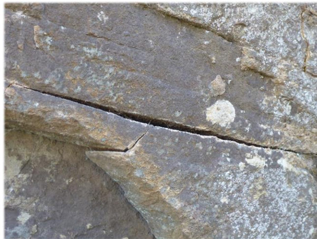
Photo 17: DA3B_LW16_026, looking at a section of rock fracturing. Taken on 06/08/2020.
