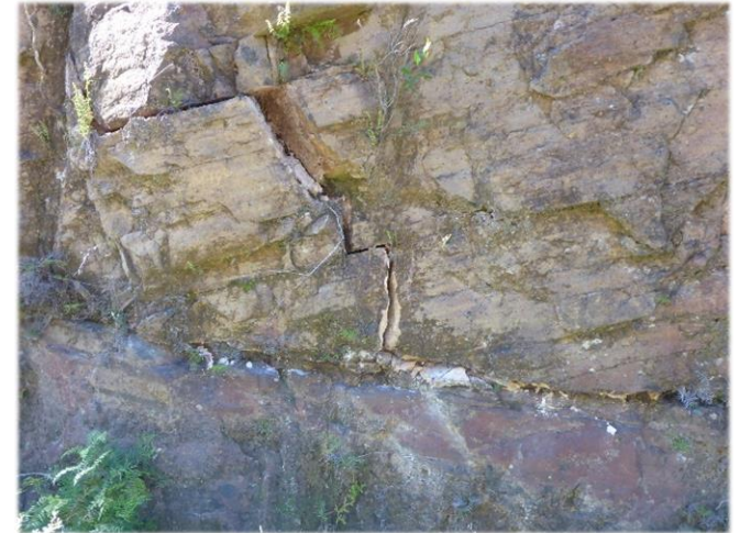
Photo 15: DA3B_LW16_022, fracturing down face of cut-through. Taken on 6/08/2020.
