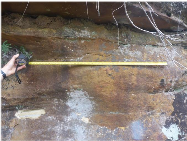
Photo 28: DA3B_LW16_049, looking at a section of rock fracturing. Taken on 30/11/2020.
