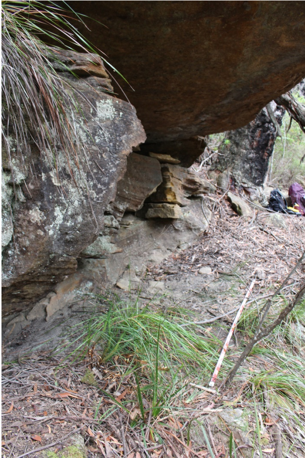
Plate 3: Close up of shelter roof and backwall facing south-east. Photo taken: 20 January 2021.
