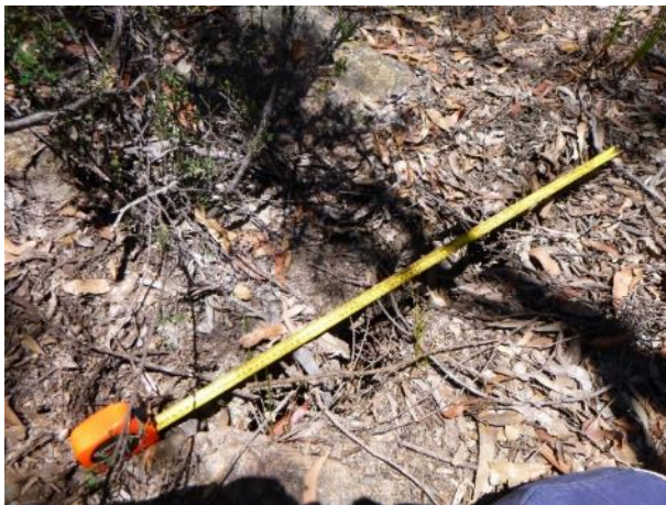
Photo 72: DA3B_LW16_044 , looking at length of soil cracking. Crack runs in orientation of tape measure. Taken on 10/11/2020.
