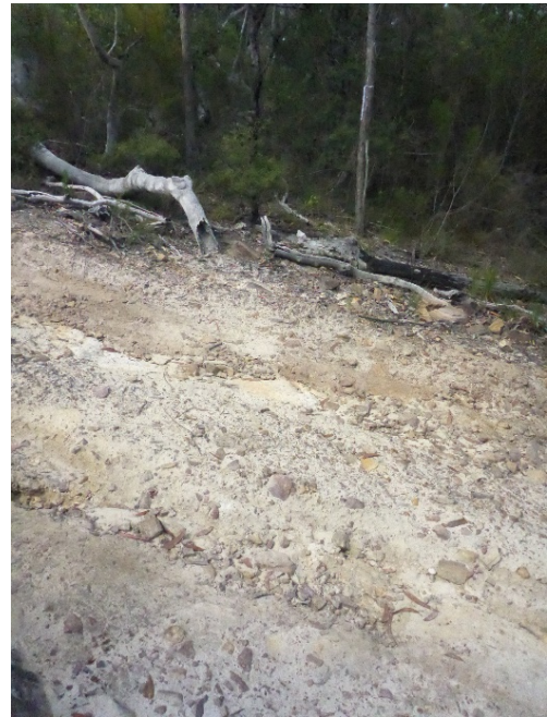
Photo 106: DA3B_LW16_004, soil cracking naturally remediated. Taken on 19/11/2020.
