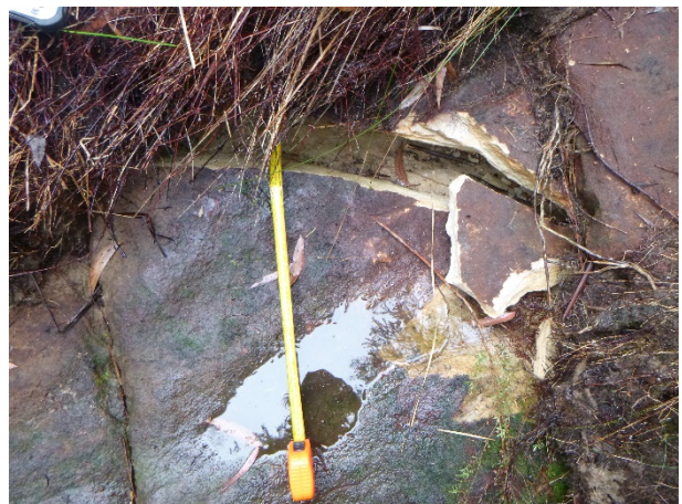
Photo 14: DA3B_LW14_017, looking at the rock fracturing and displacement. Taken on 9/09/2020.
