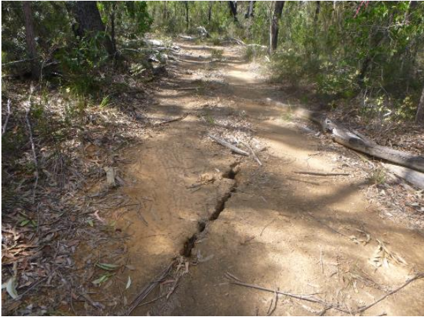
Photo 123: DA3B_LW16_027, soil cracking across Fire Road 6P. Taken on 21/08/2020.
