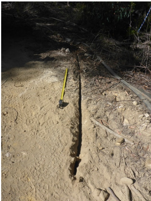
Photo 103: DA3B_LW16_003, soil cracking and rock fracturing on access track between Lake Avon and FR6A. Taken on 22/04/2020.
