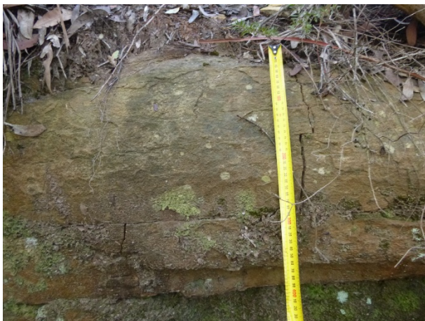
Photo 94: DA3B_LW15_002, looking at a section of rock fracturing. Taken on 05/05/2020.
