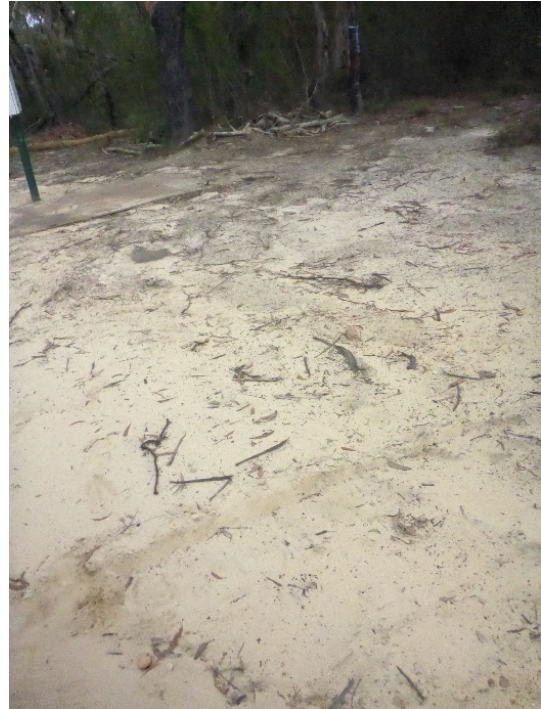
Photo 144: DA3B_LW16_005, soil cracking remediated naturally. Taken on 19/11/2020.
