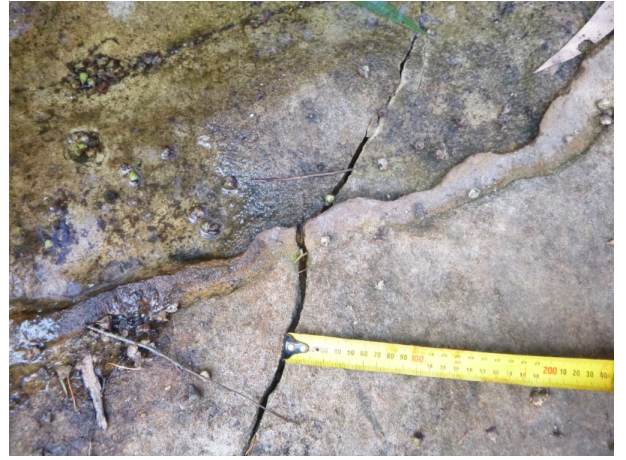
Photo 8: DA3B_LW16_028 , rock fracture across rockbar. Taken on 31/08/2020.
