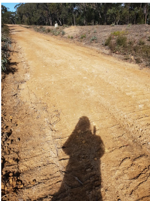
Photo 151: DA3B_LW16_019, remediated soil cracking on FR6A. Taken on 29/06/2020.
