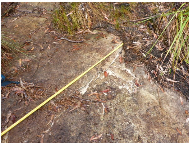
Photo 11: DA3B_LW16_028 , looking at additional rock fracturing. Taken on 25/11/2020.
