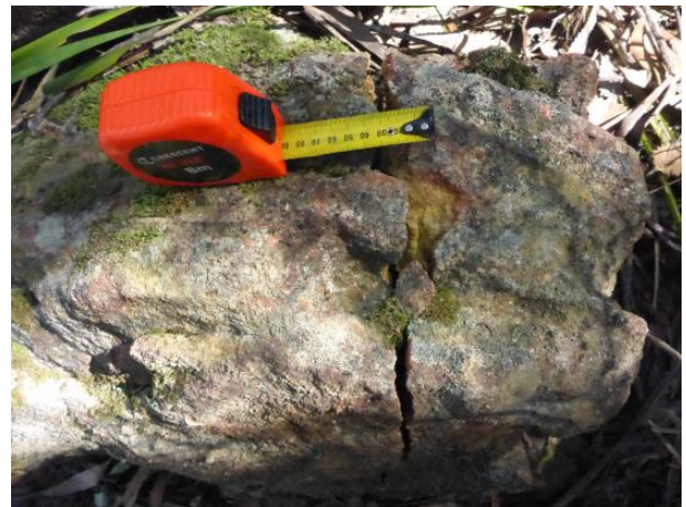
Photo 98: DA3B_LW15_026, looking at fracture to boulder. Taken on 24/08/2020.
