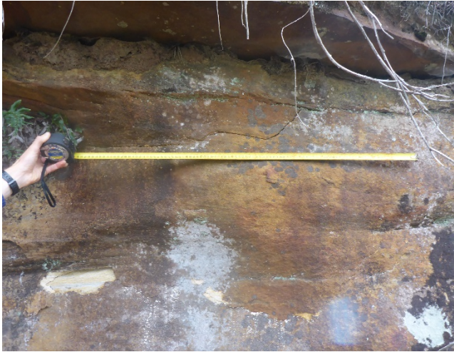
Photo 85: DA3B_LW16_049, looking at a section of rock fracturing. Taken on 30/11/2020.
