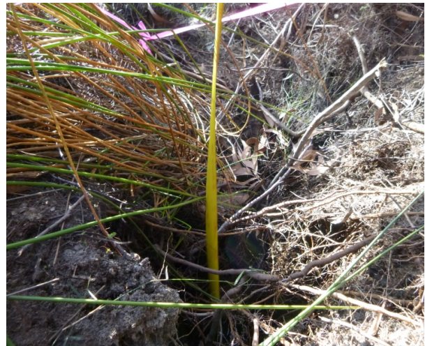
Photo 63: DA3B_LW16_030, looking at measurable depth of localised erosion. Taken on 31/08/2020.
