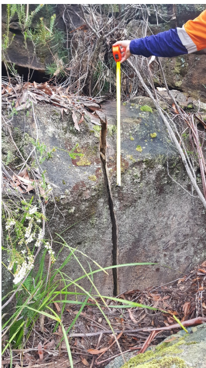
Photo 28: DA3B_LW16_012, looking at a section of rock fracturing. Taken on 28/04/2020.
