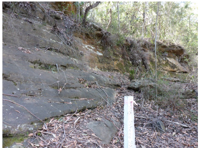
Photo 2: A3b-SS16, post-mining inspection. Taken on 28/09/20.
