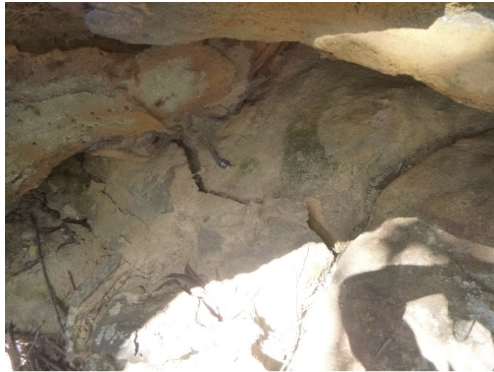
Photo 71: DA3B_LW16_036 , looking at a section of rock fracturing. Taken on 28/09/2020.
