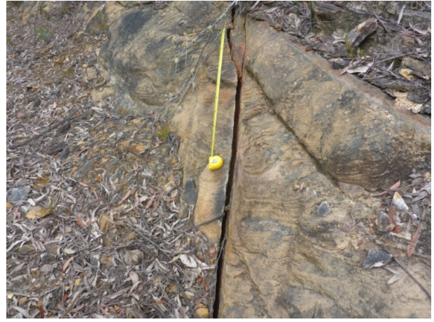
Photo 46: DA3B_LW16_022, fracturing down face of cut-through. Taken on 7/07/2020.
