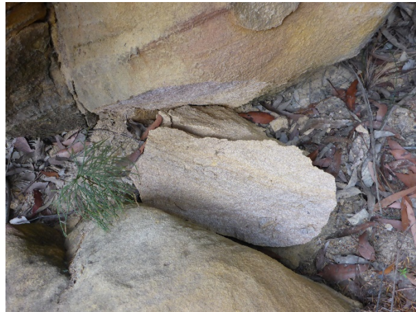
Photo 70: DA3B_LW16_035, looking at the rock fall. Taken on 30/11/2020.
