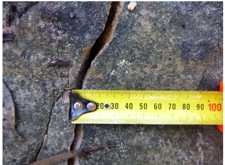
Photo 38: DA3B_LW16_017, looking at width of rock fracturing. Taken on 16/06/2020.
