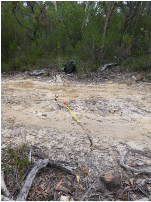
Photo 105: DA3B_LW16_004, soil cracking on access track between Lake Avon and FR6A. Taken on 16/04/2020.
