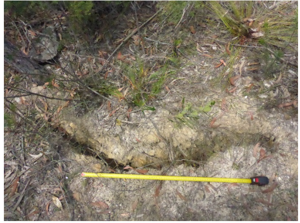
Photo 148: DA3B_LW16_013, looking at soil cracking adjacent to access track. Taken on 19/11/2020.
