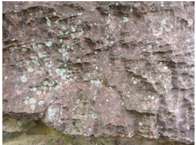
Photo 80: DA3B_LW16_046, looking at the rock fracture. Taken on 25/11/2020.
