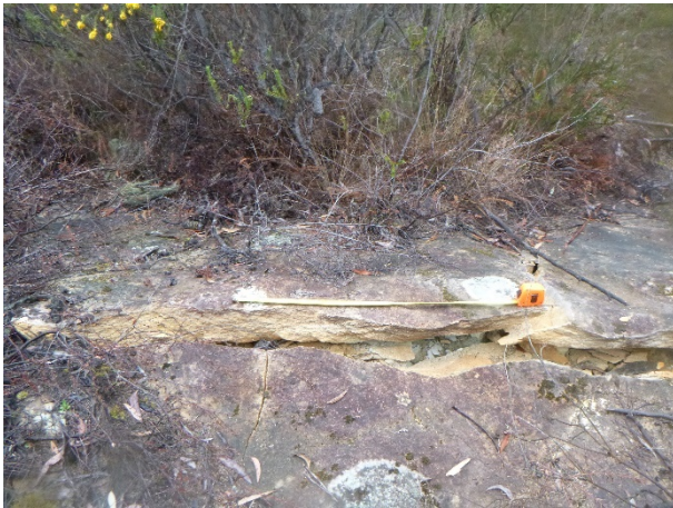
Photo 15: DA3B_LW14_019, looking at a section of rock fracturing and uplift. Taken on 9/09/2020.
