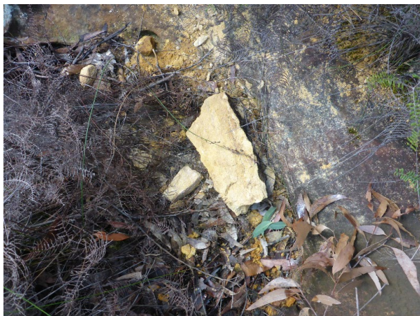
Photo 43: DA3B_LW16_021, looking at small rock fragments fallen from step. Taken on 30/06/2020.
