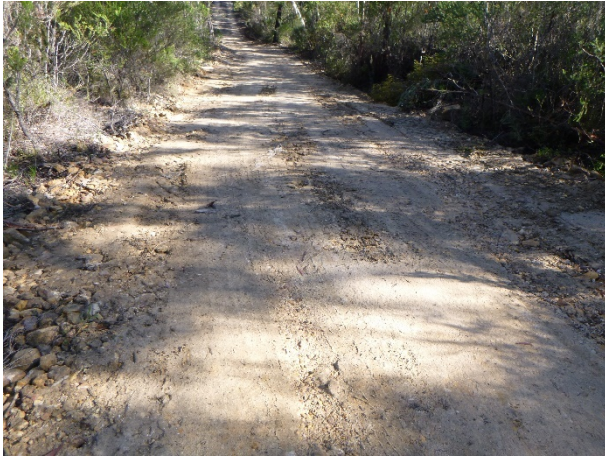
Photo 147: DA3B_LW16_013, looking at the remediated access track. Taken on 11/06/2020.
