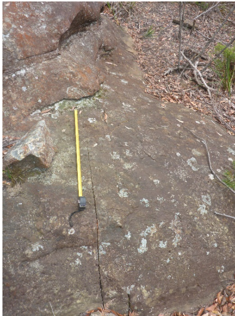
Photo 53: DA3B_LW16_025 , looking at additional rock fracturing. Taken on 30/11/2020.
