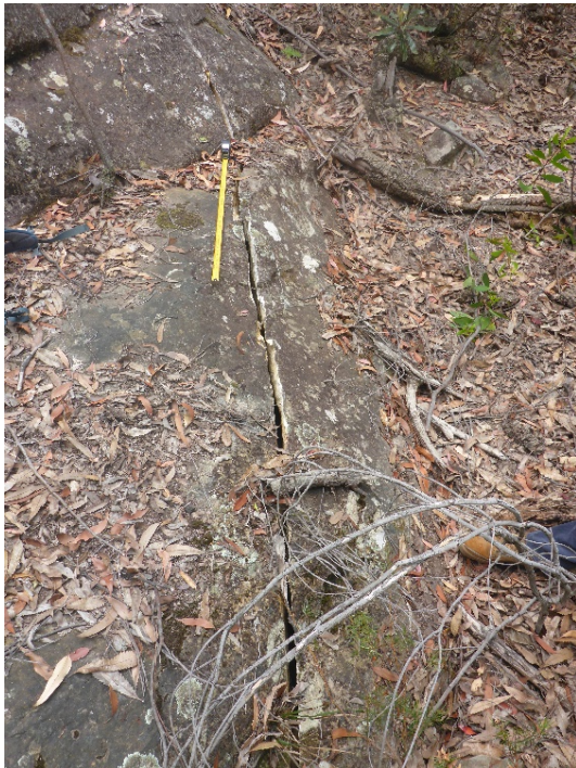
Photo 83: DA3B_LW16_048, looking at the length of rock fracturing. Taken on 30/11/2020.
