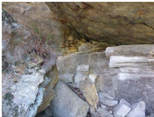
Photo 65: DA3B_LW16_031, looking at the rockfall. Taken on 28/09/2020.
