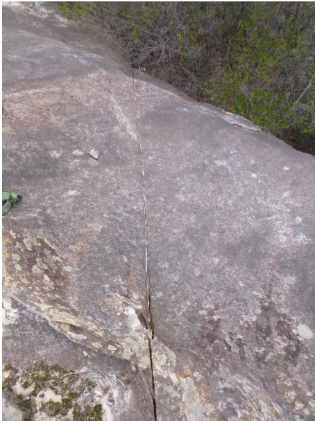
Photo 24: DA3B_LW16_010, an overview of the rock fracture. Taken on 27/04/2020.
