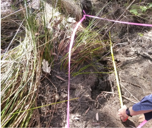
Photo 60: DA3B_LW16_030, localised erosion observed on tributary WC15. Taken on 31/08/2020.
