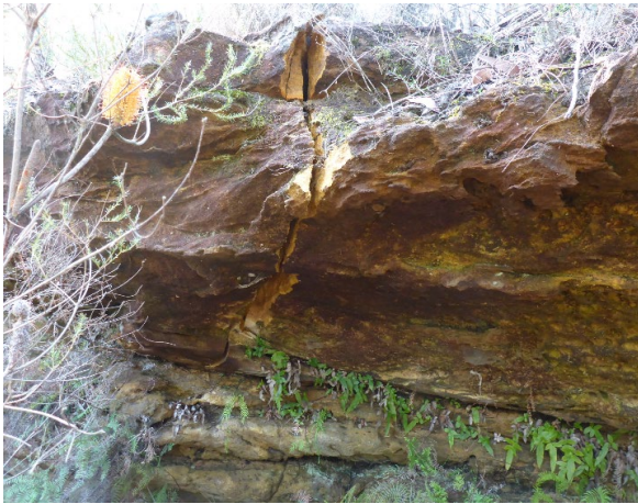
Photo 41: DA3B_LW16_021, looking at fracture on step. Taken on 30/06/2020.
