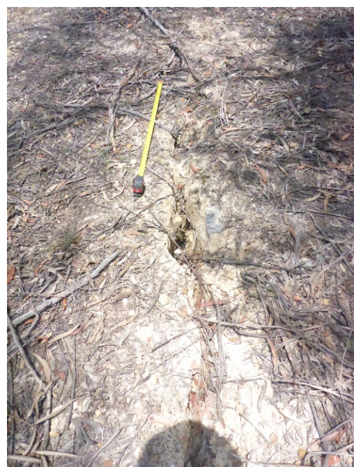
Photo 152: DA3B_LW16_019, looking at soil cracking adjacent to FR6A. Taken on 19/11/2020
