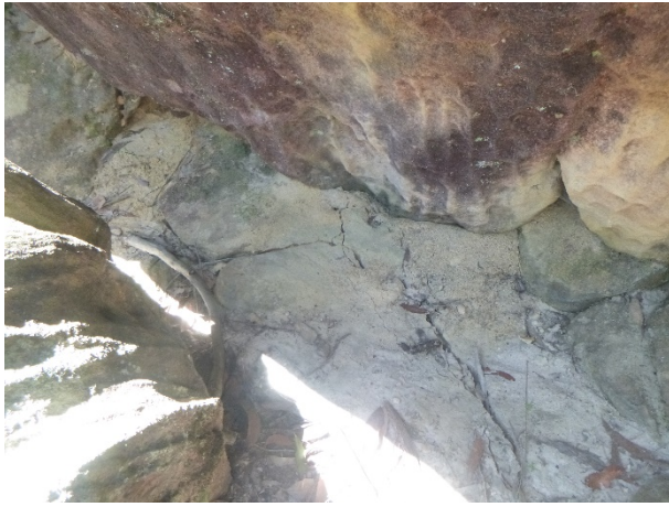
Photo 68: DA3B_LW16_035, looking at a section of soil cracking. Taken on 28/09/2020.
