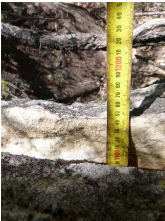
Photo 76: DA3B_LW16_045, looking at depth of rock fracturing. Taken on 10/11/2020.
