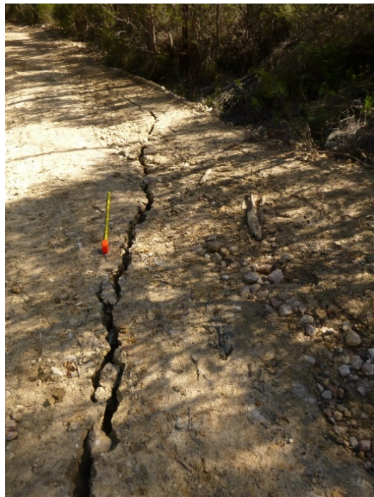
Photo 145: DA3B_LW16_013, soil cracking to access track between Lake Avon and FR6A. Taken on 12/05/2020.
