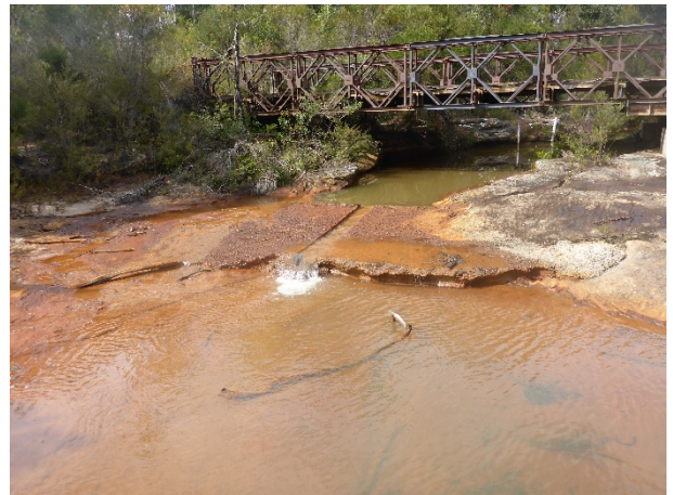
Photo 22: SCK_Rockbar 5, looking upstream at the increase in iron staining. Taken on 14/10/2020.
