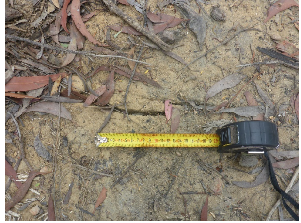
Photo 130: DA3B_LW16_037, small soil crack expected to naturally remediate. Taken on 28/09/2020.
