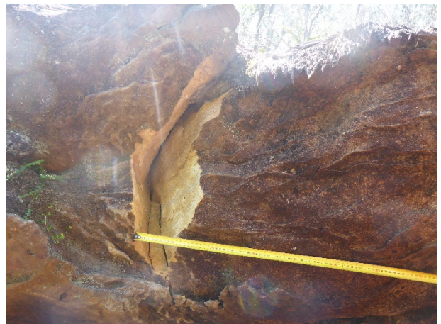
Photo 44: DA3B_LW16_021, looking at additional rock fracturing and rock fall. Taken on 1/12/2020.
