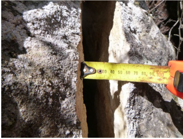
Photo 78: DA3B_LW16_045, looking at width of rock fracturing. Taken on 10/11/2020.
