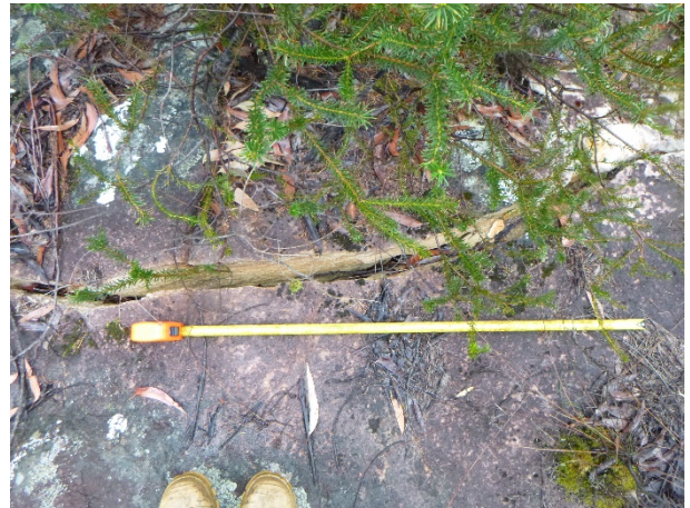
Photo 16: DA3B_LW14_019, looking at a section of rock fracturing. Taken on 9/09/2020.
