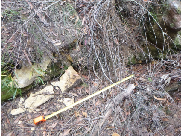
Photo 26: DA3B_LW16_011, overview of the rockfall. Taken on 27/04/2020.
