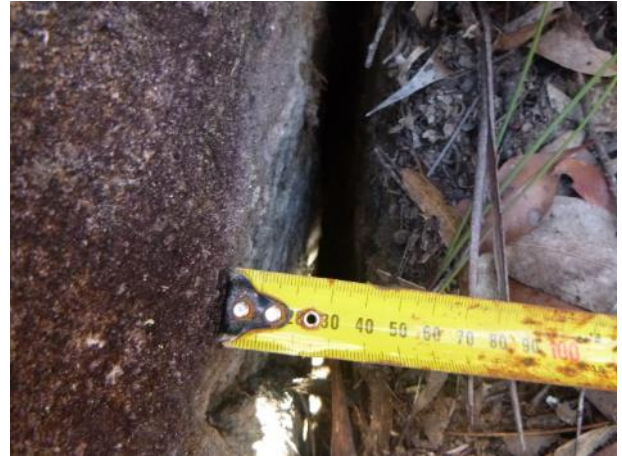
Photo 75: DA3B_LW16_044, looking at rock displacement from soil. Taken on 10/11/2020.
