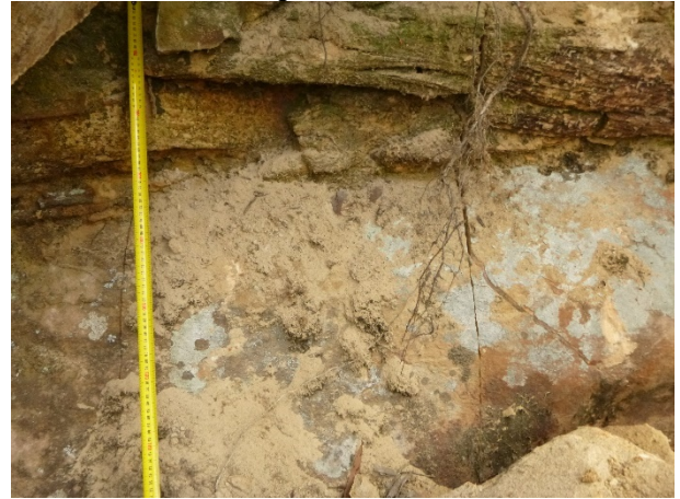
Photo 36: DA3B_LW16_016, looking at a section of rock fracturing. Taken on 15/05/2020.
