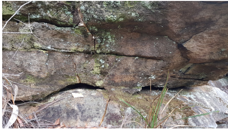
Photo 30: DA3B_LW16_012, looking at a section of rock fracturing. Taken on 28/04/2020.
