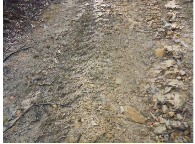
Photo 100: DA3B_LW16_001, soil cracking naturally remediated. Taken on 19/11/2020.
