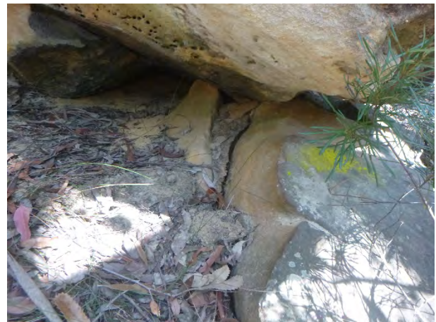
Photo 10: DA3B_LW16_035, looking at a section of displacement. Taken on 28/09/2020.
