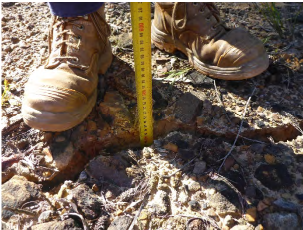
Photo 1: DA3B_LW16_019, looking at the depth of recent soil cracking. Taken on 25/06/2020.
