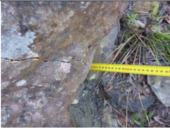
Photo 7: DA3B_LW15_026, showing fracture extending below ledge. Taken on 24/08/2020.
