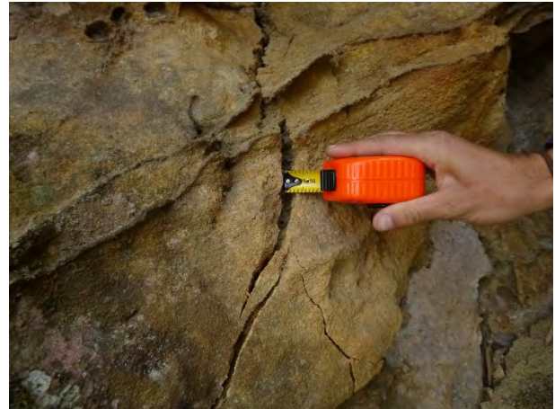
Photo 11: DA3B_LW16_015, looking at the width of rock fracturing. Taken on 15/05/2020.
