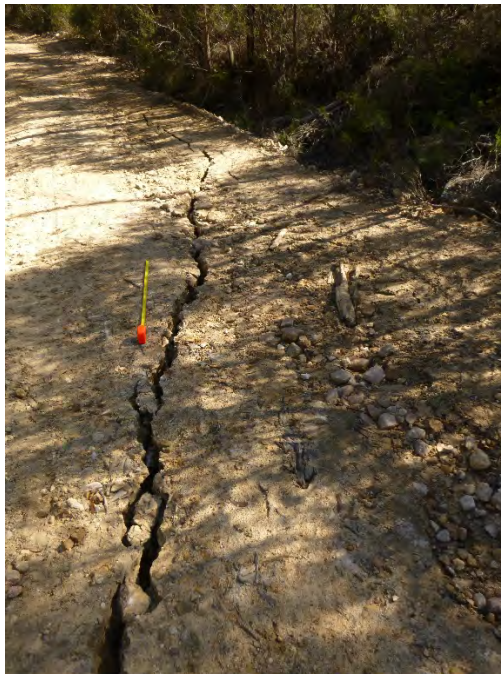
Photo 3: DA3B_LW16_013 , looking at a section of soil cracking. Taken on 12/05/2020.
