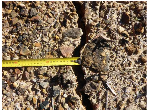
Photo 2: DA3B_LW16_019, looking at the width of recent soil cracking. Taken on 25/06/2020.
