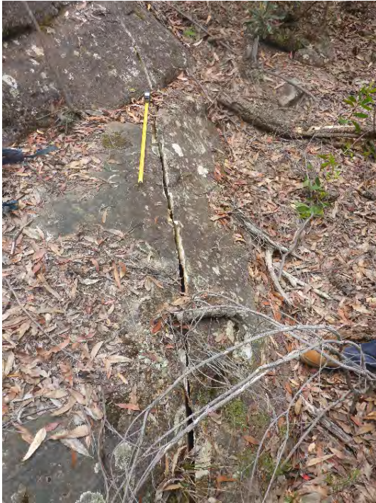
Photo 3: DA3B_LW16_048 , looking at the length of rock fracturing. Taken on 30/11/2020.
