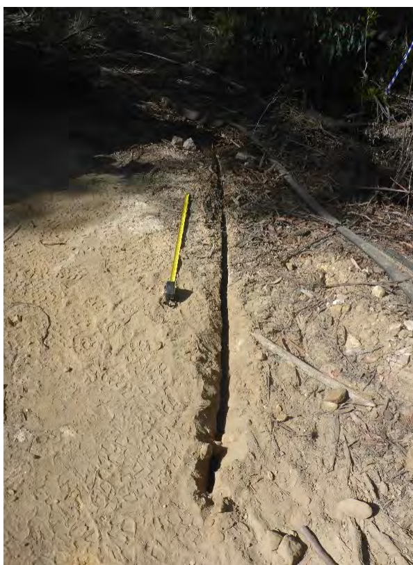
Photo 1: DA3B_LW16_003 , looking at a section of rock fracturing. Taken on 22/04/2020.
