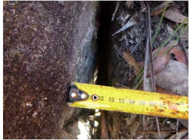
Photo 4: DA3B_LW16_044 , looking at rock displacement from soil. Taken on 10/11/2020.
