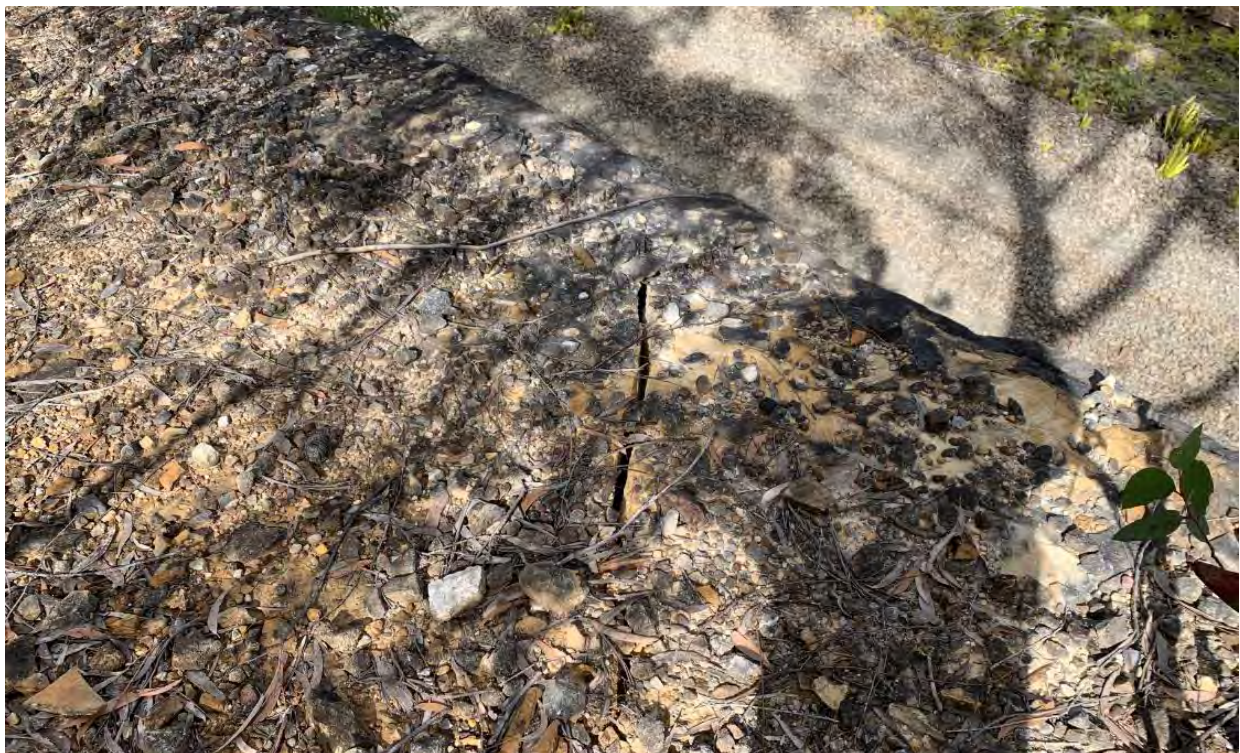
Figure 5 Propagation of joint set behind slope crest (looking south west)
