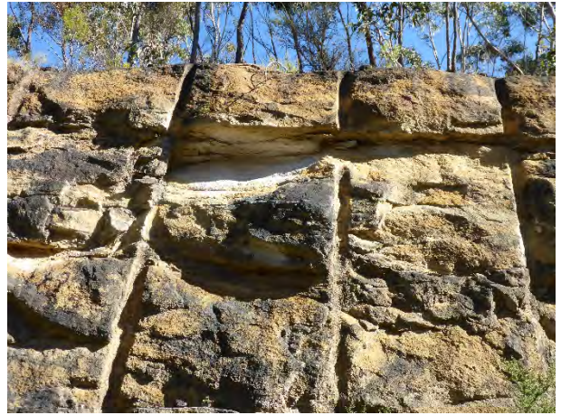
Photo 4: DA3B_LW16_022, looking at a rockfall. Taken on 6/08/2020.
