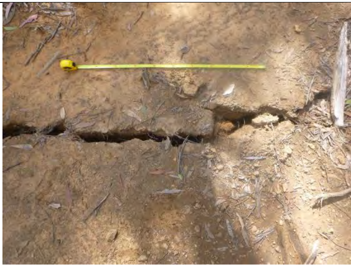
Photo 3: DA3B_LW16_027, looking down at cracking. Taken on 21/08/2020.
