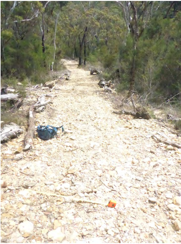
Photo 9: DA3B_LW16_042- looking down slope of access track. Taken on 7/10/2020.
