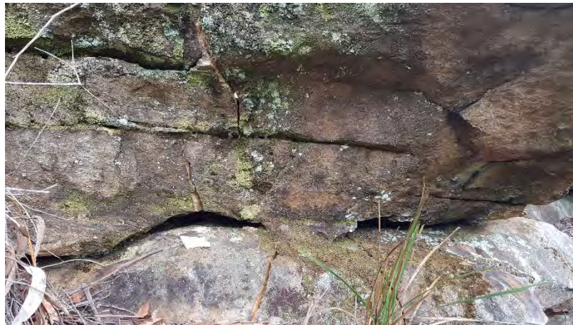
Photo 12: DA3B_LW16_012, looking at a section of rock fracturing. Taken on 28/04/2020.
