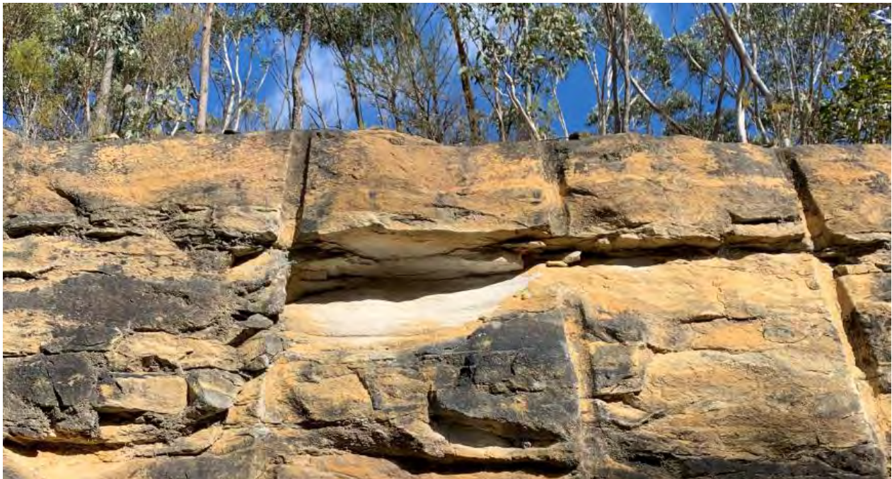
Figure 7 Recent wedge instability (intersection of bedding plane with high angle joint in southwest facing cut)
