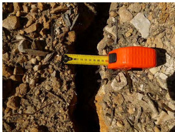
Photo 2: DA3B_LW16_013, looking at the width of soil cracking. Taken on 12/05/2020.
