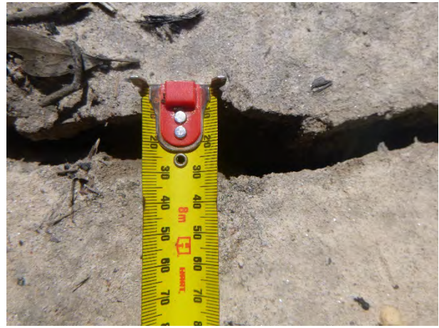
Photo 8: DA3B_LW16_034 looking at the width of soil cracking. Taken on 28/09/2020.
