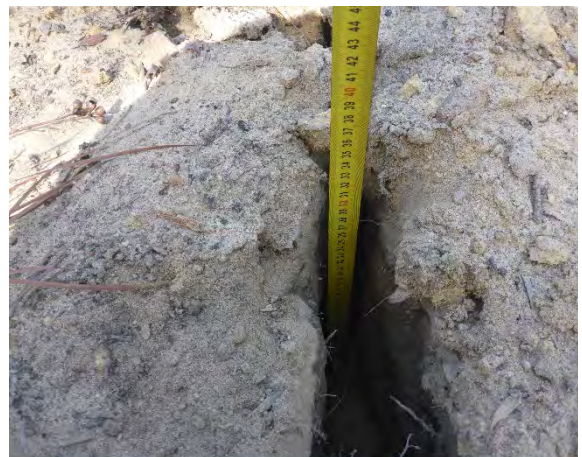
Photo 5: DA3B_LW16_004, looking at the depth of the soil cracking. Taken on 22/04/2020.
