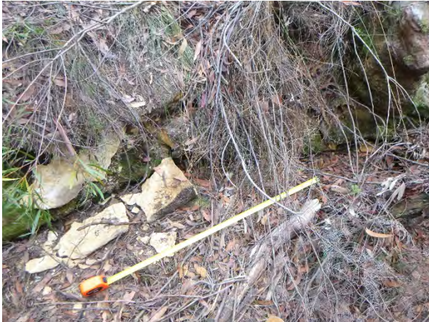
Photo 8: DA3B_LW16_011, overview of the rockfall. Taken on 27/04/2020.
