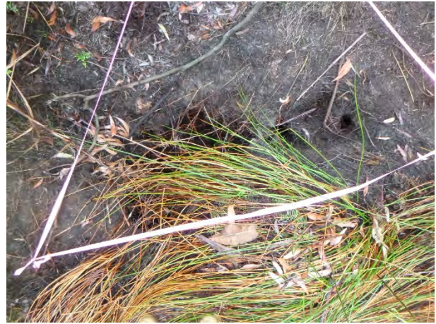
Photo 10: DA3B_LW16_030, localised erosion observed on tributary WC15. Taken on 09/09/2020.
