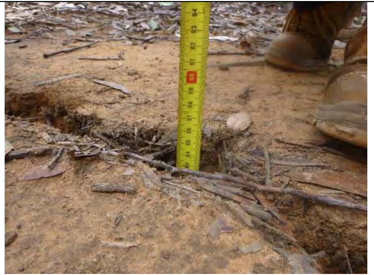
Photo 2: DA3B_LW16_027, showing depth of crack. Taken on 21/08/2020.
