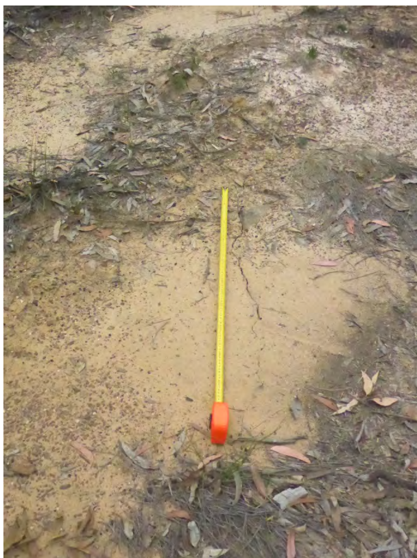
Photo 1: DA3B_LW16_039 soil cracking to access track. Taken on 7/10/2020.
