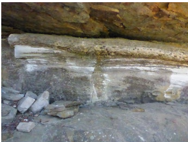
Photo 1: DA3B_LW16_031 , looking at the rock fracturing. Taken 28/09/2020.
