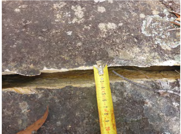
Photo 4: DA3B_LW16_048 , looking at the width of rock fracturing. Taken on 30/11/2020.
