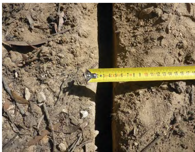
Photo 2: DA3B_LW16_003 , looking at the width of the rock fracturing. Taken on 22/04/2020.
