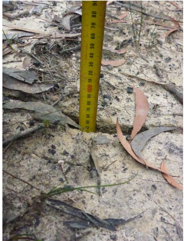
Photo 14: DA3B_LW16_043- depth measurement of soil cracking. Taken on 7/10/2020.
