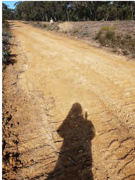
Photo 5: DA3B_LW16_019, looking at the remediated soil cracking. Taken on 29/06/2020.
