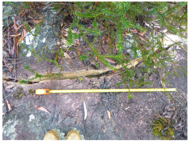
Photo 6: DA3B_LW14_019, looking at a section of rock fracturing. Taken on 9/09/2020.
