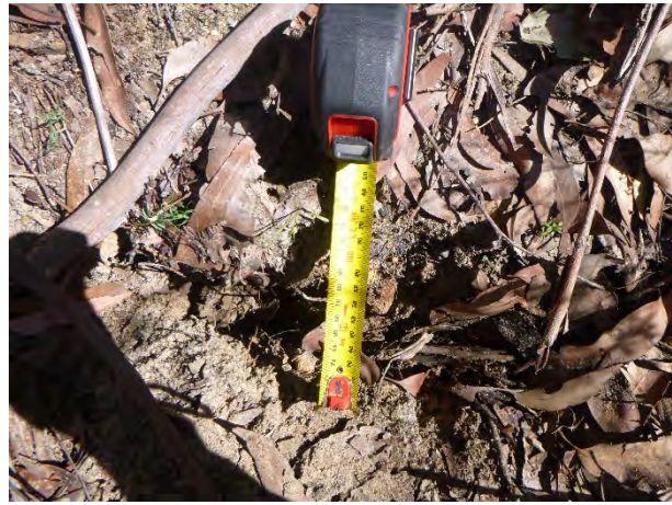
Photo 4: DA3B_LW16_032, looking at the width of soil cracking. Taken on 28/09/2020.
