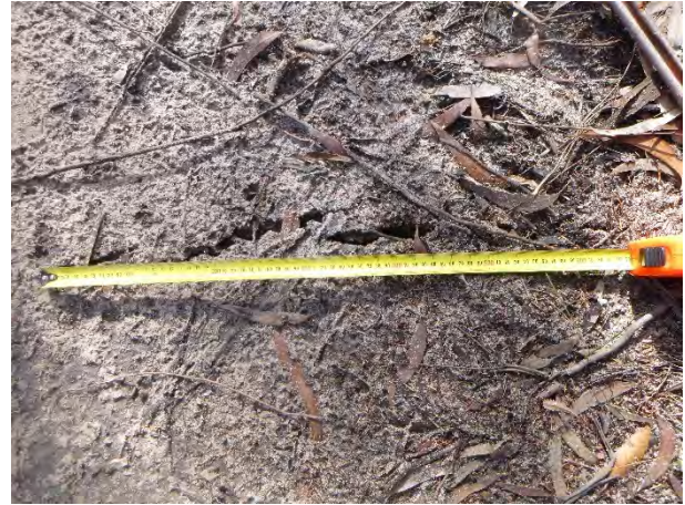
Photo 4: DA3B_LW16_013, looking at a section of soil cracking. Taken on 28/05/2020.
