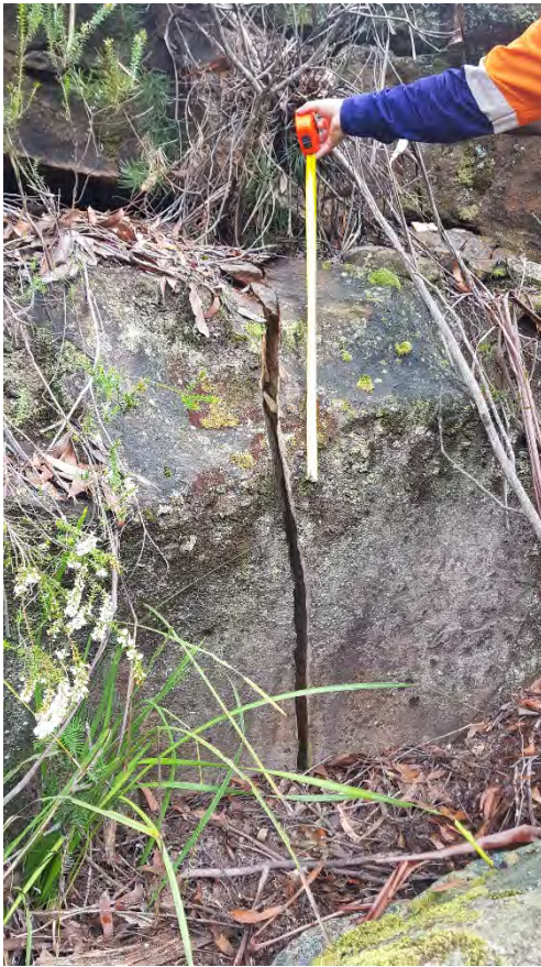
Photo 10: DA3B_LW16_012, looking at a section of rock fracturing. Taken on 28/04/2020.
