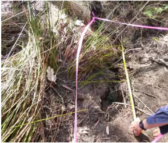
Photo 9: DA3B_LW16_030, localised erosion observed on tributary WC15. Taken on 31/08/2020.
