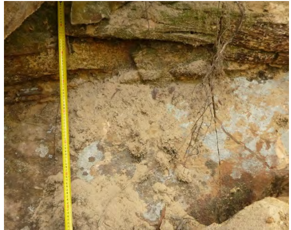
Photo 14: DA DA3B_LW16_016 looking at a section of rock fracturing. Taken on 15/05/2020.
