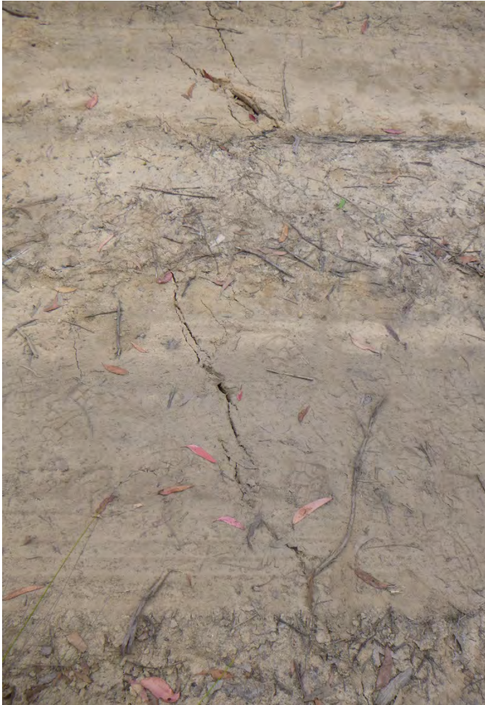
Photo 1: DA3B_LW16_008, an overview of the soil cracking. Taken on 27/04/2020.
