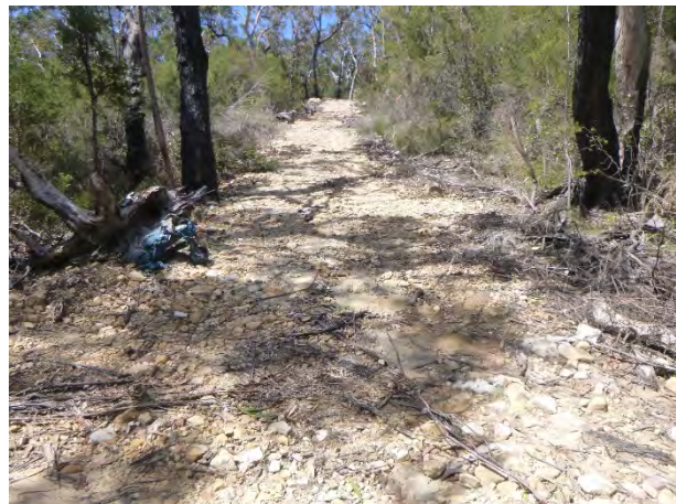
Photo 6: DA3B_LW16_033 looking at an overview of soil cracking. Taken on 28/09/2020.
