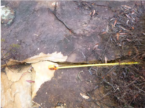
Photo 7: DA3B_LW14_019, looking at a section of rock fracturing and displacement. Taken on 9/09/2020.
