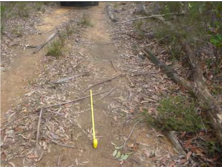
Photo 5: DA3B_LW16_027, looking along track, showing narrower section of cracking. Taken on 21/08/2020.
