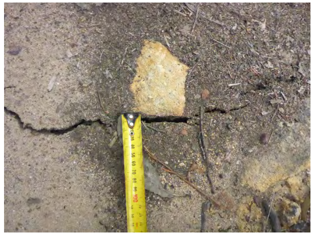
Photo 6: DA3B_LW16_041- soil cracking to access track. Taken on 7/10/2020.
