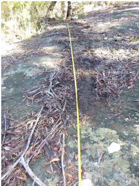
Photo 1: DA3B_LW16_017 , looking at the length of rock fracturing. Taken on 16/06/2020.
