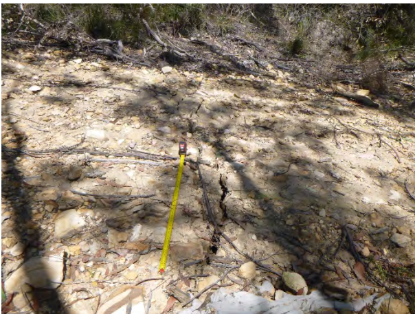
Photo 5: DA3B_LW16_033, looking at a length of soil cracking. Taken 28/09/2020.
