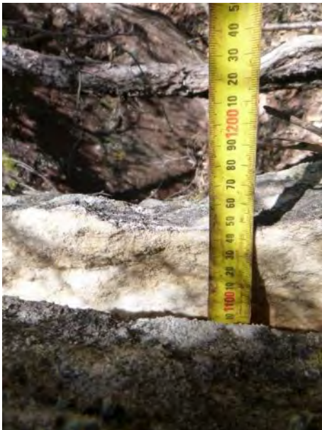
Photo 5: DA3B_LW16_045 , looking at depth of rock fracturing. Taken on 10/11/2020.
