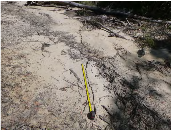
Photo 7: DA3B_LW16_034, looking at the length of soil cracking. Taken 28/09/2020.
