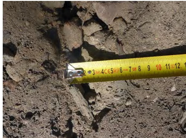
Photo 9: DA3B_LW16_007, looking at the width of the soil cracking. Taken on 22/04/2020.
