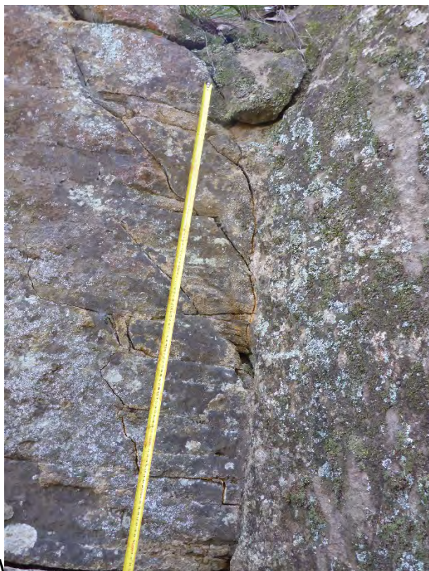
Photo 15: DA3B_LW16_026 , looking at a section of rock fracturing. Taken on 6/08/2020.
