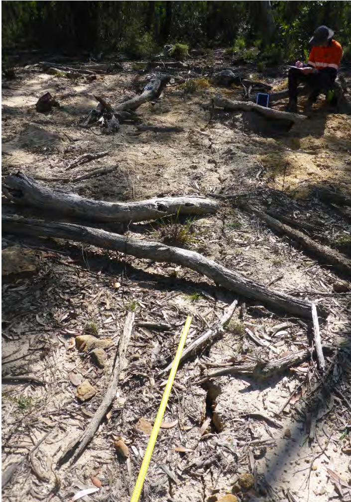
Photo 3: DA3B_LW16_005, an overview of the soil cracking. Taken on 22/04/2020.
