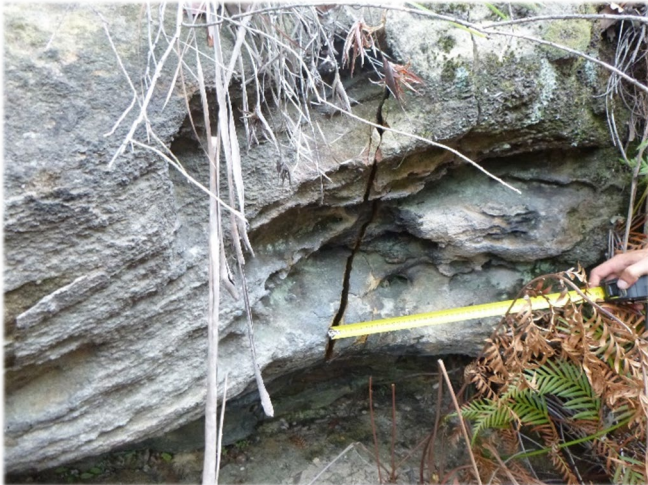
Photo 18: DA3B_LW15_019, looking at width of rock fracture. Taken on 27/02/2020.
