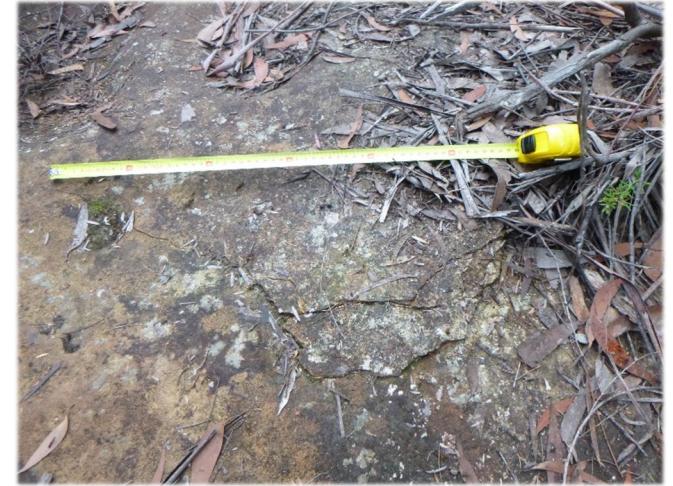
Photo 3: DA3B_LW15_015, looking at a section of rock fracturing. Taken on 11/10/2019.
