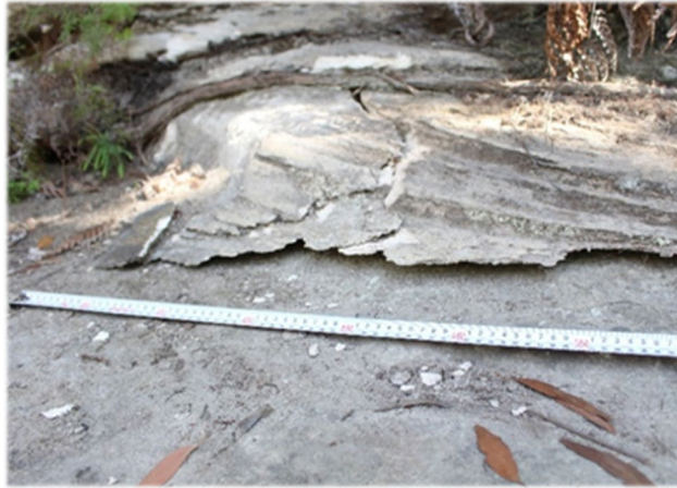
Photo 29: Browns Road Site 11, subsidence related fracturing and exfoliation. Taken: 15th March 2020.
