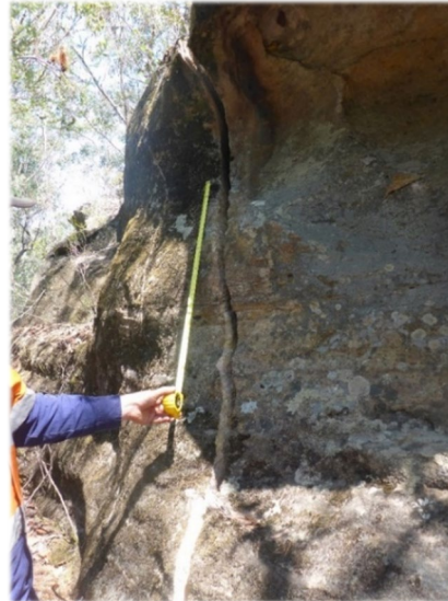
Photo 22: DA3B_LW15_023, looking at a section of rock fracturing. Taken on 25/10/2019.
