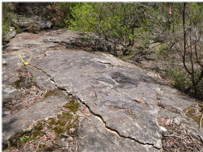
Photo 4: DA3B_LW15_027, looking at the rock fracture. Taken on 21/01/2020.
