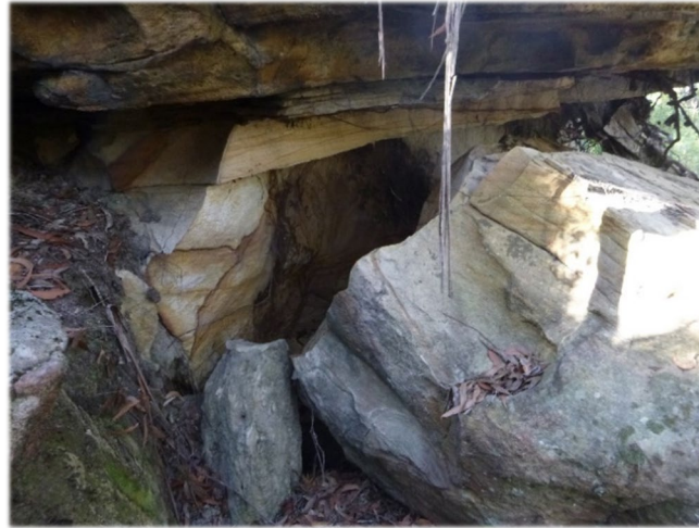
Photo 10: DA3B_LW15_002 , looking at the rockfall. Taken on 29/05/2019.
