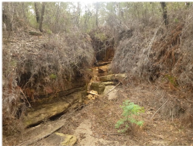
Photo 5: DA3B_LW13_010, rockfall at the inflow step to WC21_Pool 53. Taken on 26/02/2020.
