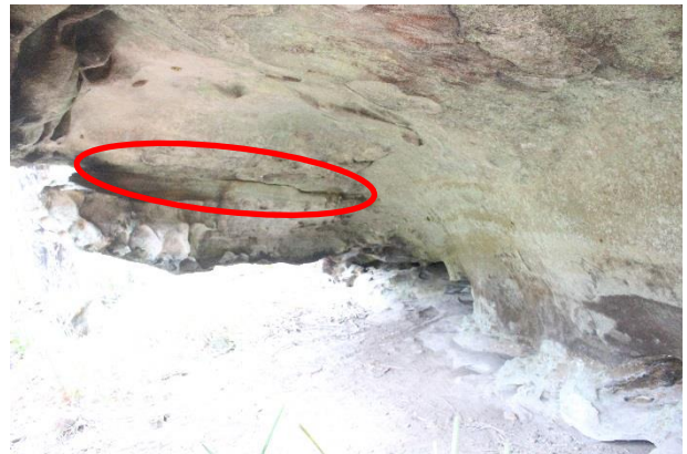
Plate 34: Comparison image of interior of the shelter taken during Biosis (2012) Longwall 9 -18 baseline recording. Location of natural fissuring circled in red (source: Biosis 2012).
