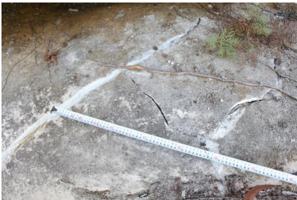
Plate 6: Location of cracks 3 and 4 from an aerial aspect.
