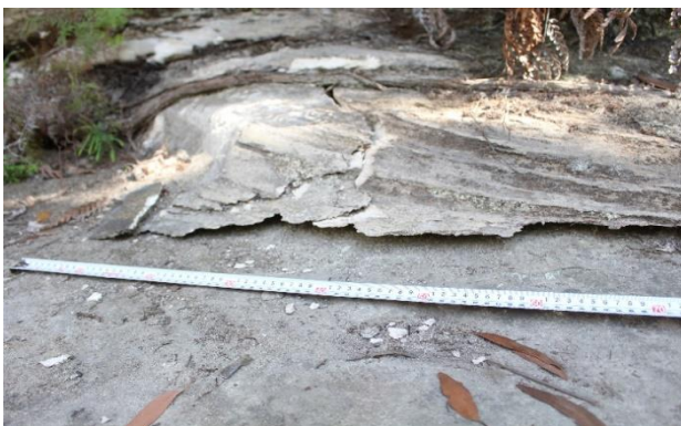
Plate 10: Sandstone exfoliation platform at crack 6.
