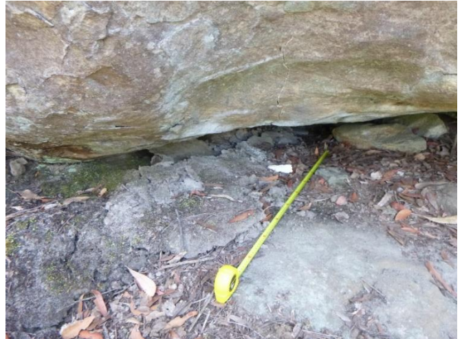
Photo 83: DA3B_LW15_024, looking at area of soil uplift. Taken on 21/01/2020.
