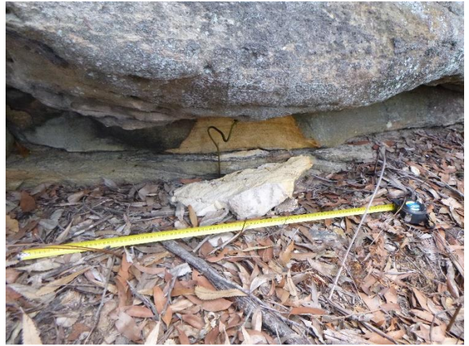
Photo 67: DA3B_LW15_017, looking at the area of rockfall. Taken on 27/02/2020.
