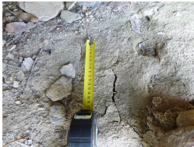
Photo 92: DA3B_LW15_026, looking at soil cracking. Taken on 27/02/2020.
