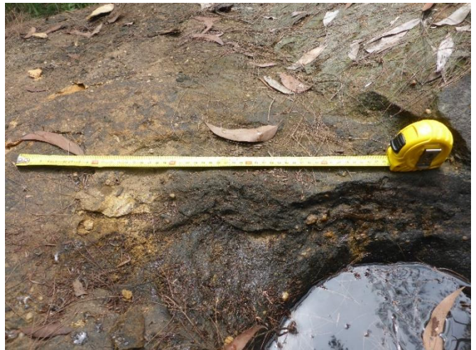
Photo 41: DA3A_LW8_003, looking at the rock fracturing and uplift. Taken on 28/01/2020.
