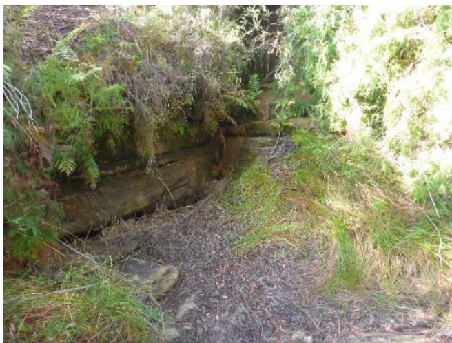
Photo 15: DA3B_LW13_010, step at WC21_Pool 53. Taken on 27/10/2017.
