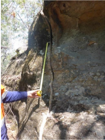
Photo 80: DA3B_LW15_023, looking at section of rock fracture. Taken on 25/10/2019.
