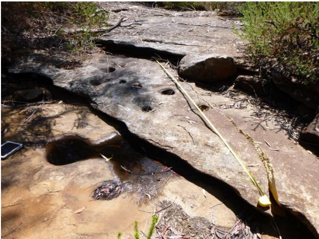
Photo 31: DA3B_LW14_016, looking at the rock fracture and displacement. Taken on 21/01/2020.
