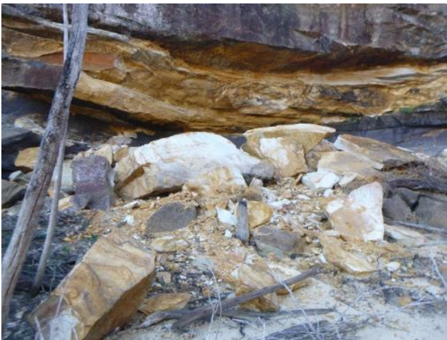
Photo 98: DA3B_LW14_015, looking at the rockfall and associated debris. Taken on 11/6/2019.
