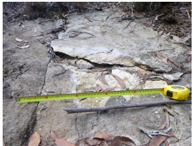
Photo 44: DA3A_LW8_004, looking at the rock fracturing and uplift. Taken on 28/01/2020.
