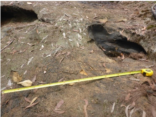
Photo 40: DA3A_LW8_003, looking at the rock fracturing and uplift. Taken on 28/01/2020.
