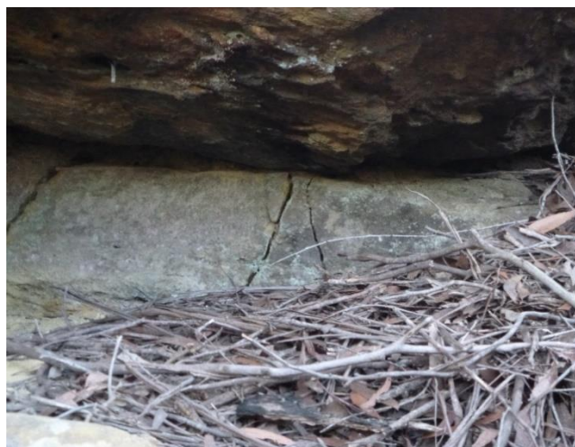
Photo 46: DA3B_LW15_001, looking at a section of rock fracturing. Taken on 29/05/2019.
