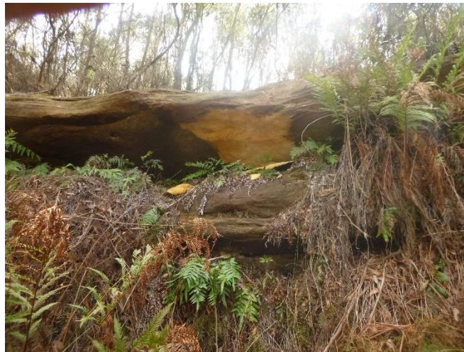
Photo 59: DA3B_LW15_009, looking at a section of rockfall. Taken on 26/02/2020.
