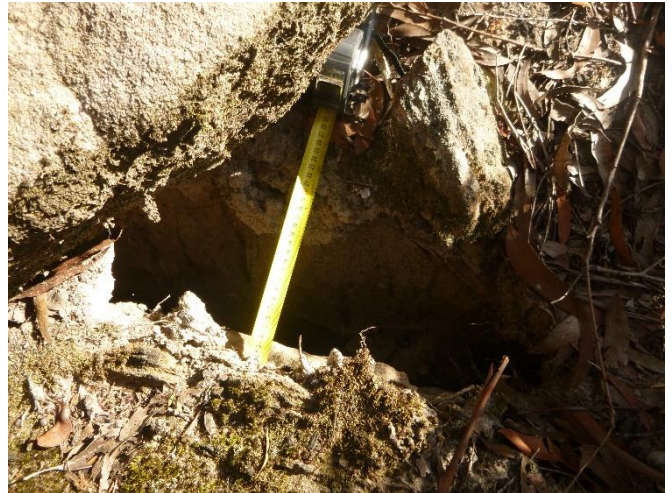
Photo 85: DA3B_LW15_024, looking at rock uplift. Taken on 28/02/2020.
