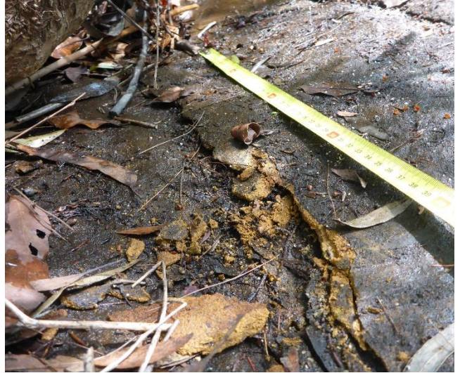
Photo 39: DA3A_LW8_002, looking at the rock fracturing and uplift. Taken on 28/01/2020.
