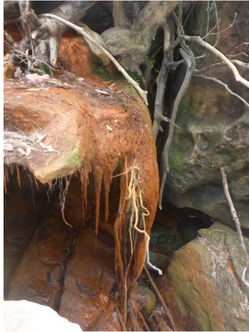
Photo 42: DA3A_LW8_003, looking at iron staining on step. Taken on 28/01/2020.
