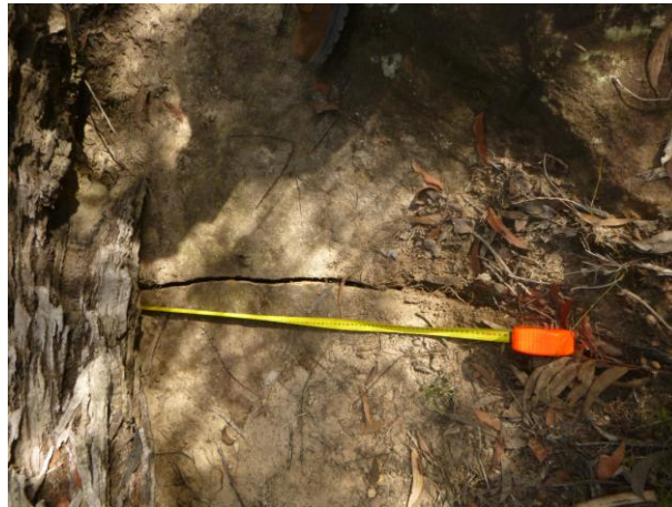
Photo 53: DA3B_LW15_006, looking at soil cracking. Taken on 09/07/2019.
