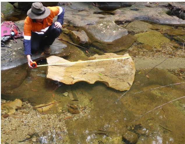
Photo 29: DA3B_LW13_046, looking at the section of rock displaced. Taken on 10/03/2020.
