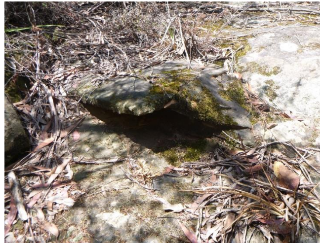
Photo 20: DA3B_LW15_027, looking at an area of uplift. Taken on 21/01/2020.
