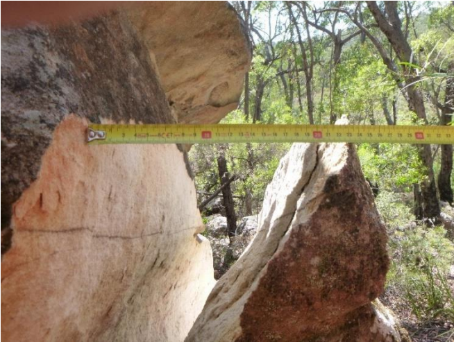
Photo 86: DA3B_LW15_025, looking at the rockfall. Taken on 21/01/2020.
