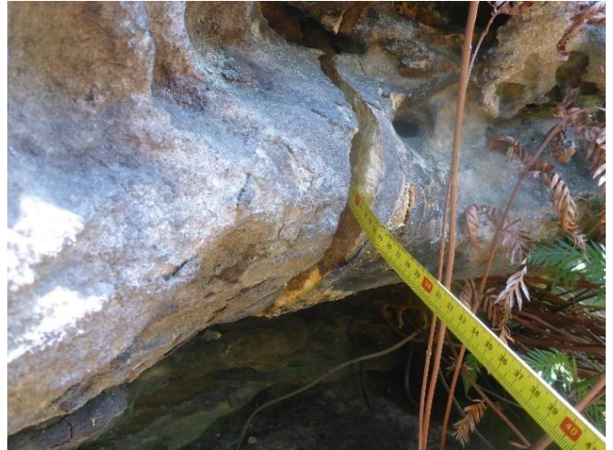
Photo 71: DA3B_LW15_019, looking at horizontal depth of rock fracture. Taken on 25/10/2019.
