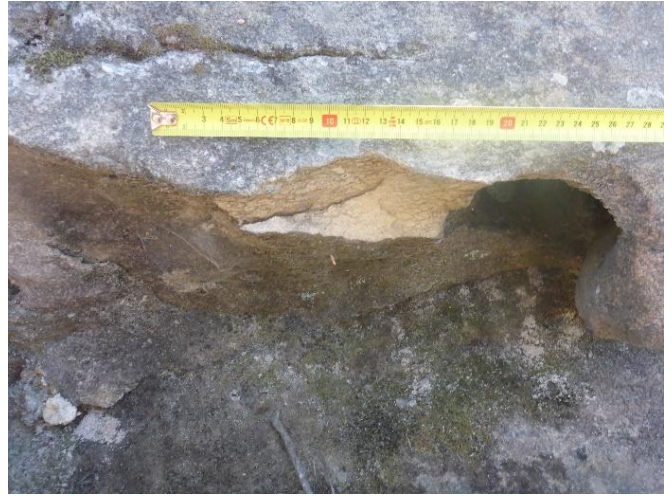
Photo 78: DA3B_LW15_022, looking at area of rock displacement. Taken on 25/10/2019.
