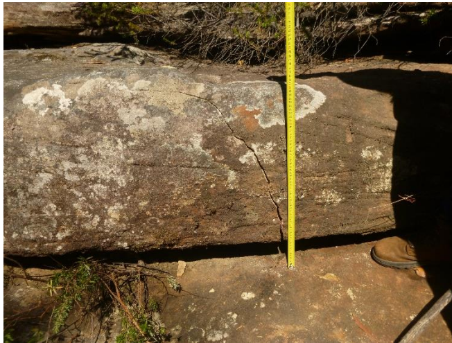
Photo 35: DA3B_LW14_016, looking at the rock fracture. Taken on 28/02/2020.
