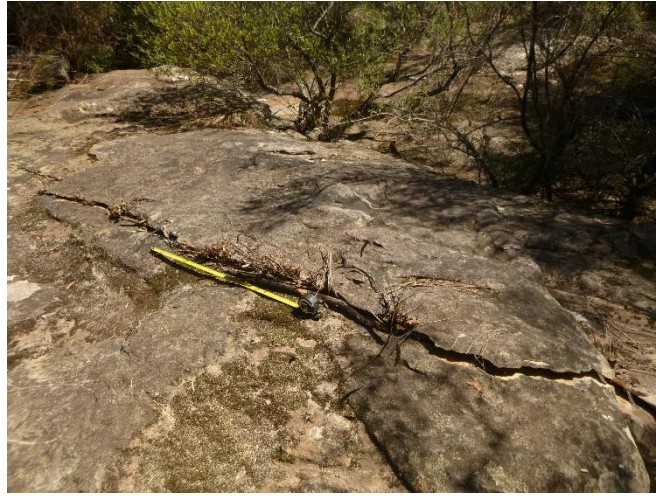
Photo 21: DA3B_LW15_027, looking at the rock fracture. Taken on 28/02/2020.
