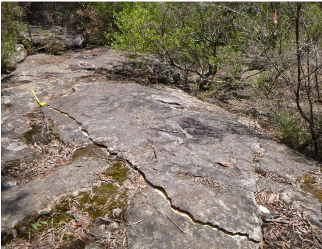
Photo 19: DA3B_LW15_027, looking at rock fracture. Taken on 21/01/2020.
