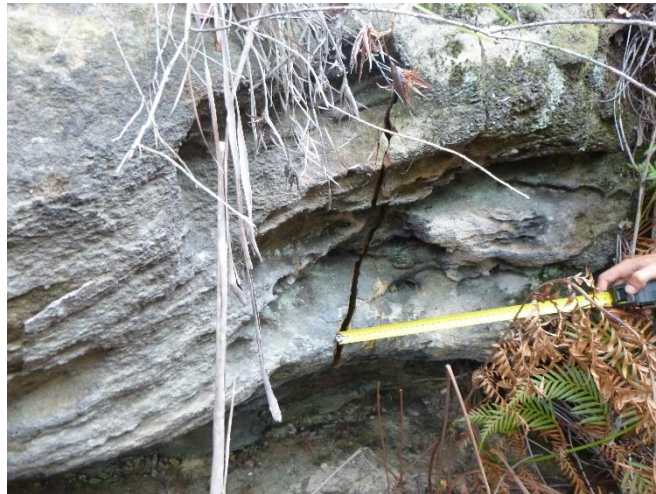
Photo 72: DA3B_LW15_019, looking at width of rock fracture. Taken on 27/02/2020.
