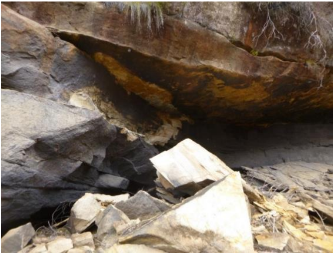
Photo 96: DA3B_LW14_015, looking at the original rockfall. Taken on 5/12/2018.
