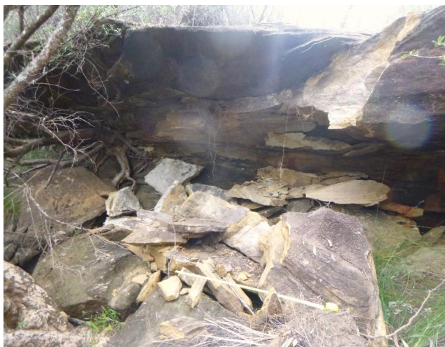
Photo 9: DA3B_LW15_014 , an overview of the rockfall. Taken on 11/10/2019.
