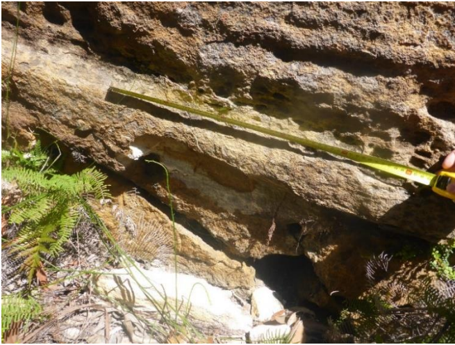
Photo 73: DA3B_LW15_020, looking at area of rockfall. Taken on 25/10/2019.
