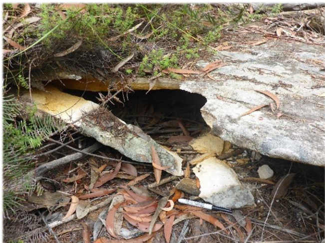
Photo 1: DA3B_LW14_016, looking at fracturing and dislodged rock segments. Taken on 21/01/2019.
