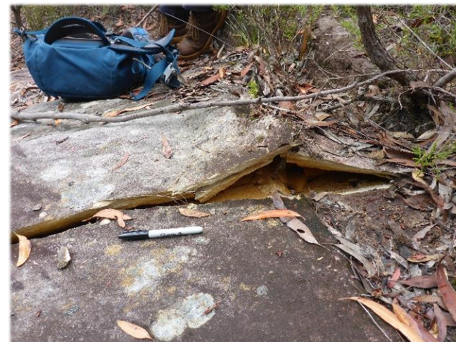
Photo 9: DA3B_LW13_035, fracturing and uplift on rockbar. Taken on 21/01/2019.
