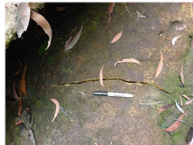
Photo 6: DA3B_LW14_021, looking at the section of rock fracturing. Taken 20/02/2019.
