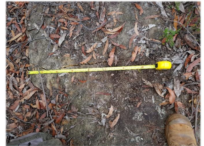
Photo 20: DA3B_LW14_028, looking at a section of rock fracturing. Taken 10/05/2019.
