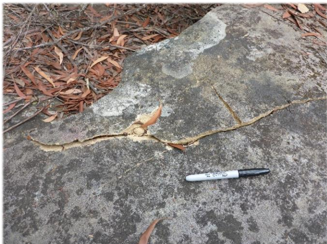
Photo 7: DA3B_LW14_022, looking at the section of rock fracturing. Taken 20/02/2019.
