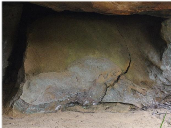
Photo 25: Subsidence related cracking in the north side of the Site 1-DB1 shelter. Taken: 10 th May 2019.
