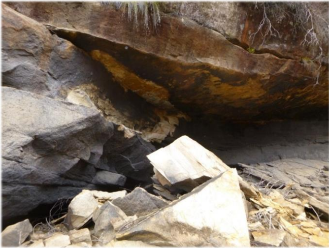
Photo 15: DA3B_LW14_015, looking at the rockfall. Taken 5/12/2018.
