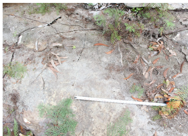
Plate 4: Subsidence cracking north of the shelter.
